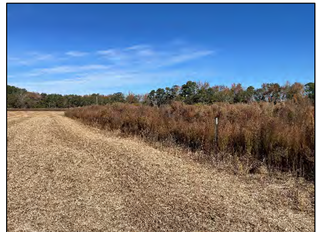
Former encroachment area showing extra posts and grown-up vegetation (11/20/2023)
