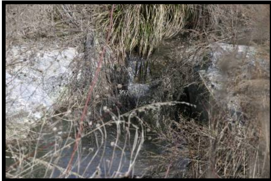
Station 08+20 Big Drop
