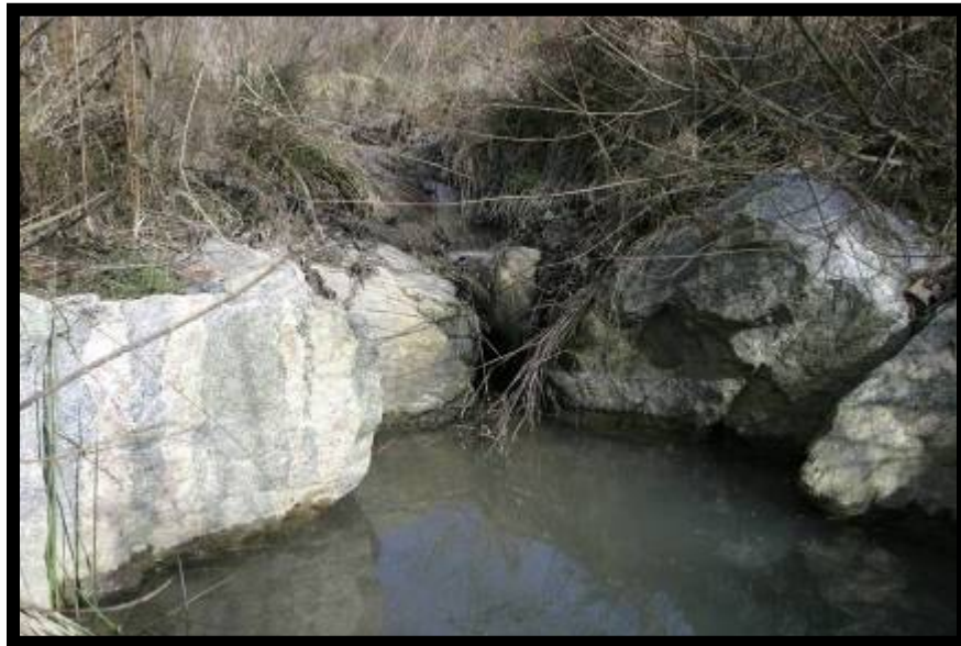
Station 03+40 Piping Vane Upstream
