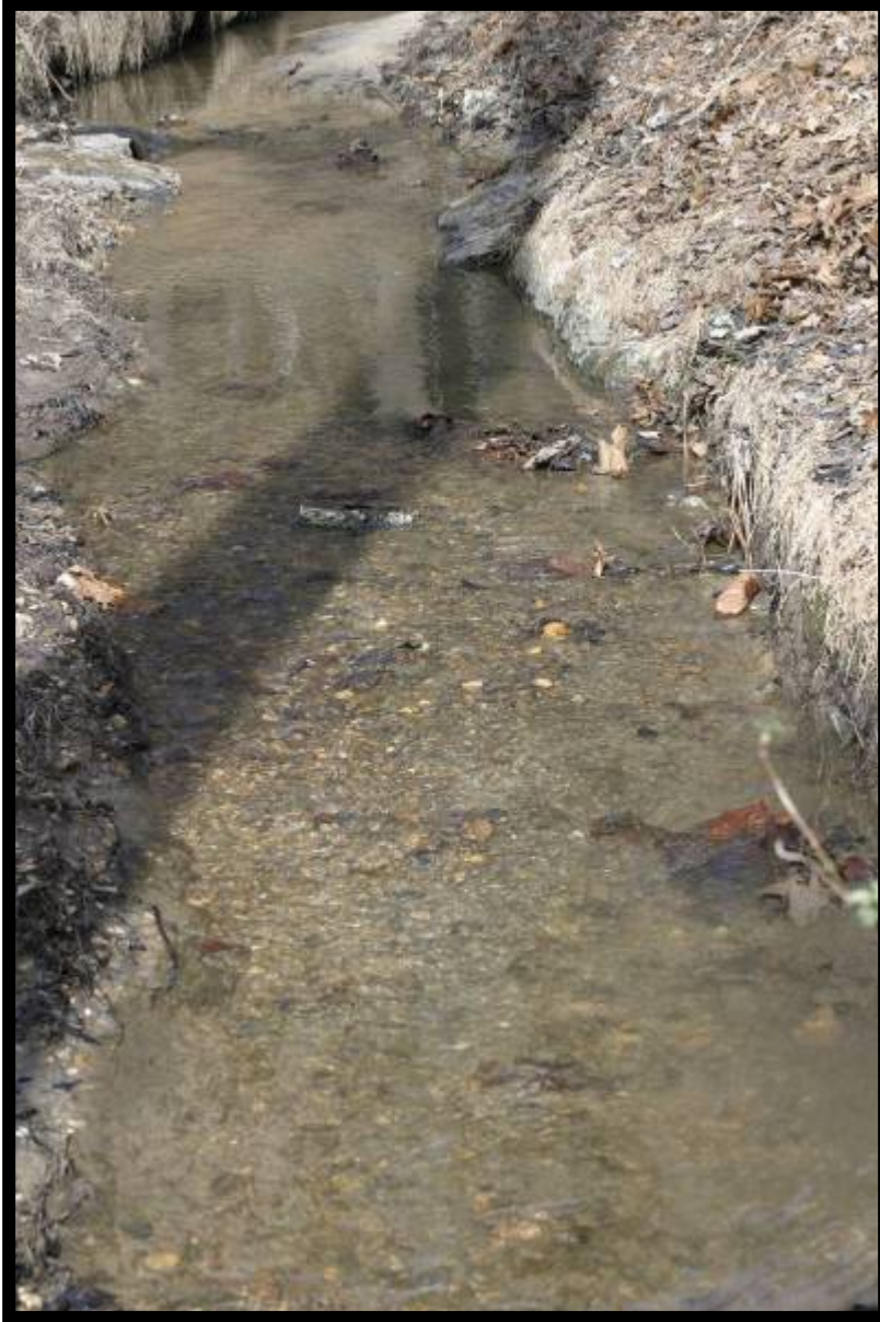
Station 13+50 Unnecessary Vane
