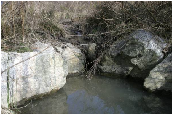
Issue Photo 1. Piping under Structure STA: 3+25
