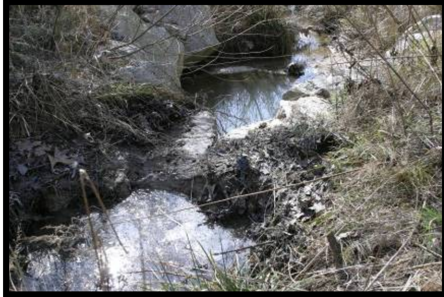
Station 03+40 Piping Vane Downstream
