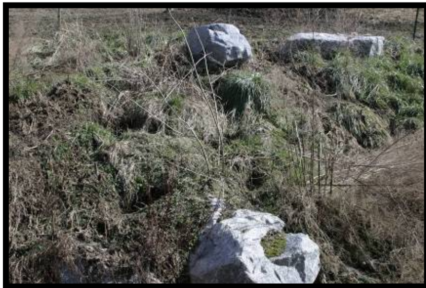
Station 07+70 Runoff Gulley
