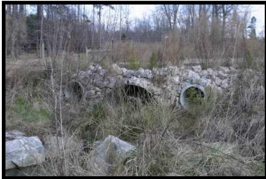
Station 05+60 Floodplain Culvert Outlet
