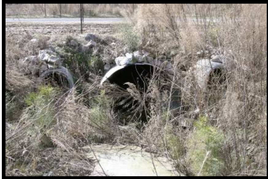
Station 04+30 Floodplain Culvert Inlet
