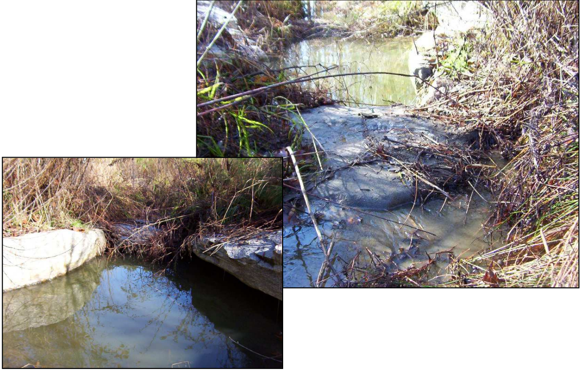
Photo 9. Piping of flow behind Rock Vane 11.
