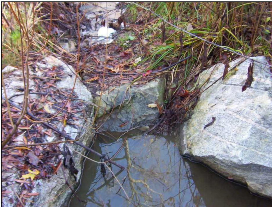
Photo 2. Piping of flow behind Rock Vane 3.
