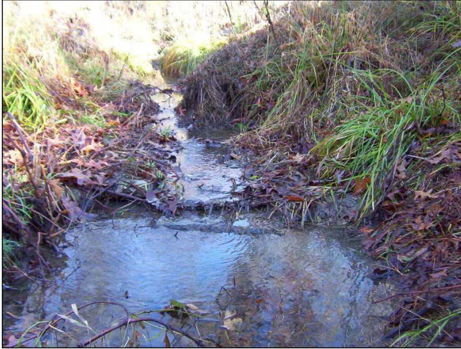
Photo 1. Rock Vane 2 has filled in with sediment but stream remains stable.
