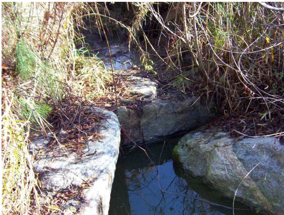
Photo 6. Piping of flow behind Rock Vane 11.
