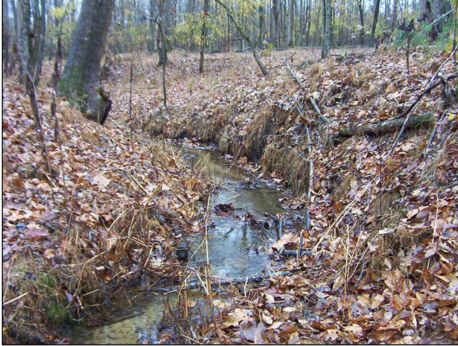
Photo 11. Minor erosion along outside bend where channel is pinched.
