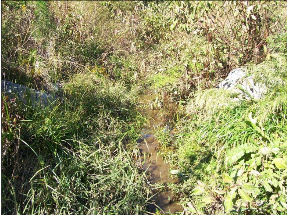
Photo 8. Rock Vane 14 has filled in with sediment but stream remains stable.
