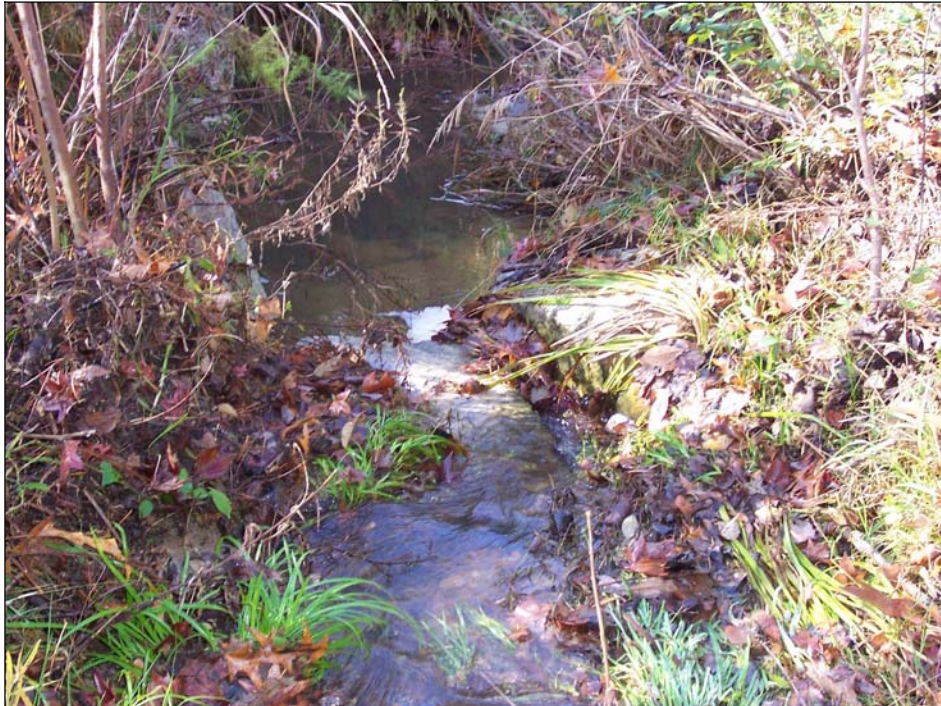
Photo 2. Piping of flow behind Rock Vane 3.
