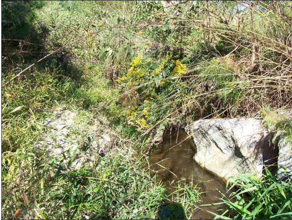
Photo 9. Rock Vane 16 has accrued sediment but stream remains stable.
