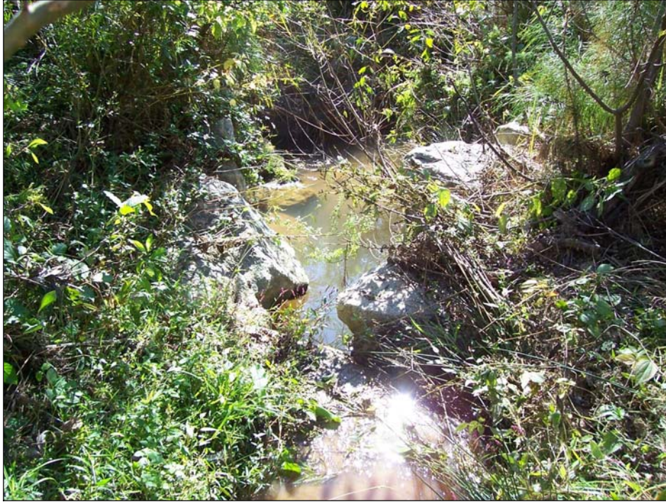
Photo 5. Piping of flow behind Rock Vane 8.
