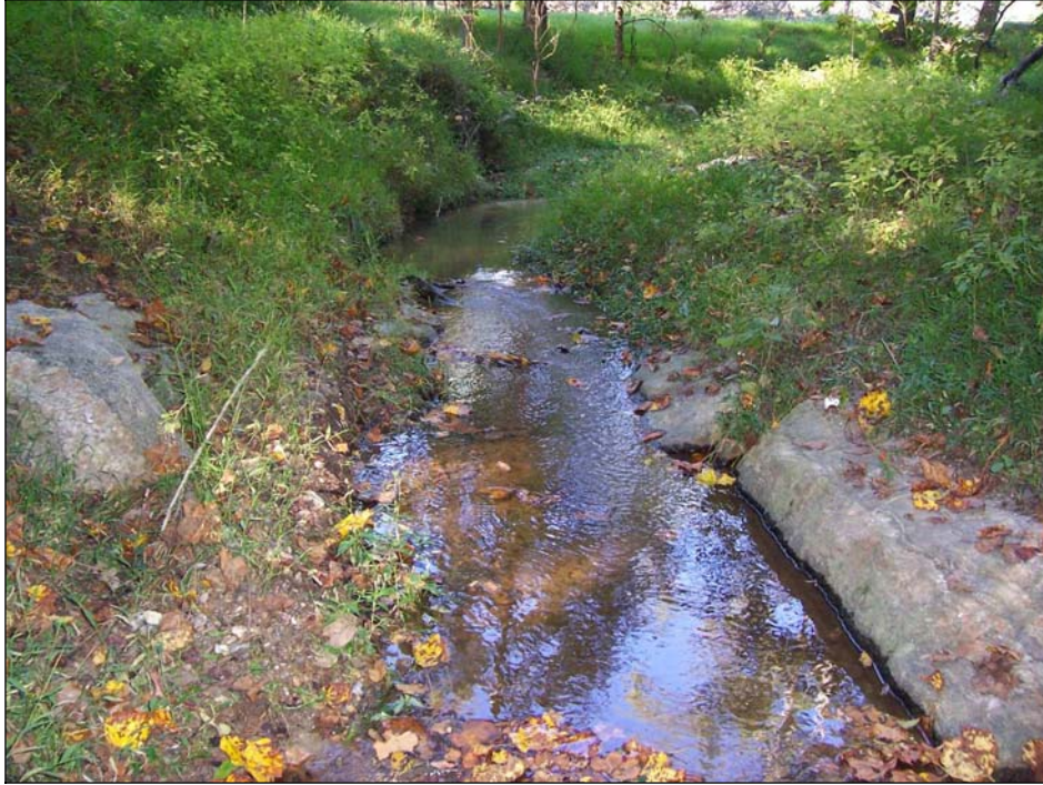
Photo 13. Rock Vane 24 has filled accrued sediment but stream remains stable.
