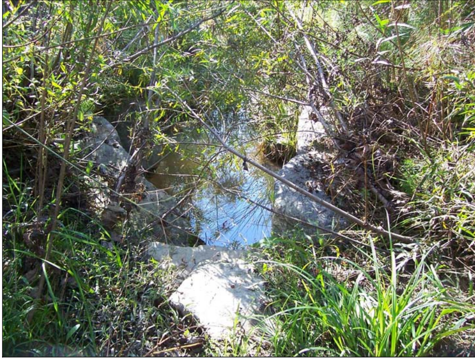
Photo 7. Piping of flow behind Rock Vane 11.
