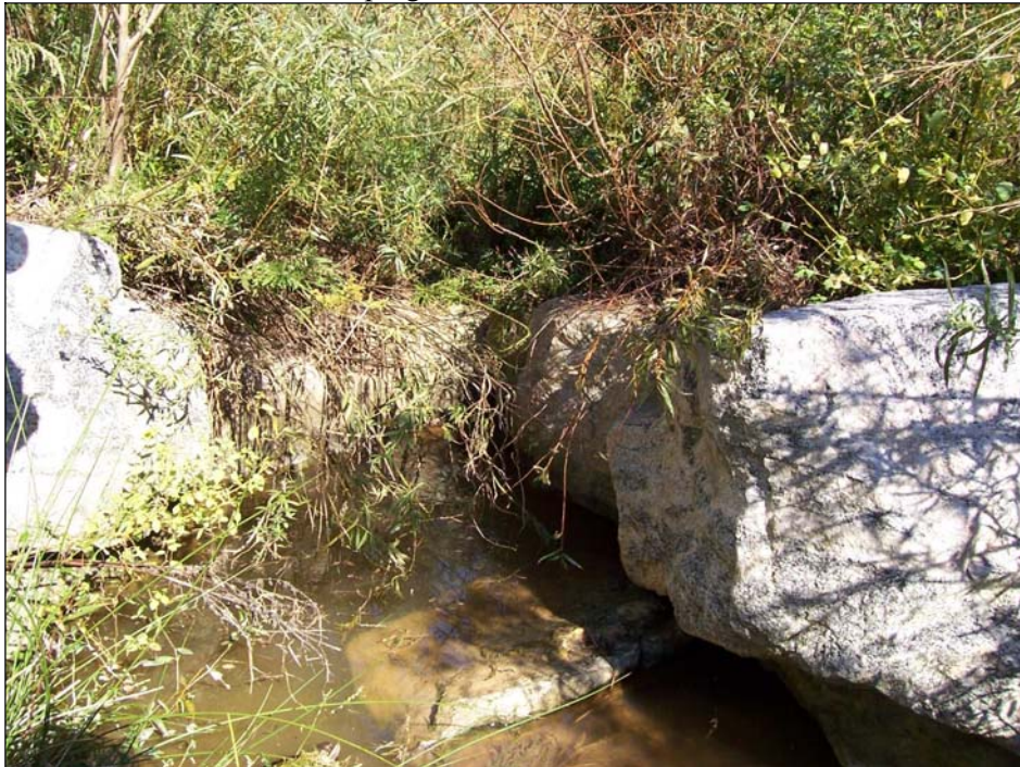
Photo 6. Piping of flow behind Rock Vane 10.
