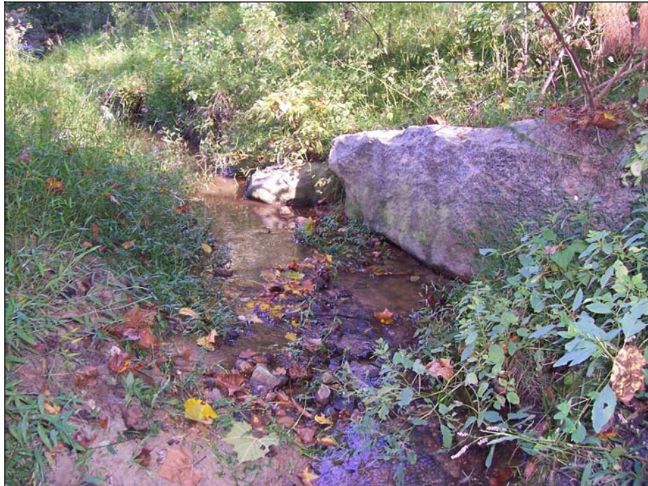
Photo 12. Rock Vane 22 has accrued sediment but stream remains stable.
