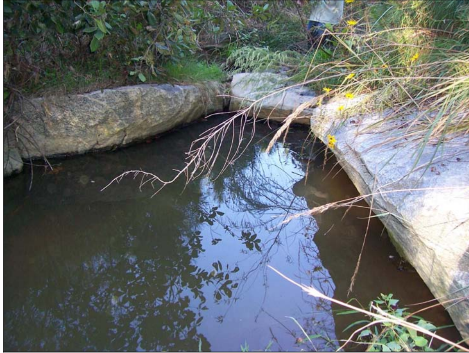
Photo 11. Piping of flow behind Rock Vane 19.
