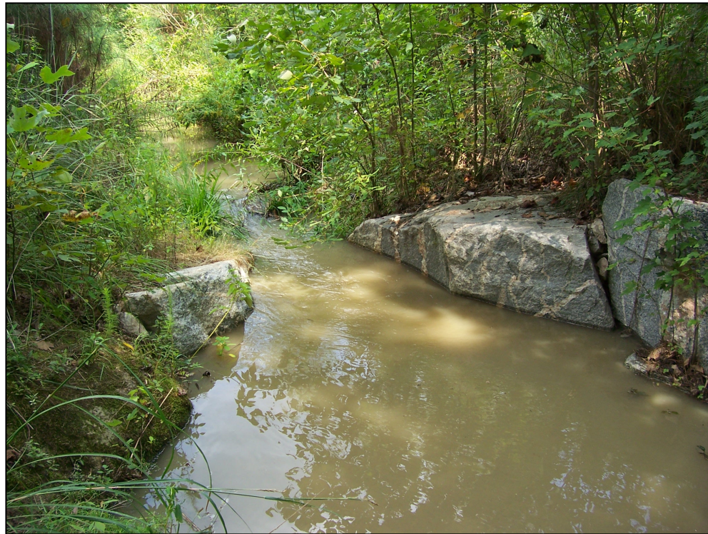
Photo 9. Rock vane 20 flooded from downstream beaver dams.
