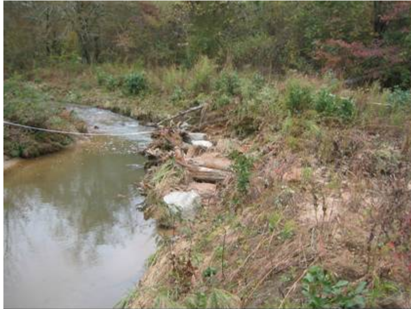
SP1. Station 3+60 to 4+20 Erosion and scour around root wads
