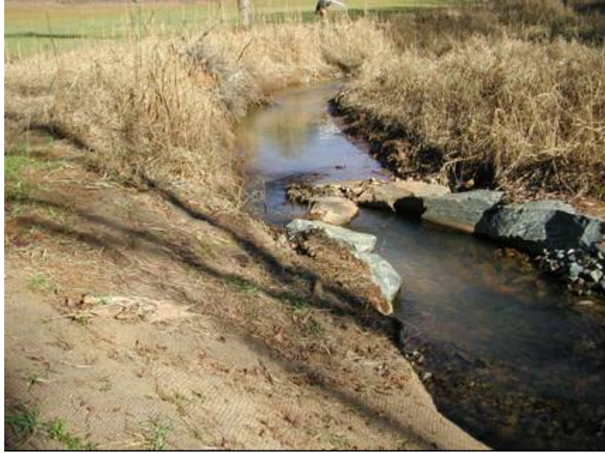
SP13. 2002 Station 13+50 to 13+80 Cutting around cross vane
