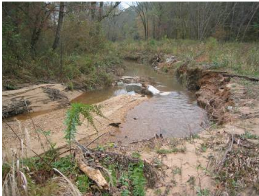
SP18. Station 22+20 to 22+80 Blowout around vane
