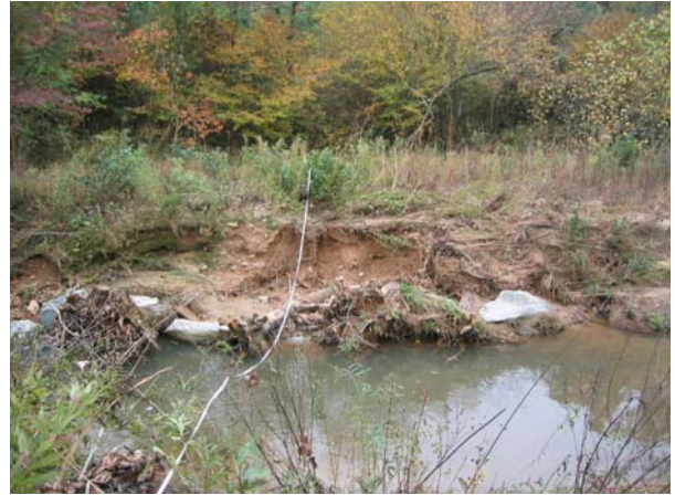
Photo 9. Station 3+80 Cross section 2. Left Bank
