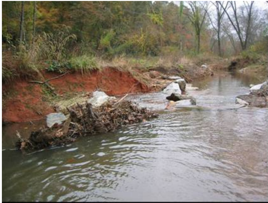
SP10. Station 12+00 to 12+60 Blowout around root wad and cross vane
