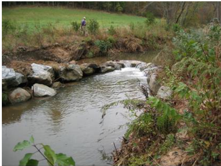
SP6. Station 10+60 Piping through cross vane
