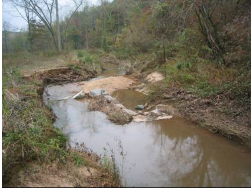
SP19. Station 22+20 to 22+80 Blowout around vane
