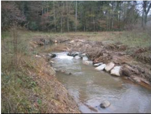
SP27. Station 40+30 to 40+50 Piping around vane
