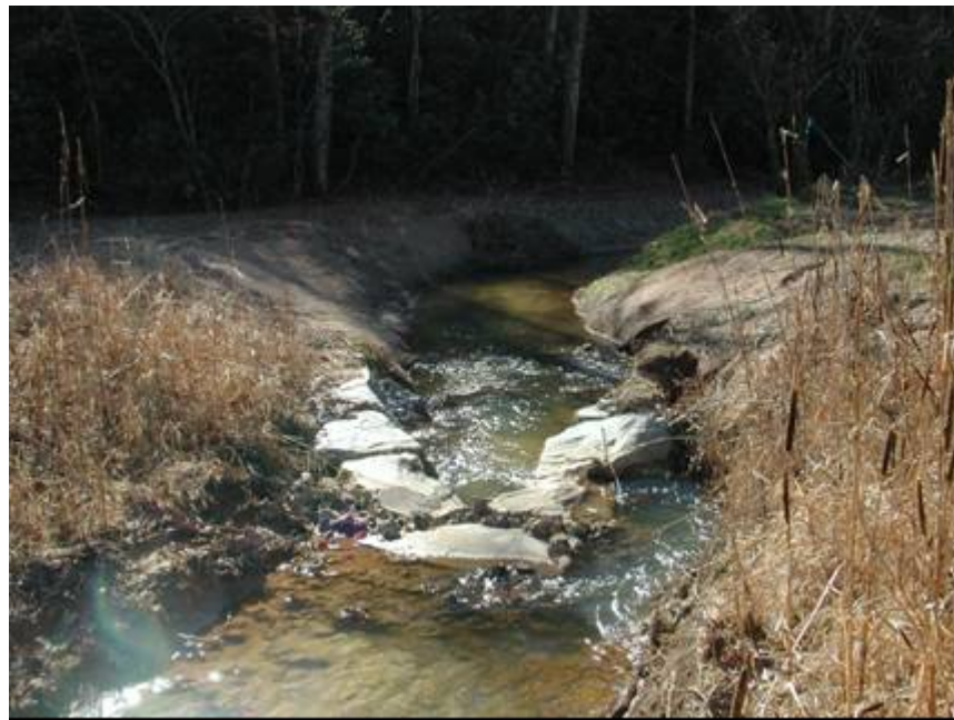
SP12. 2002 Photo Station 13+50 to 13+80 Cutting around cross vane
