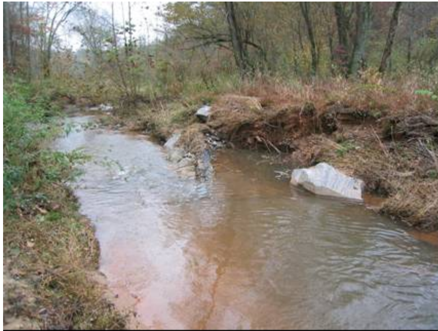
SP16. Station 17+00 to 17+20 Cutting around log cross vane
