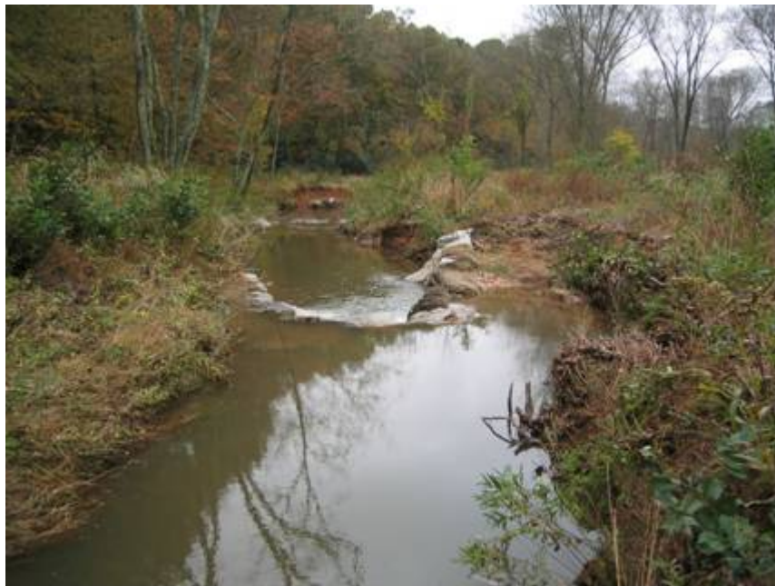
SP8. Station 11+10 to 11+30 Scour downstream of cross vane
