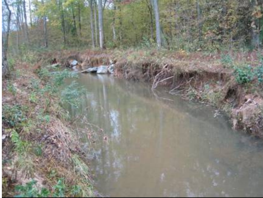
SP5. Station 8+80 to 9+20 Erosion and scour around root wads
