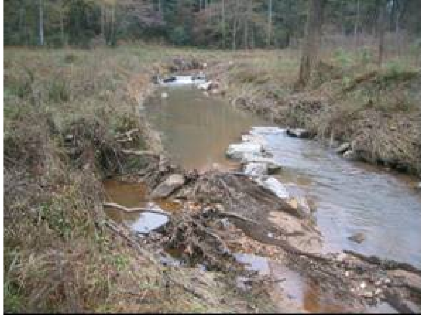
SP29. Station 40+90 to 41+10 Cutting around vane
