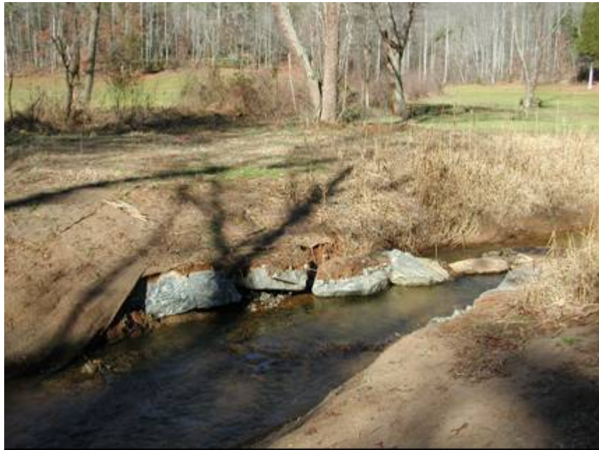
SP14. 2002 Station 13+50 to 13+80 Cutting around cross vane
