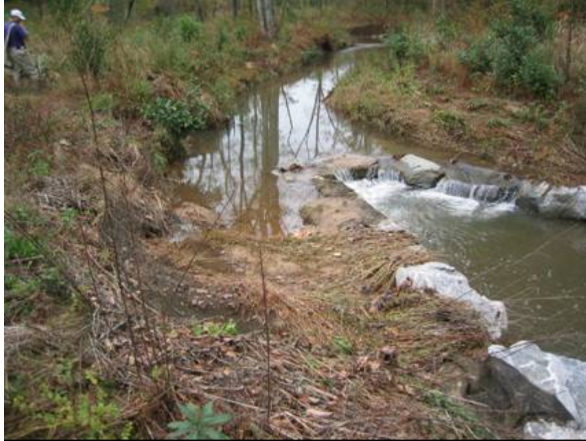
SP7. Station 11+10 to 11+30 Scour downstream of cross vane
