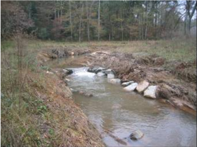
Photo 32. End of the project looking upstream
