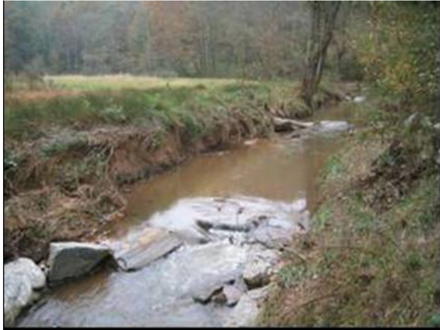
SP26. Station 39+20 to 39+40 Bare lower bank
