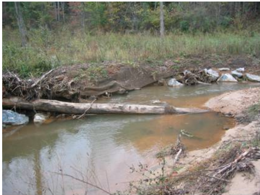
SP20. Station 24+80 to 25+10 Log vane moved
