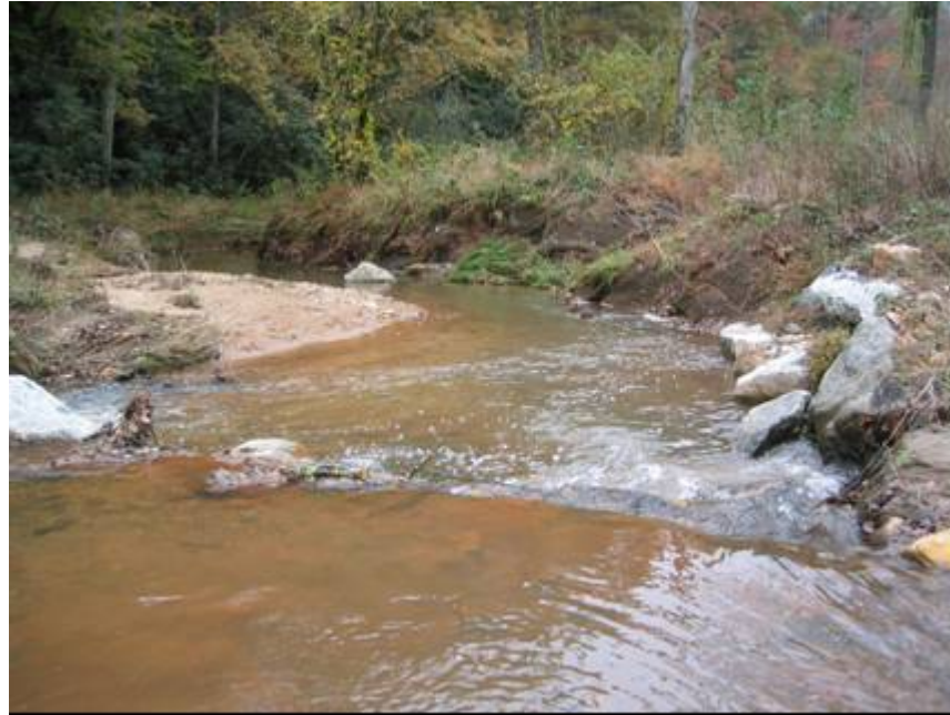
SP11. Station 13+50 to 13+80 Cutting around cross vane
