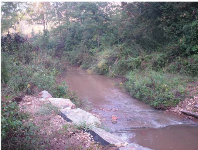
P41 facing downstream
