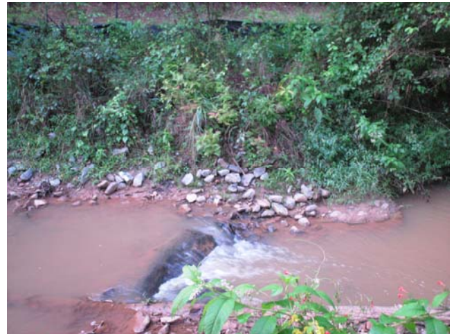
P34 facing left bank
