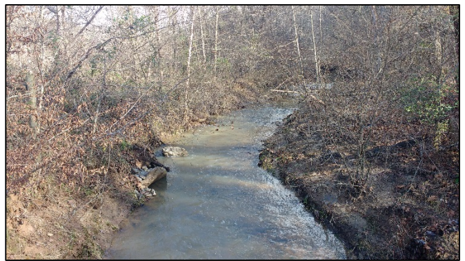
P42 facing upstream
