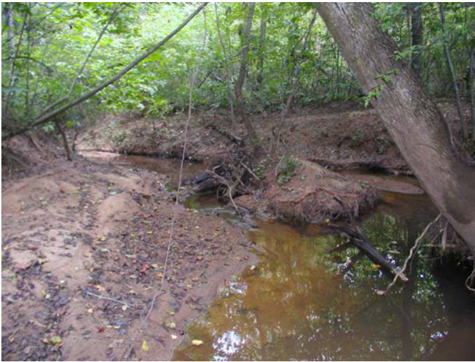
Photo 2 UT1 Channel Widening
