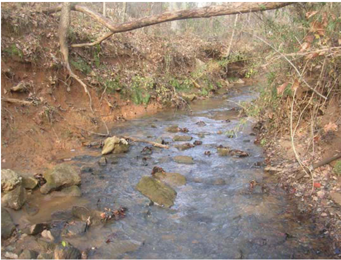
Photo 1 UT1 Bank Erosion at Riffle
