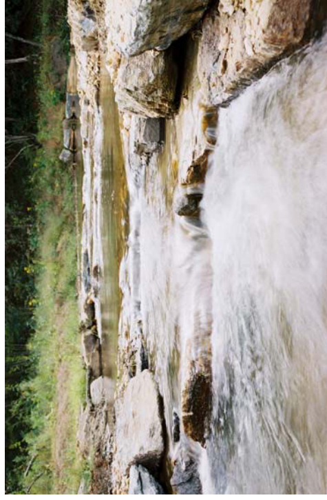
Double Drop Rock Cross Vane
