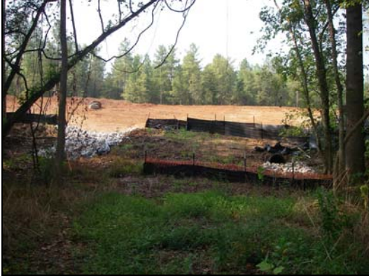
Detention Pond – Adjacent to UT2 at STA 20+00
