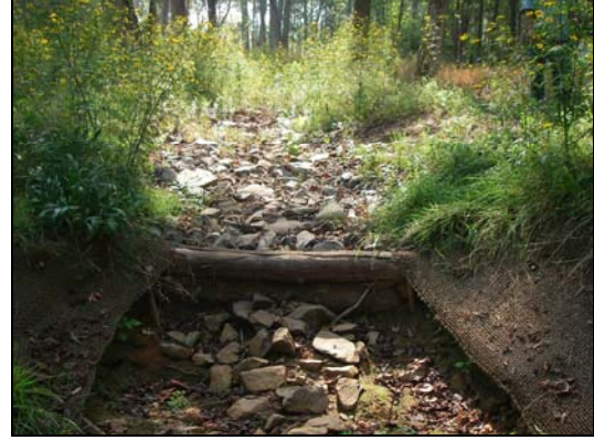
Beginning headcut below riffle at STA 20+00 on UT2
