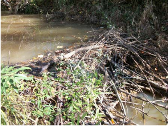
UT1 – Beaver dam at Station 10+20
