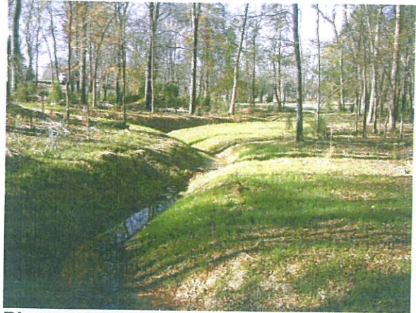
Photograph 2 Fixed Station 2. Overview of UT1, looking upstream near station 19+00.
