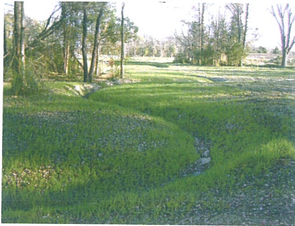
Photograph 5 Fixed Station 5. Overview of UT1, looking downstream from upstream project limits.
