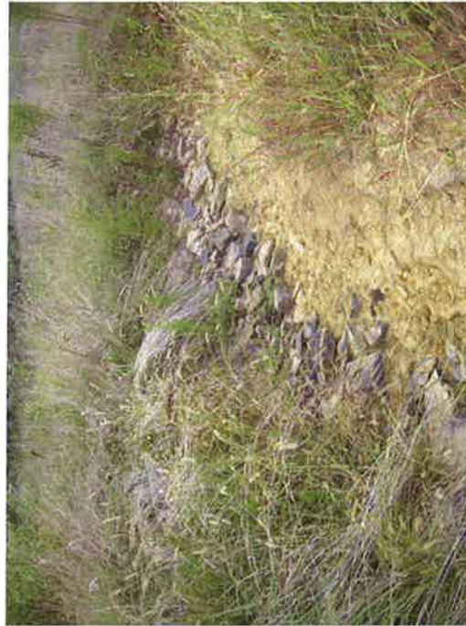
Cross-section photo – looking upstream
