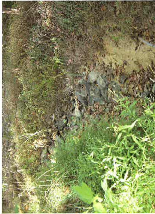
Cross-section photo – looking upstream
