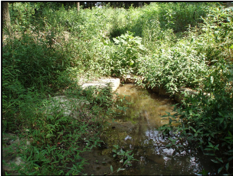
SPA 4. UT2 Sta. 211+70 Header rocks set to high at rock A-vane.
