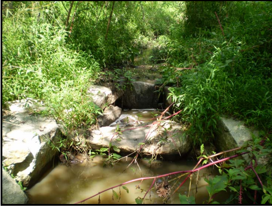
SPA5 – Piping around header rock on rock A-vane @ station 211+30 (UT2)
