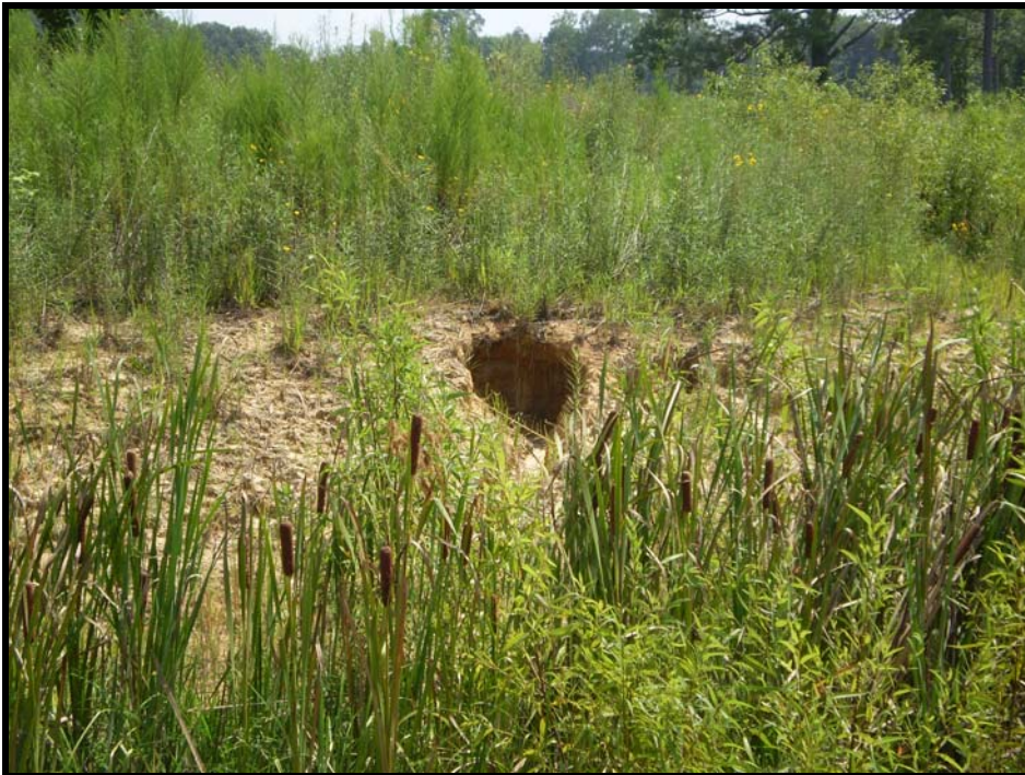
SPA6 – Erosion on left bank @ station 329+50 (UT3)
