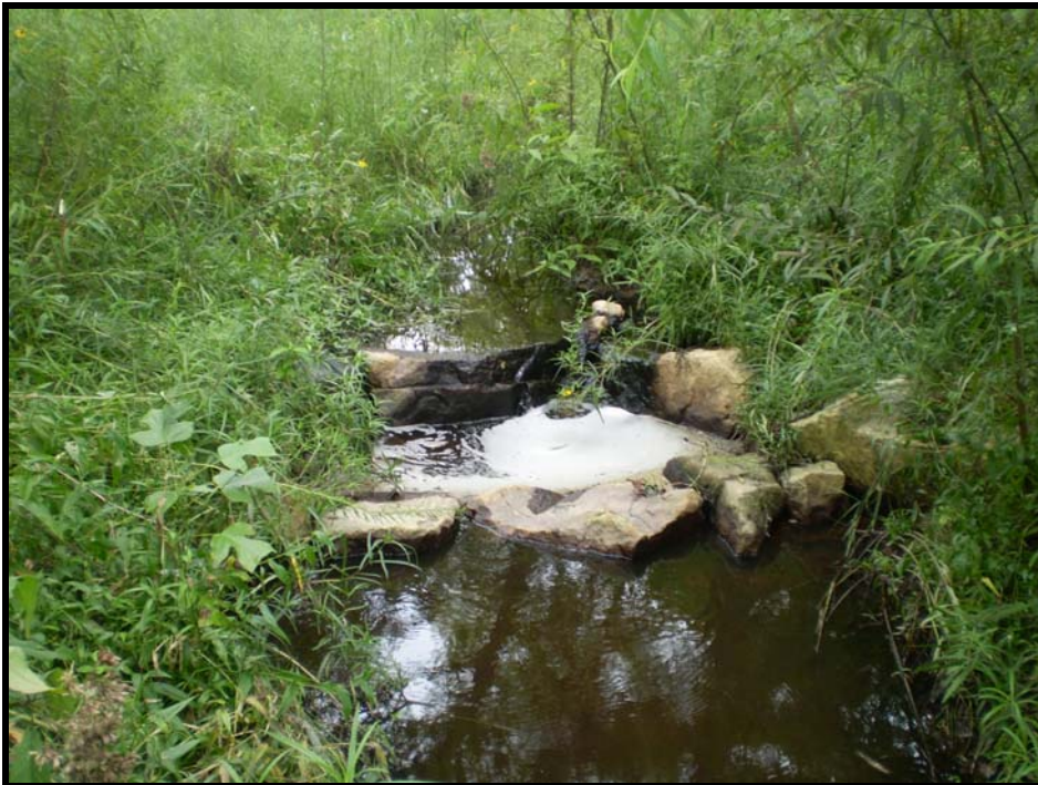
SPA2 – Piping around header rock on rock A-vane @ station 133+40 (UT1-A)
