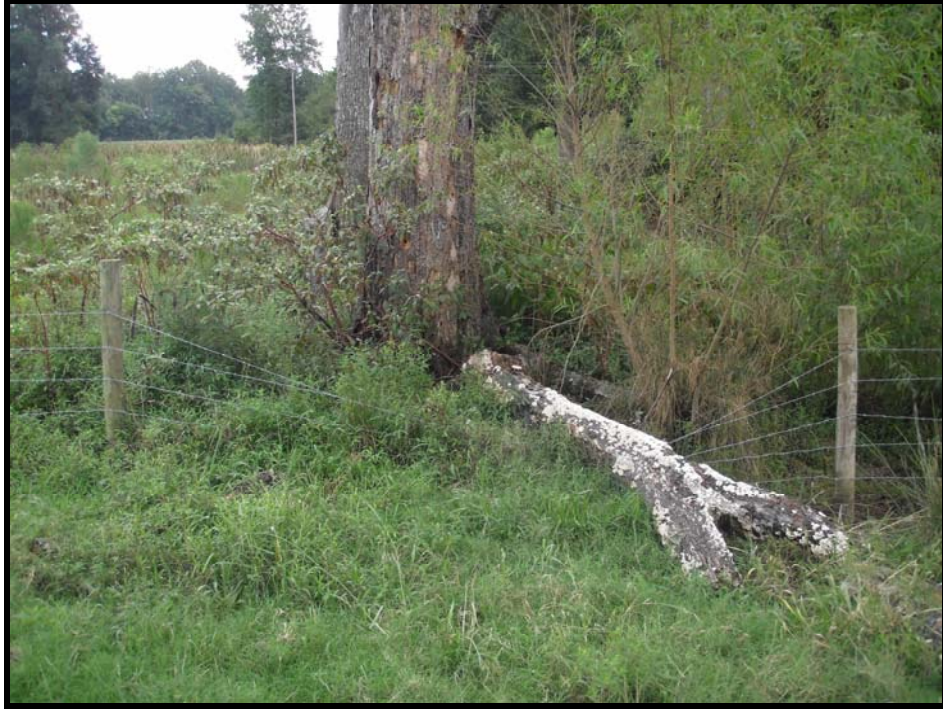
SOA3 – Easement fencing is down at Sta. 118+70 (UT1-B)
