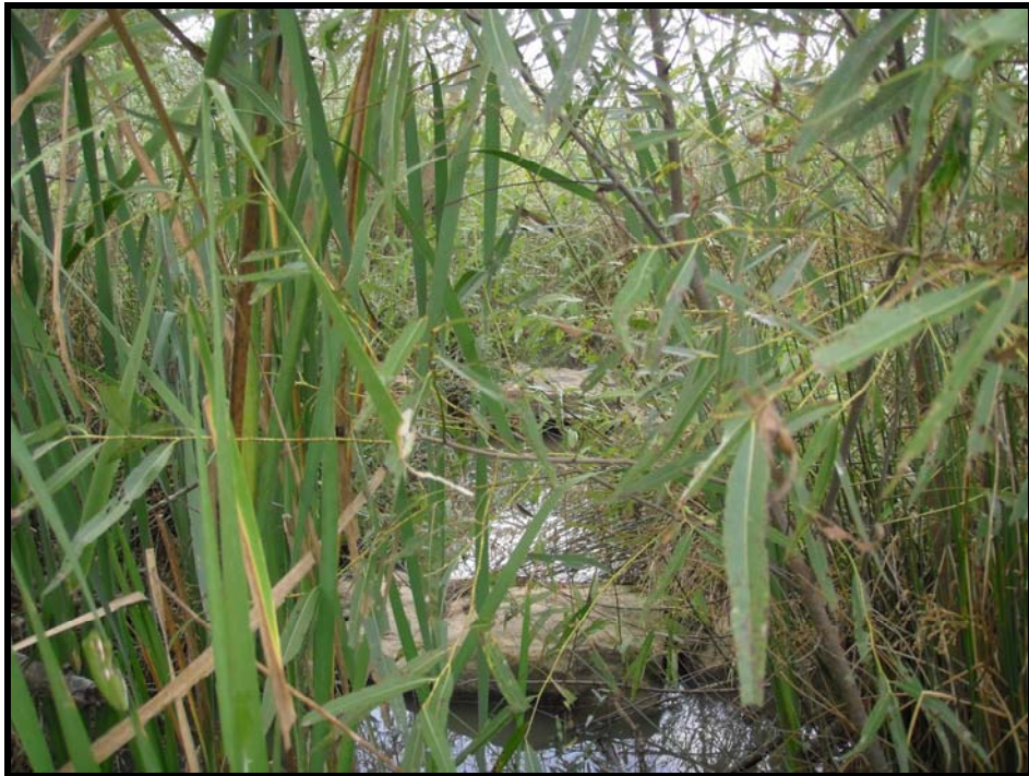
SOA4 – Piping around header rock on rock A-vane at Sta. 119+50 (UT1-B2)
