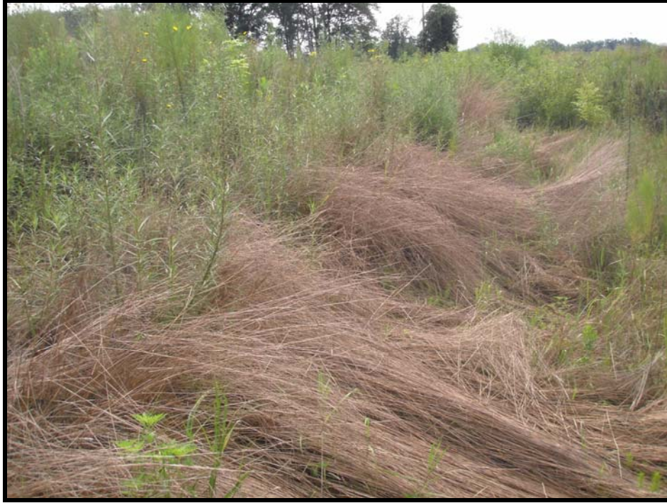
SOA5 – Minor rills and left bank erosion at Sta. 329+50 – 331+00 (UT3)
