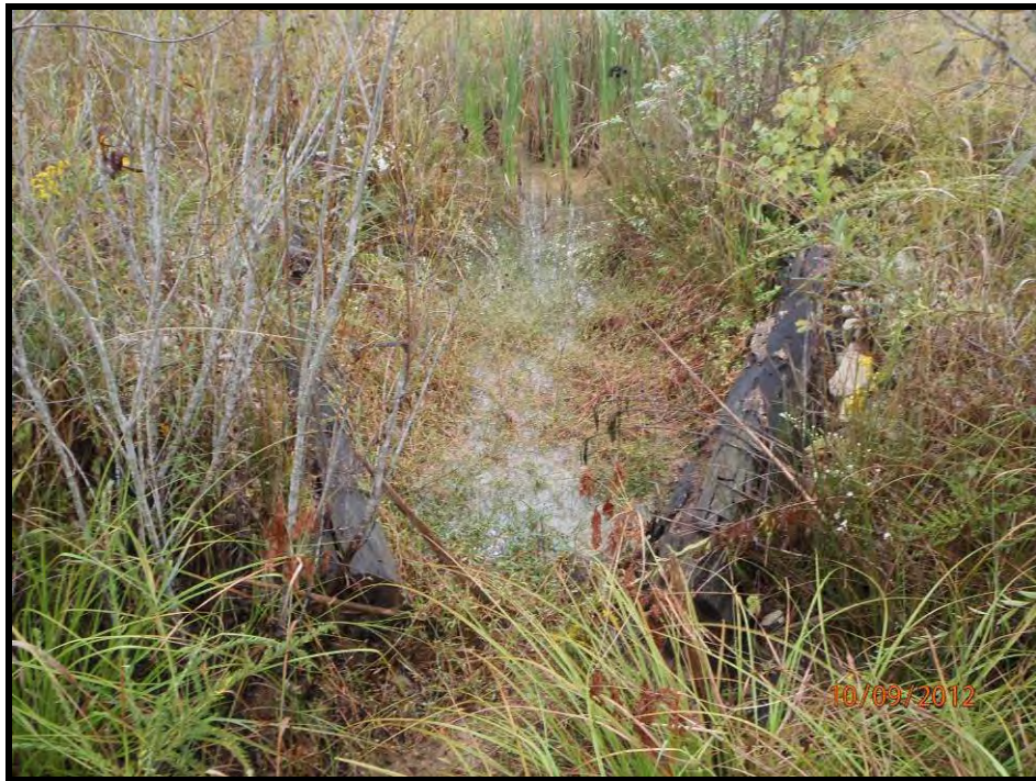
Log weir (typical)
