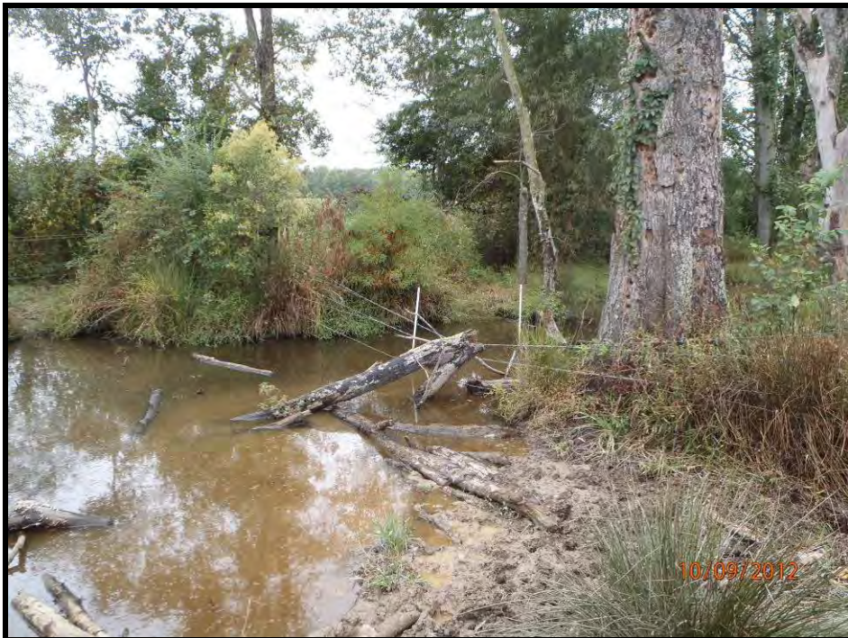
SOA2 – Easement fencing is loose at Sta. 118+90 (UT1-B)
