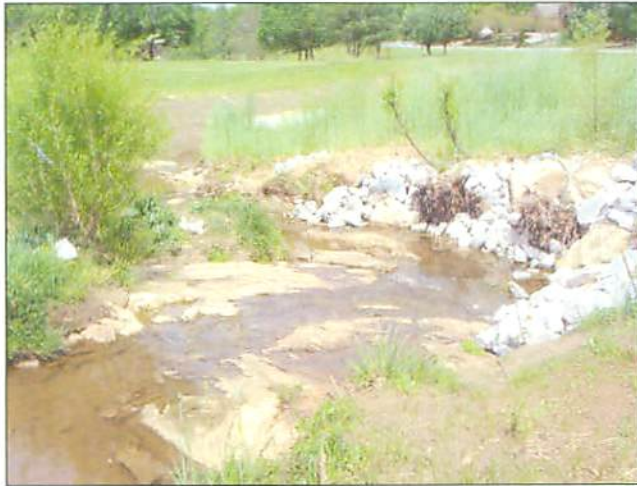
PP 25 Knick point with 90 degree bend with Root Wad Cluster #4, Transplants, and toe protection
