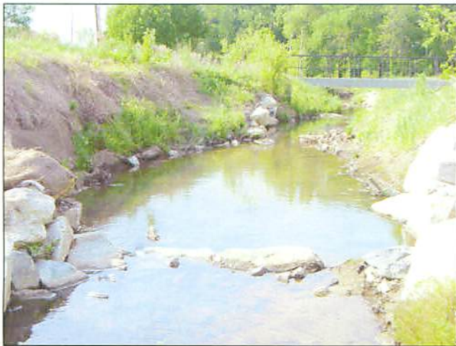
PP#19 R1 Double Drop Cross Vane #2
