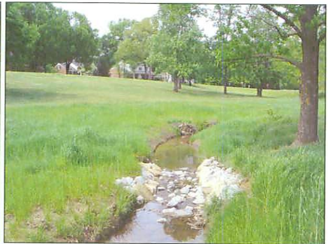
PP#35 Riffle #14, Root Wad Cluster #10, and Cross Section #4
