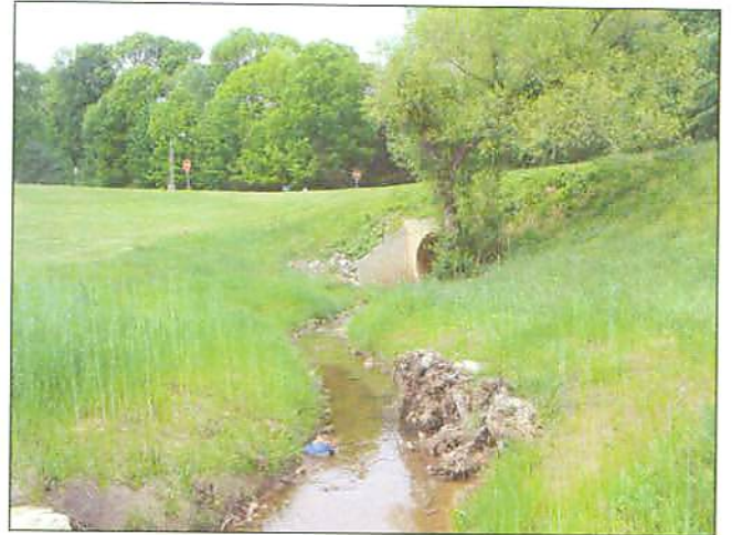
PP#41 Root Wad Cluster #16 into Culvert at Reach End
