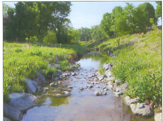
PP#10A R1 Toe protection on left bank into Constructed Riffle #2
