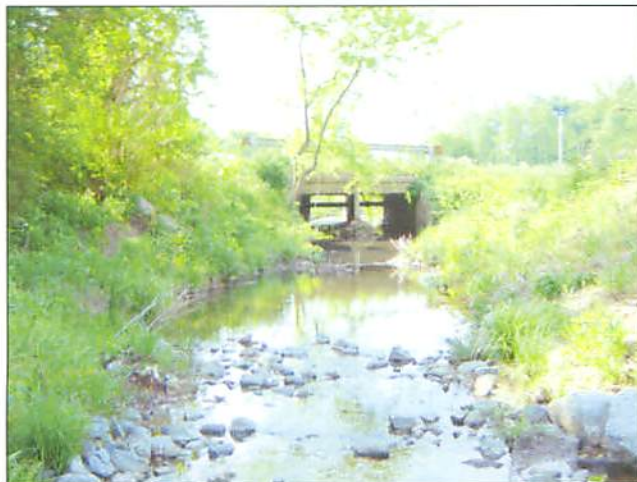
PP#14 R1 Constructed Riffle #4
