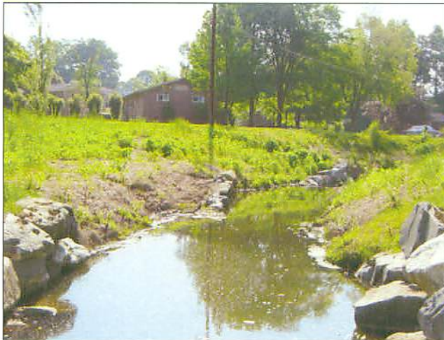
PP#38 R2 Double Drop Cross Vane #4
