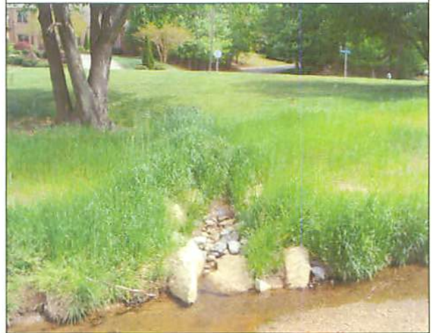
PP#31 Swale into Step Pool #7
