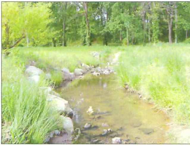
PP#30 R2 Rock Vane #4 and Constructed Riffle #3
