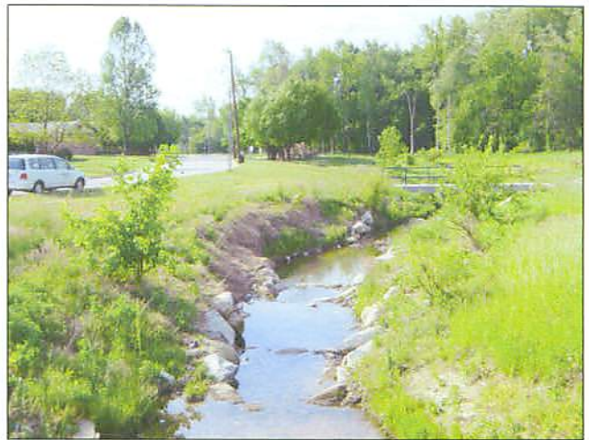
PP#17 R2 Downstream View from South Benbow Road
