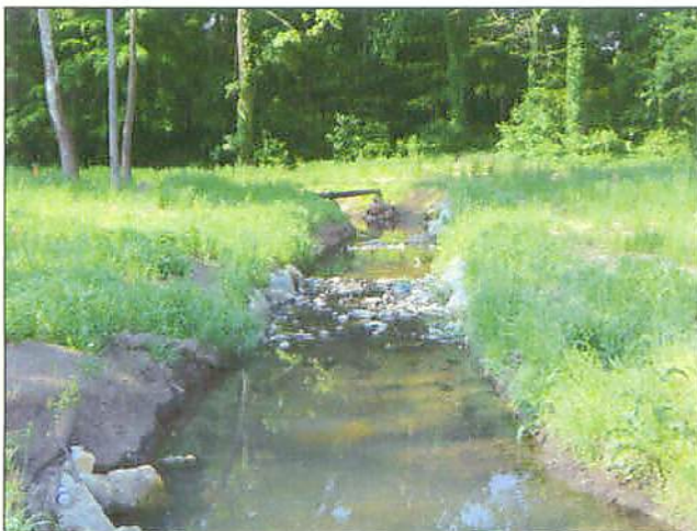
PP#35 R2 Constructed Riffle #5
