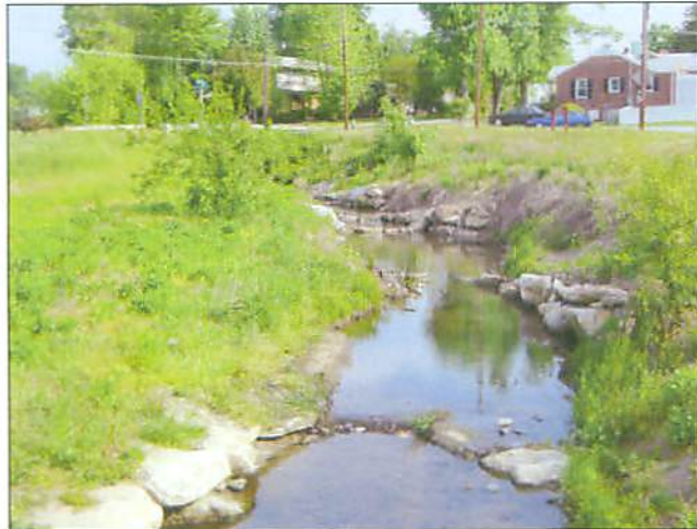
PP#23A R2 Upstream View from Pedestrian Bridge
