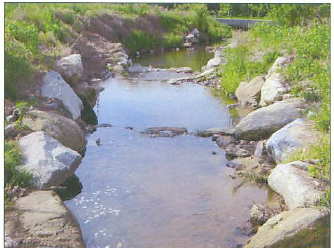
PP#18B R2 Double Drop Cross vane #1
