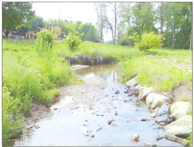
PP#29 R2 Constructed Riffle #2 and Root Wad Cluster #3
