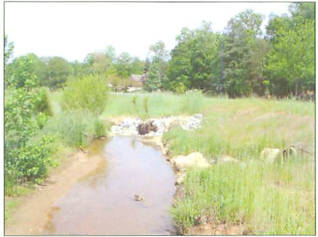
PP24 Run into Bedrock Knick point with 3 ft drop. Step Pool #5 on Right Bank
