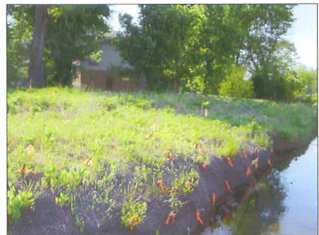
PP#11A R1 Bare-root and Live-stakes Plot #1
