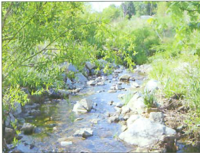
PP#3 R1 Constructed Riffle #1
