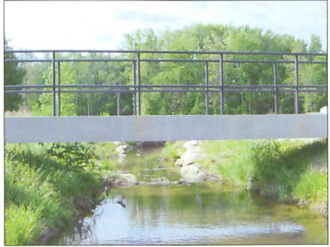
PP#22 R2 Newly Installed Pedestrian Bridge
