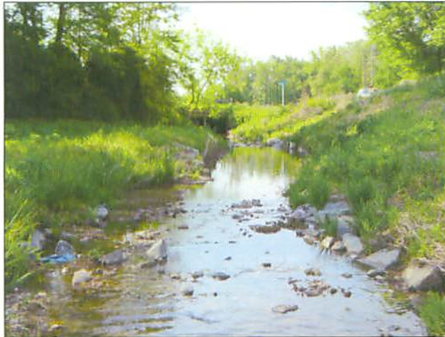
PP#12B R1 Constructed Riffle #3 and Cross Section #3
