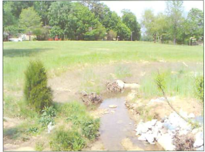
PP26 Root Wad Cluster #5 with toe protection
