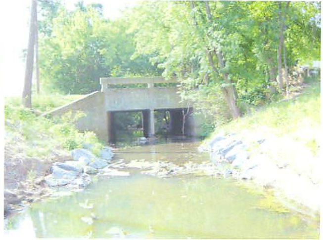
PP#43 R2 Toe protection and rock weir into culvert at end of R2
