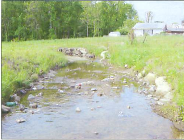
PP#26 R2 Constructed Riffle #1
