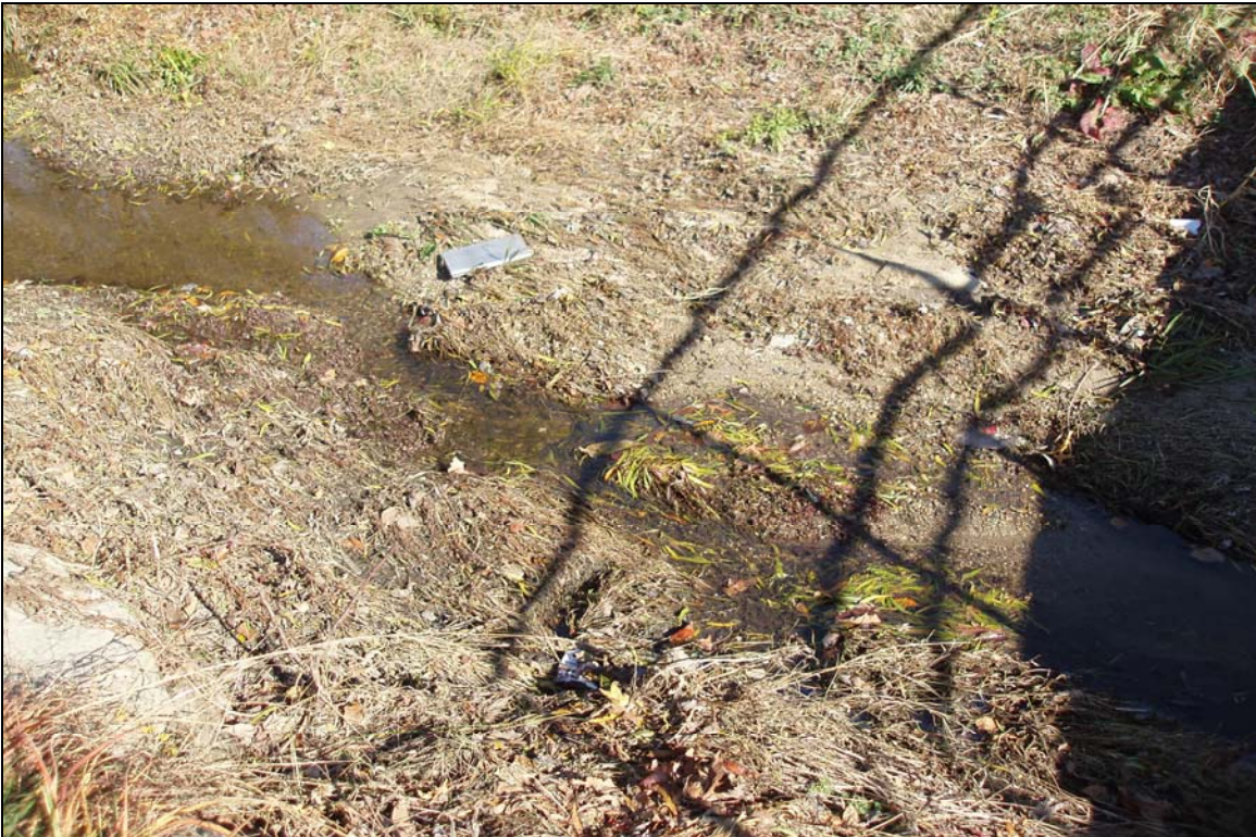
SP4 - Aggradation narrowing channel. Photo taken near Station 20+15. 11/16/07 - MY 03
