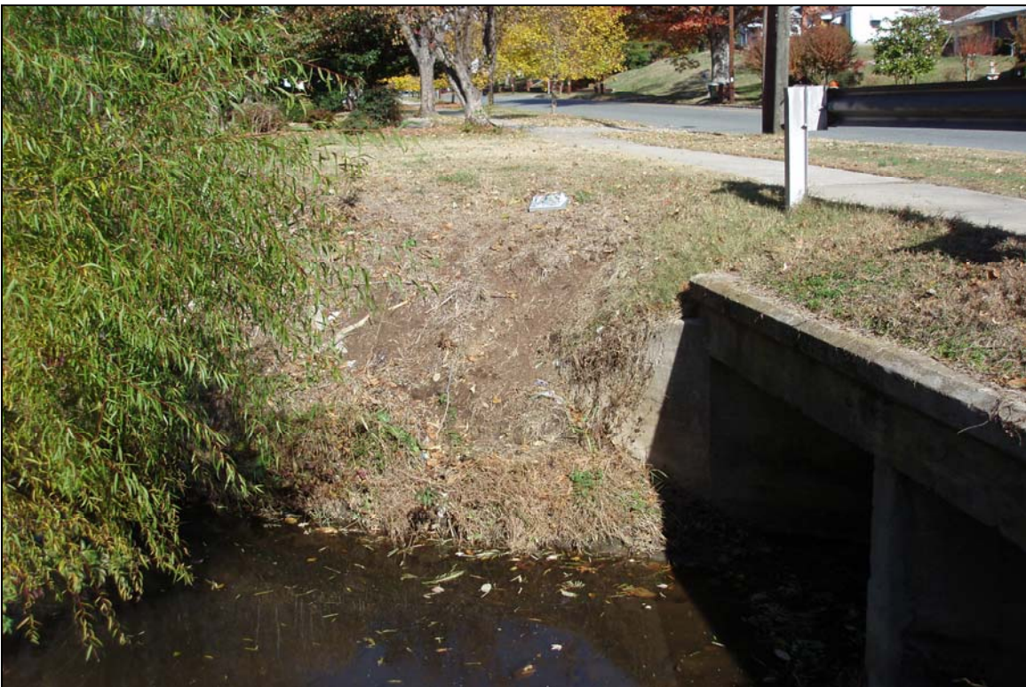
VP2 - Bare bank with coir matting exposed. Photo taken near Station 17+75. 11/16/07 - MY 03
