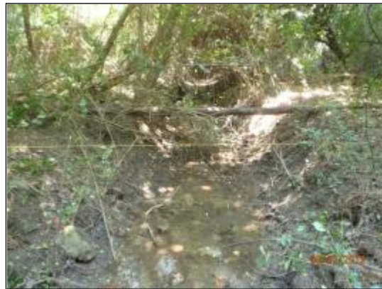
Facing downstream on UT6. 8/2/2012
