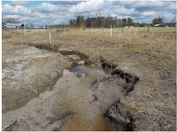
SPA2- Bank Erosion and Loose log structures- UT1 @ Sta. 15+90 to 16+80
