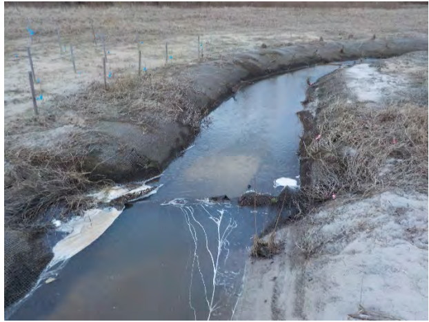
SPA4- Bank Erosion and Loose log structure- UT2 @ Sta. 25+50
