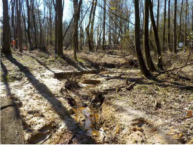
SPA6- Floodplain erosion/concentrated flow- UT4 @ Sta 10+25 to 11+00
