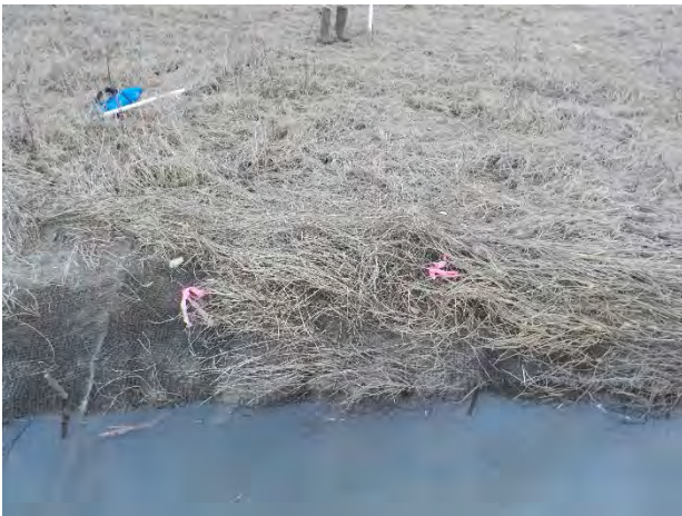
Bank Pin Array 8 UT2 STA 23+55 (2/9/2016)
