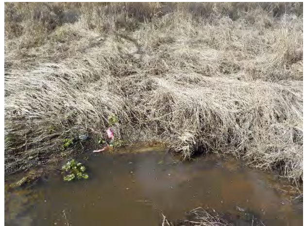
Bank Pin Array 4 UT1 STA 9+90 (2/9/2016)
