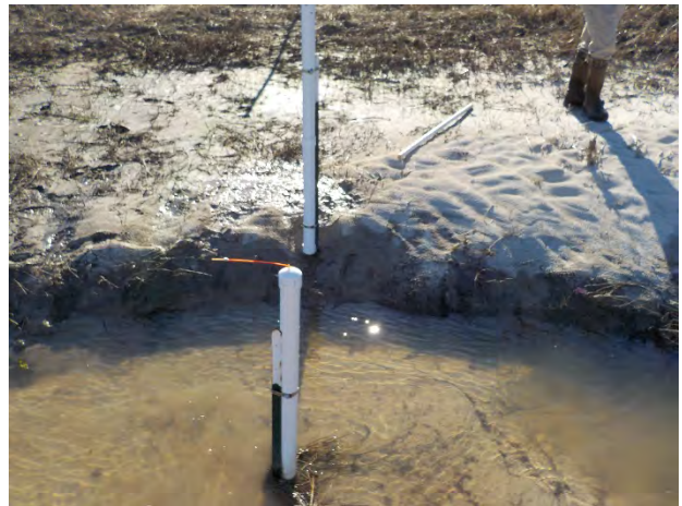
Bank Pin Array 8 UT2 STA 28+45 (2/9/2016)
