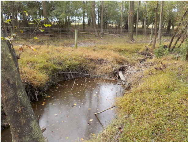
SPA3- Relic Channel Floodplain Erosion- UT4 @ Sta. 10+25 – 11+00
