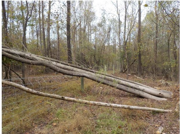
SPA4- Easement Fencing Damage- UT3 and UT4 (All damaged fence has been repaired)
