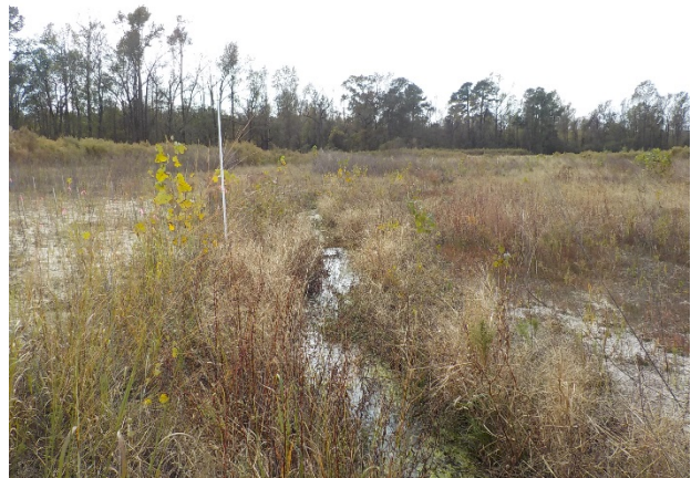
MY1 - SPA4- Bank Erosion and Loose log structures- UT2
