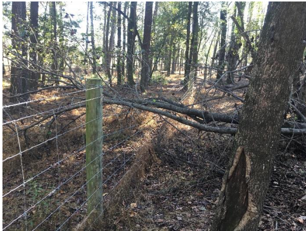
SPA1 – Fence Damage UT3 @ Sta. 7+50
