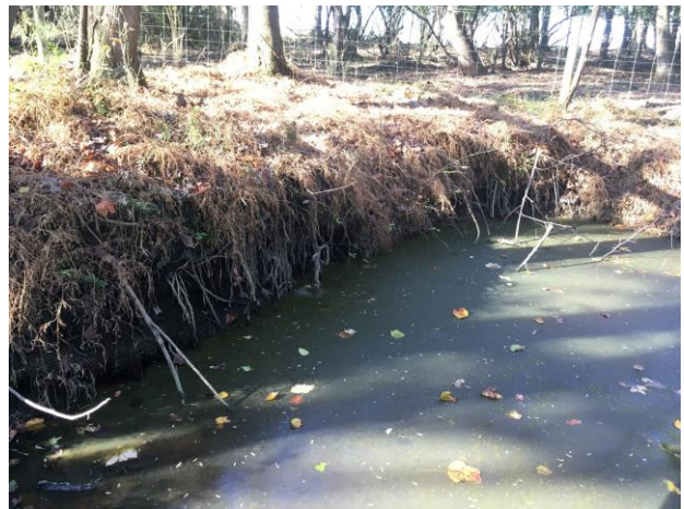
SPA4 – Relic Channel Floodplain Plug Subsidence UT4 @ Sta. 8+75 to 11+03
