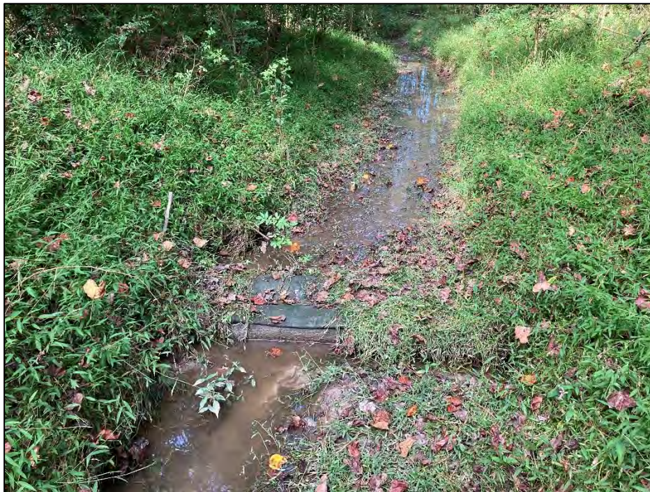
Photo 2 – Piping Log Sill UT6 (Repaired October 2020)
