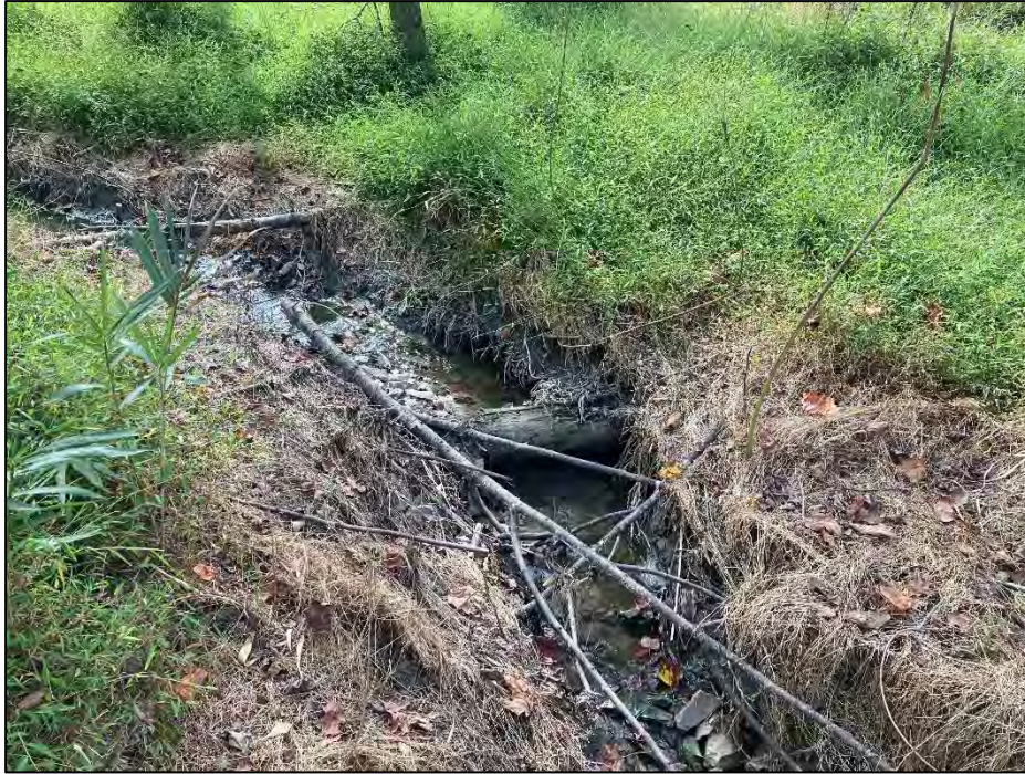
Photo 1 – Piping Log Sill UT4 (Repaired October 2020)
