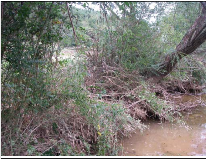
UT1. High shear stress forces cause bank instability, resulting in loss of bank vegetation.
