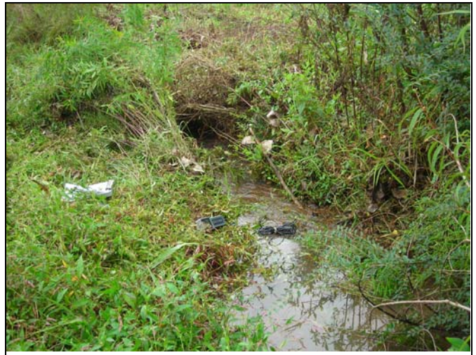
UT1 – below agricultural crossing. Continuous bed and bank disturbance resulted in a lack of bed definition.
