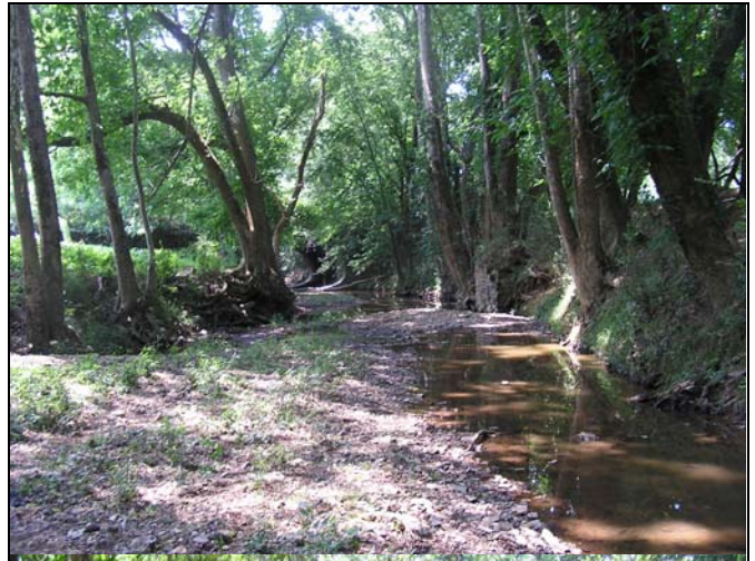
Big Cedar Creek – near Mount Zion Road culvert. Mass aggradation in overly wide channel.
