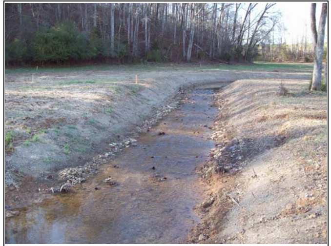
BCC PID 38 – Constructed Riffle, BCC Reach 2
