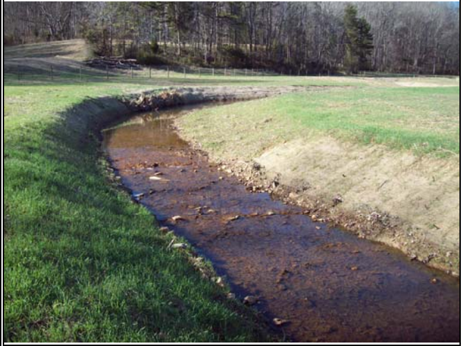
BCC PID 26 – Constructed Riffle, BCC Reach 2
