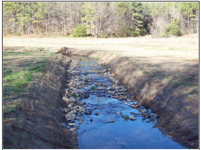
UT1 PID 16 – Constructed Riffle, UT1 Reach 3
