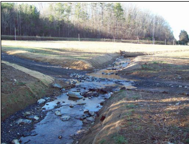
UT1 PID 5 – Riffle Crossing, UT1 Reach 4
