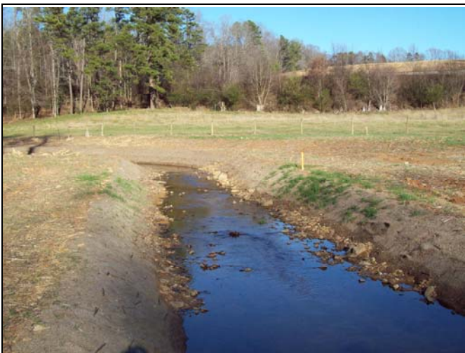
BCC PID 41 – Constructed Riffle, BCC Reach 1
