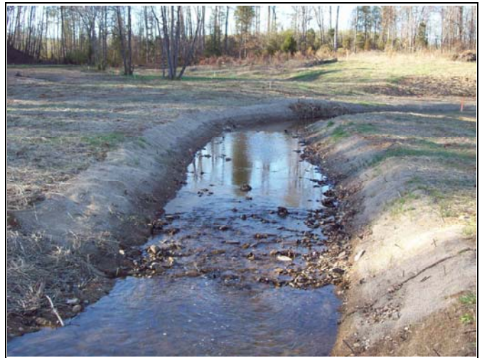
BCC PID 40 – Constructed Riffle, BCC Reach 1 End
