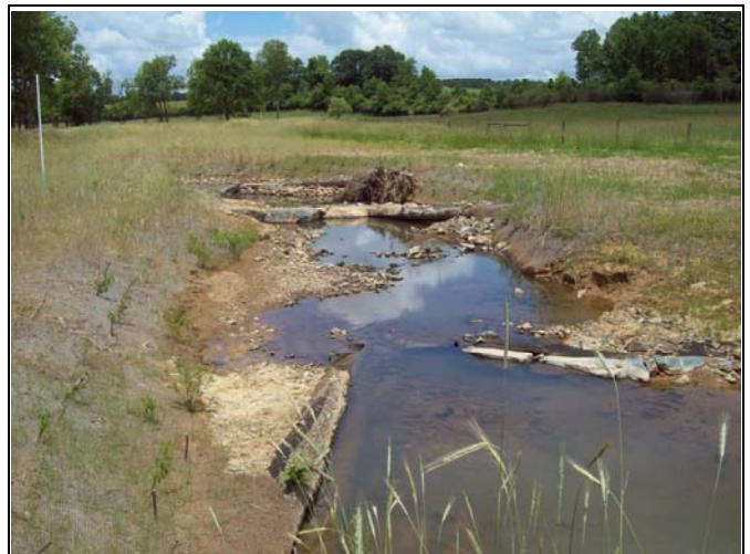
BCC PID 12 – Log J-Hook Step Pool, BCC Reach 3
