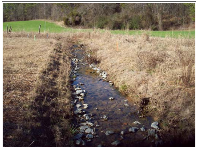
UT1 PID 48 – Constructed Riffle, UT1 Reach 1
