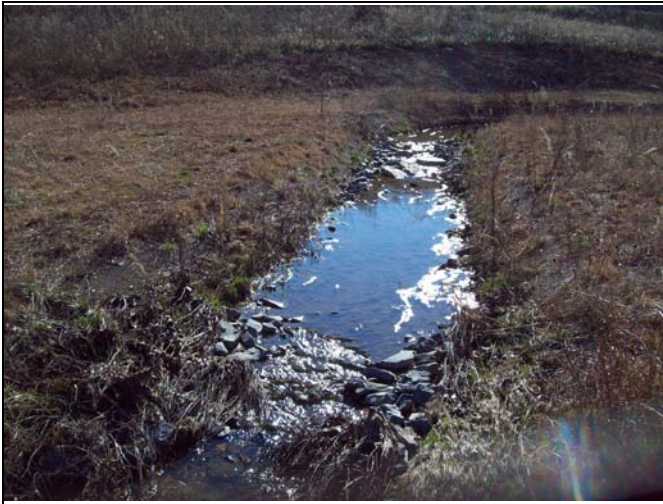
UT1 PID 49 – Constructed Riffle, UT1 Reach 1
