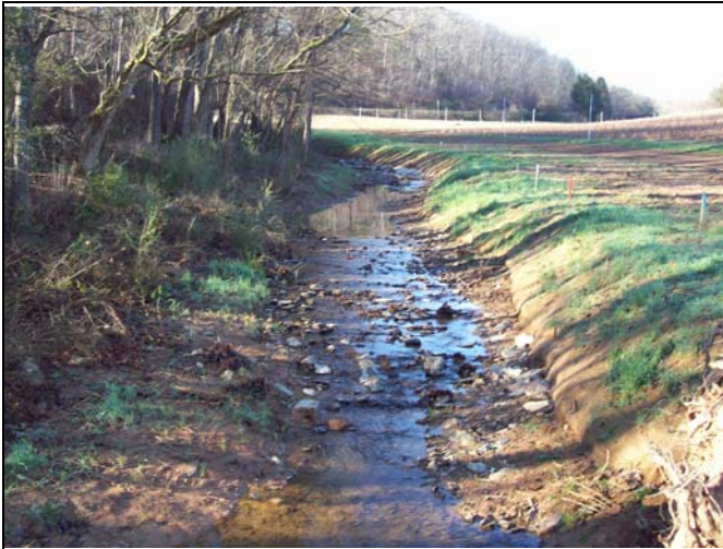
UT1 PID 3 – Constructed Riffle, UT1 Reach 4
