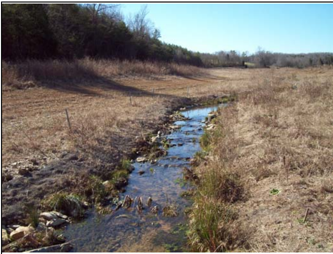
UT1 PID 33 – Constructed Riffle, UT1 Reach 2
