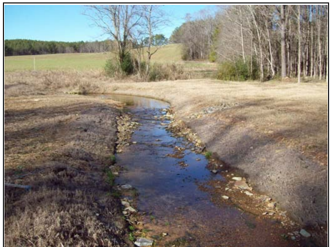
UT1 PID 30– Constructed Riffle, UT1 Reach 3 Start
