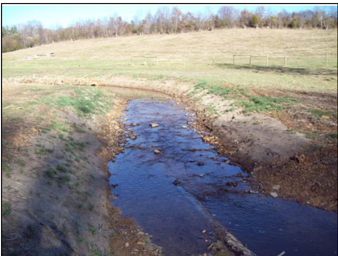
BCC PID 35 – Constructed Riffle, BCC Reach 2
