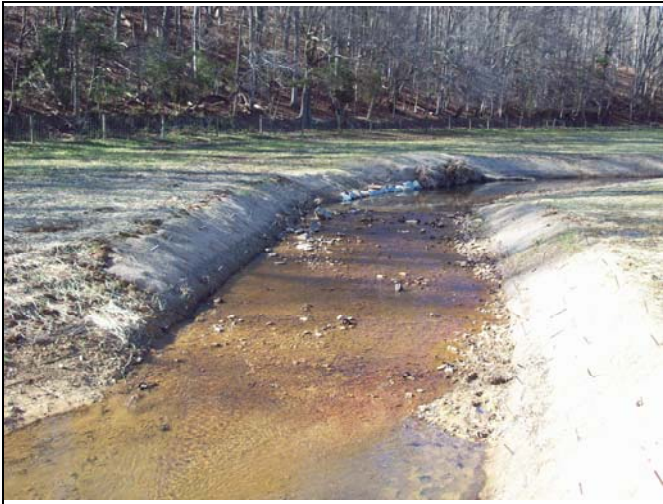
BCC PID 19 – Constructed Riffle, BCC Reach 3
