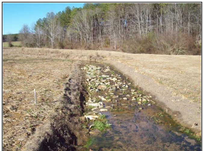
UT1 PID 24 – Constructed Riffle, UT1 Reach 3
