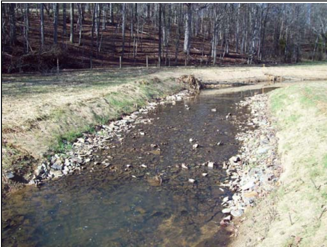
BCC PID 9 – Constructed Riffle, BCC Reach 4
