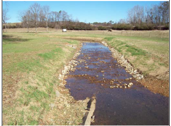
BCC PID 14 – Constructed Riffle, BCC Reach 3
