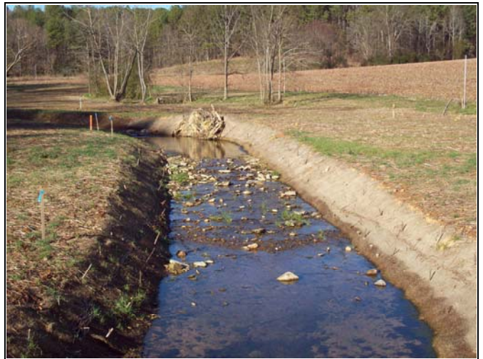
UT1 PID 10 – Constructed Riffle, UT1 Reach 4
