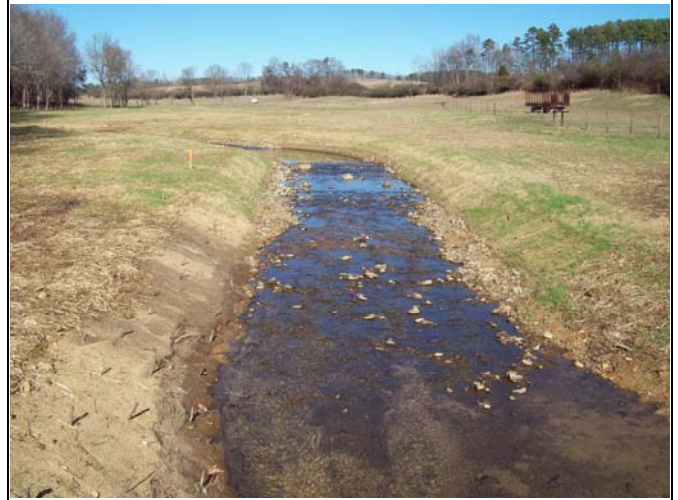
BCC PID 8 – Constructed Riffle, BCC Reach 4
