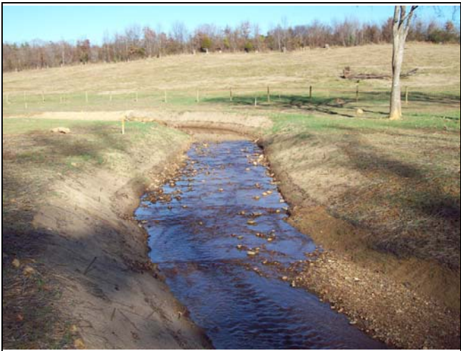
BCC PID 33 – Constructed Riffle, BCC Reach 2
