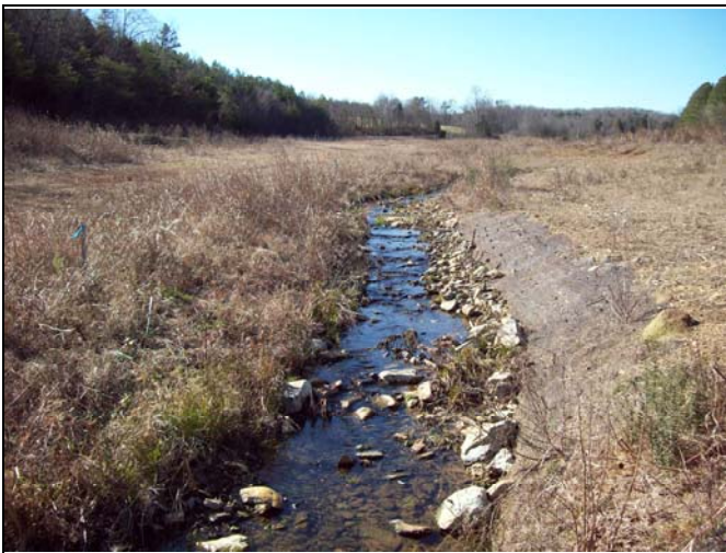
UT1 PID 35 – Constructed Riffle, UT1 Reach 2
