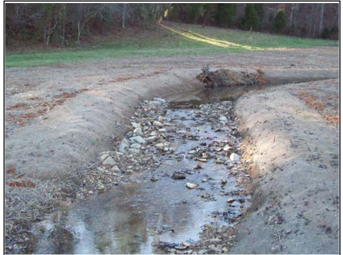
UT2 PID 4 – Constructed Riffle
