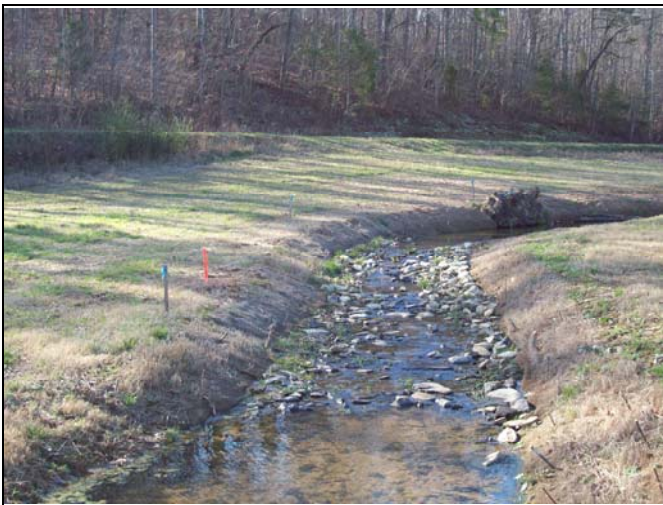
UT1 PID 17 – Constructed Riffle, UT1 Reach 3
