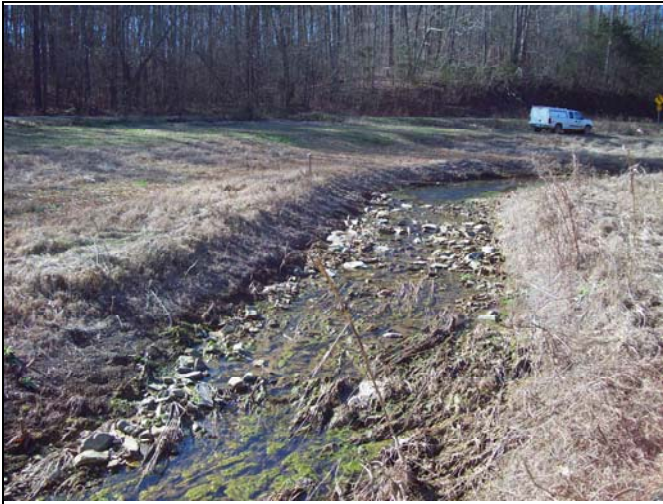
UT1 PID 25 – Constructed Riffle, UT1 Reach 3
