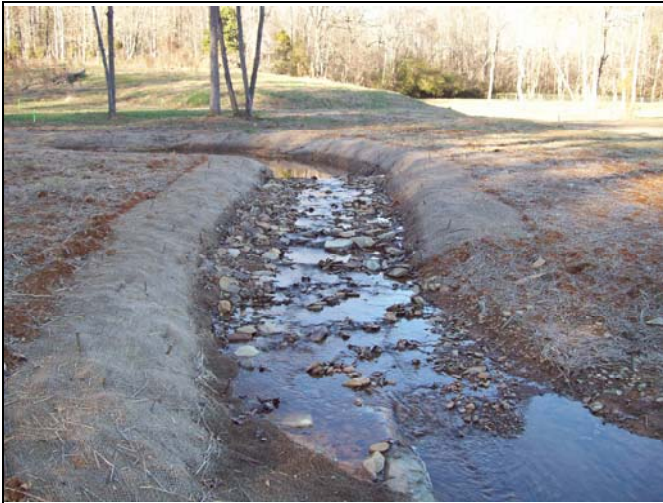
UT2 PID 3 – Constructed Riffle
