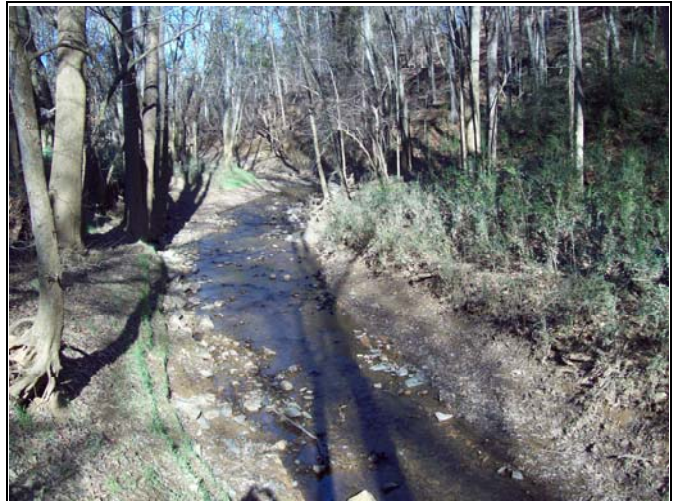
BCC PID 4 – Re-graded Riffle, BCC Reach 6
