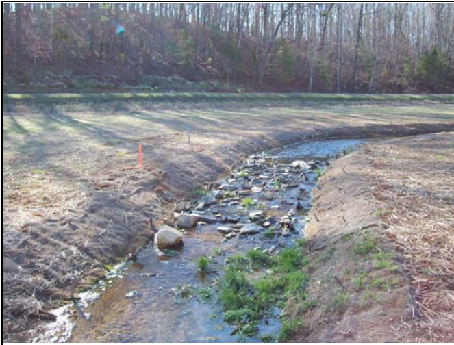
UT1 PID 19 – Constructed Riffle, UT1 Reach 3
