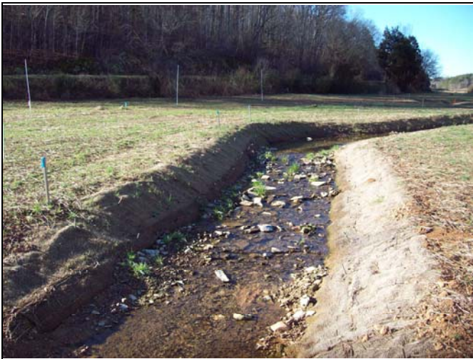
UT1 PID 9 – Constructed Riffle, UT1 Reach 4
