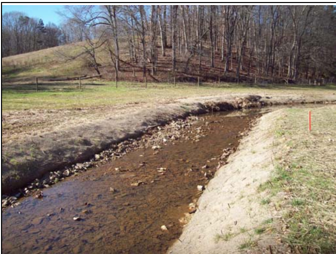
BCC PID 17 – Constructed Riffle, UT1 Reach 3
