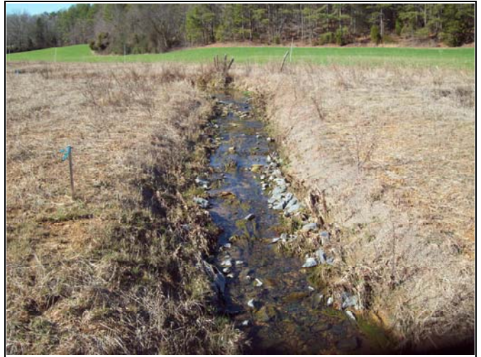
UT1 PID 44 – Constructed Riffle, UT1 Reach 1
