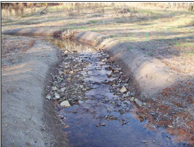
UT2 PID 5 – Constructed Riffle
