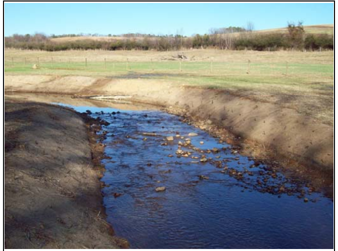
BCC PID 20 – Constructed Riffle, BCC Reach 3
