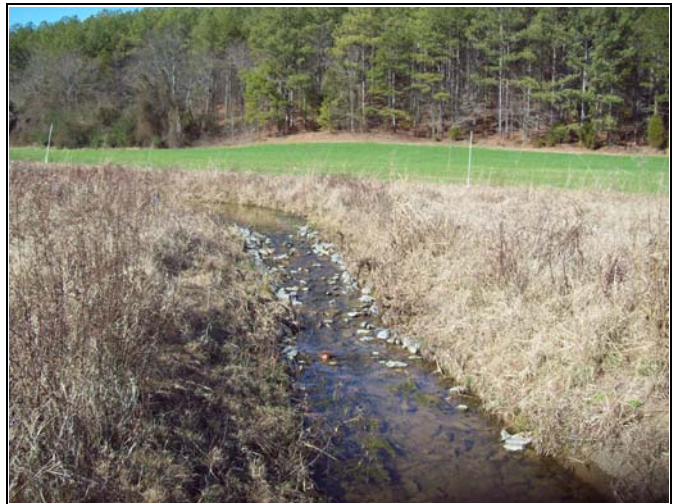
UT1 PID 46 – Constructed Riffle, UT1 Reach 1
