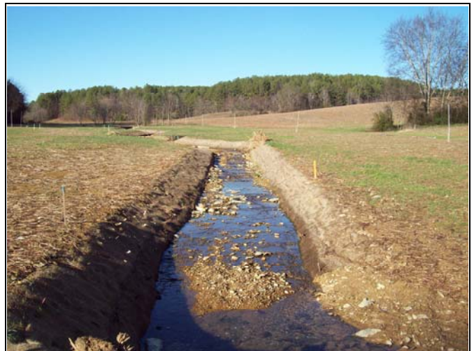
UT1 PID 6 – Constructed Riffle, UT1 Reach 4
