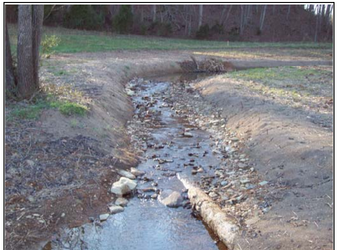
UT2 PID 6 – Constructed Riffle
