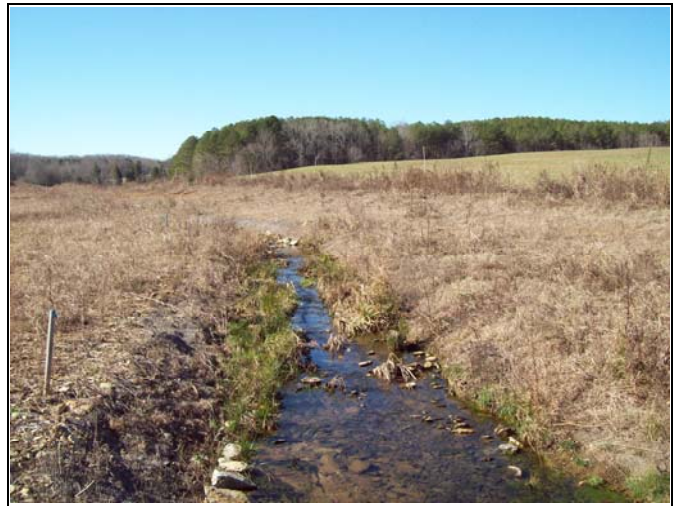
UT1 PID 34 – Constructed Riffle, UT1 Reach 2
