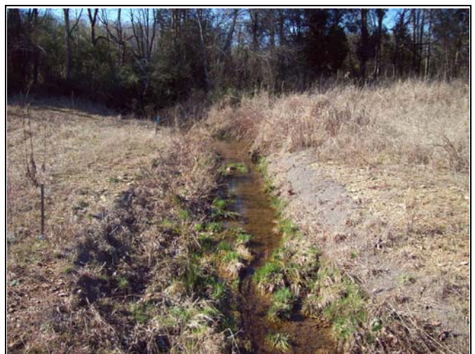
UT1 PID 54 – Constructed Riffle, UT1 Reach 1 Start
