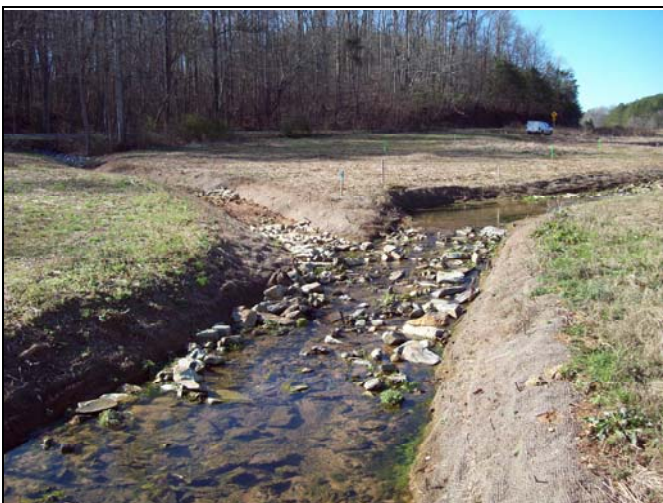
UT1 PID 23 – Constructed Riffle, UT1 Reach 3
