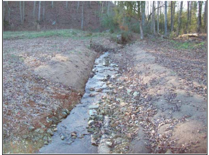
UT2 PID 8 – Constructed Riffle, UT2 Start
