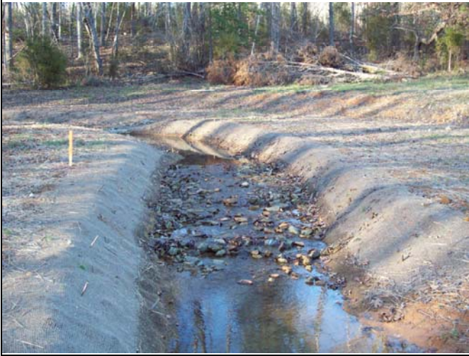
UT2 PID 7 – Constructed Riffle
