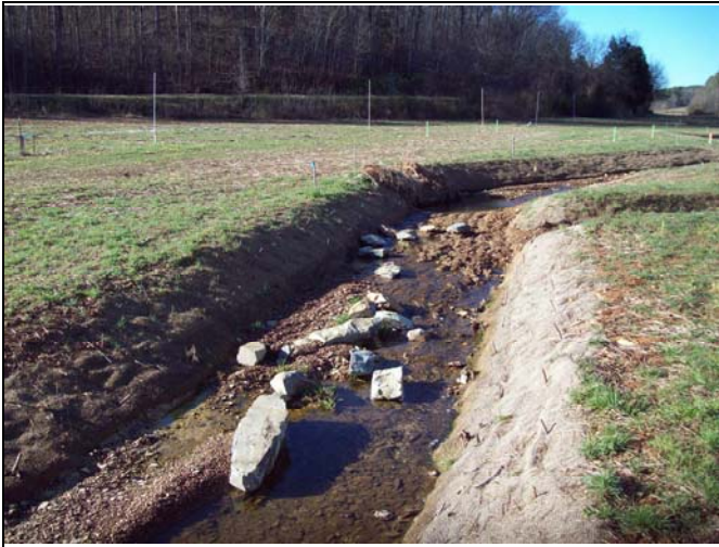
UT1 PID 7 – Constructed Riffle, UT1 Reach 4
