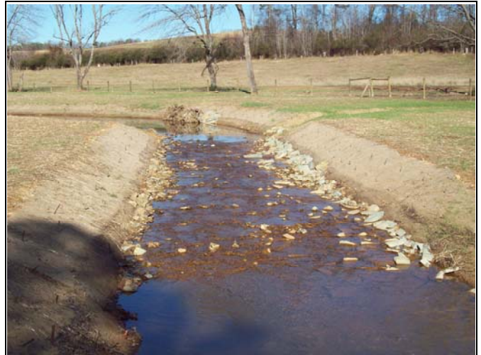
BCC PID 16 – Constructed Riffle, BCC Reach 3
