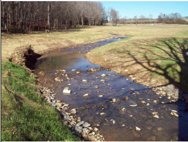
BCC PID 7 – Constructed Riffle, BCC Reach 4 End
