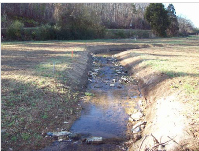
UT1 PID 11 – Constructed Riffle, UT1 Reach 4 Start
