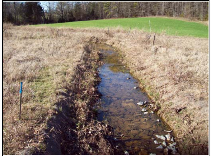
UT1 PID 50 – Constructed Riffle, UT1 Reach 1
