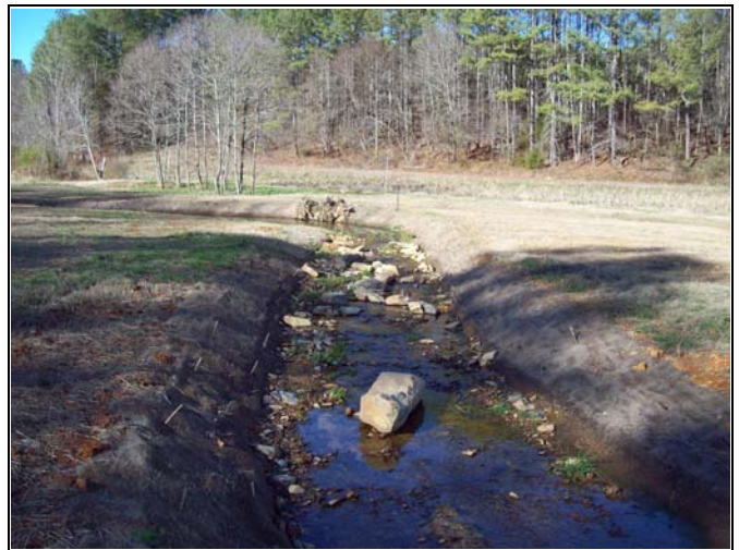
UT1 PID 18 – Constructed Riffle, UT1 Reach 3
