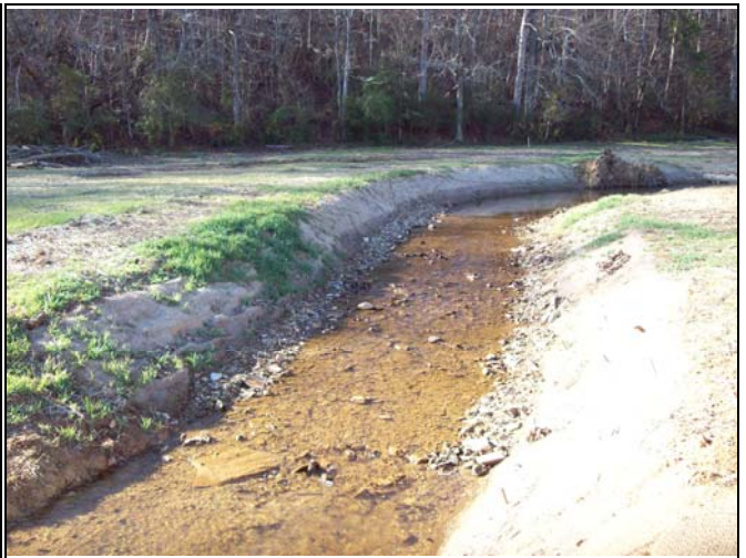
BCC PID 34 – Constructed Riffle, BCC Reach 2
