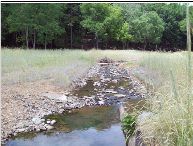
BCC PID 11 – Log J-Hook & Constructed Riffle , BCC Reach 3 End
