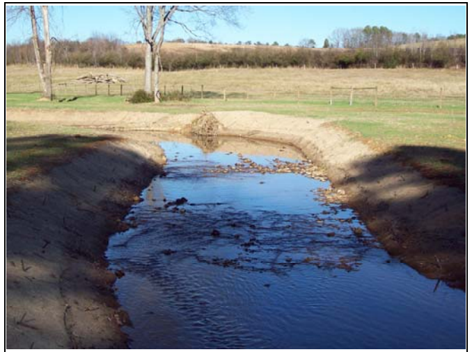
BCC PID 22 – Constructed Riffle, BCC Reach 3
