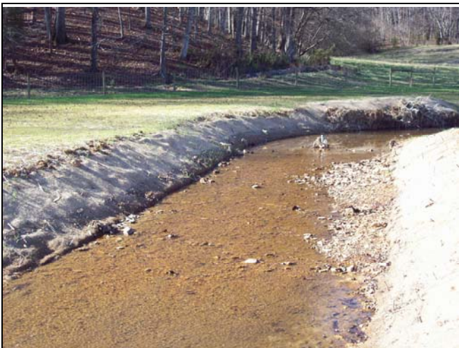
BCC PID 23 – Constructed Riffle, BCC Reach 3 Start
