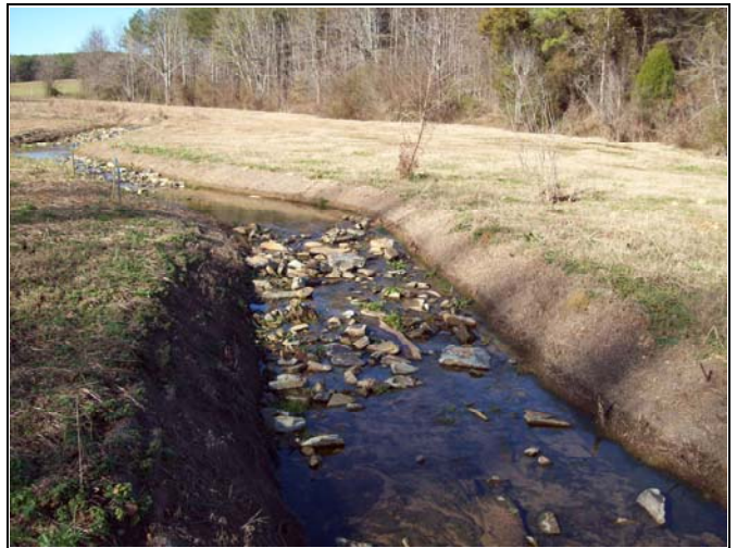
UT1 PID 22 – Constructed Riffle, UT1 Reach 3
