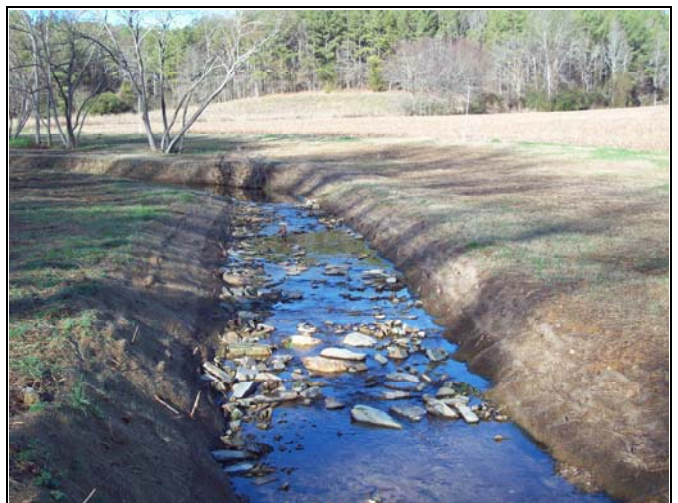
UT1 PID 12 – Constructed Riffle, UT1 Reach 3 End
