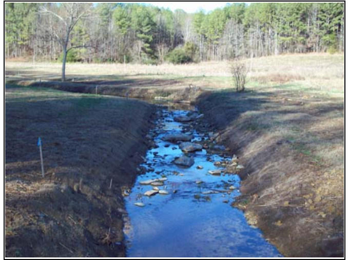
UT1 PID 14 – Constructed Riffle, UT1 Reach 3
