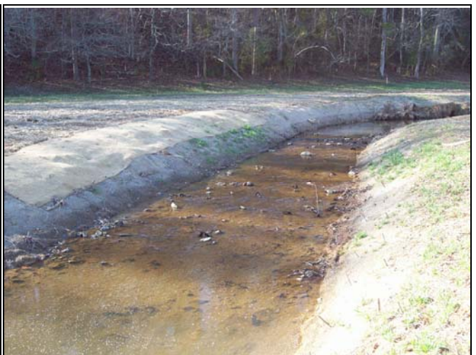
BCC PID 36 – Constructed Riffle, BCC Reach 2
