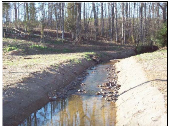
BCC PID 42 – Constructed Riffle, BCC Reach 1 Start
