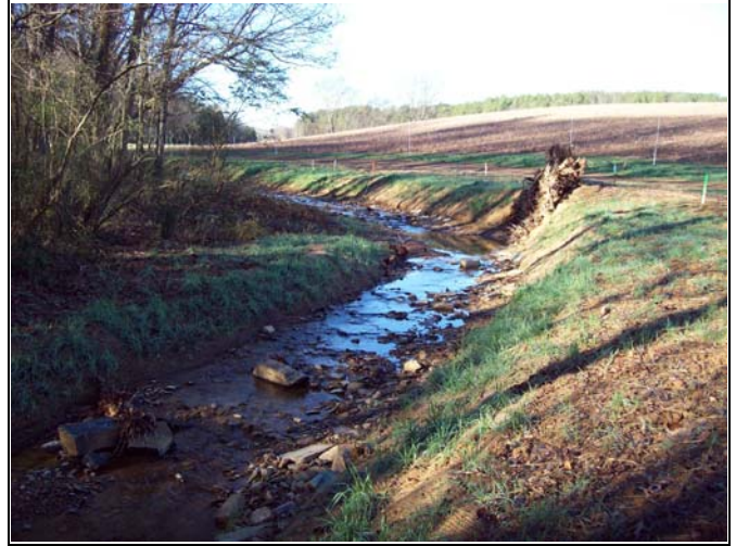
UT1 PID 2 – Constructed Riffle, UT1 Reach 4
