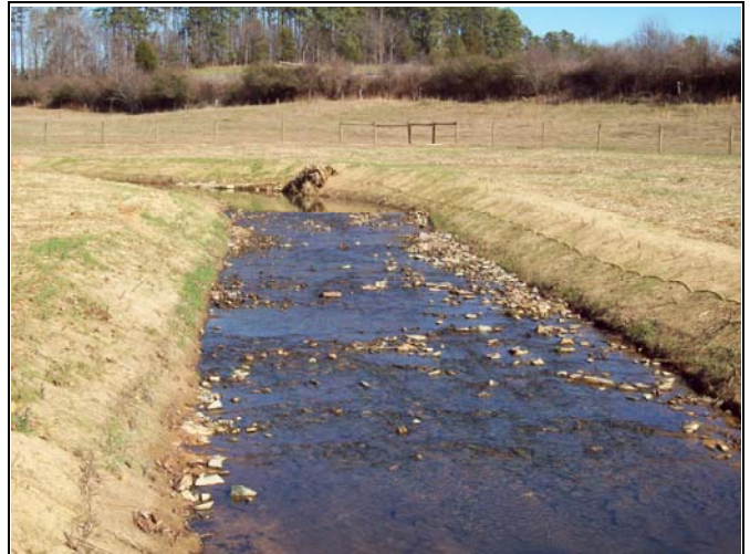
BCC PID 10 – Constructed Riffle, BCC Reach 4 Start
