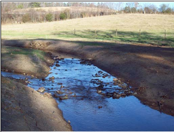
BCC PID 39 – Constructed Riffle, BCC Reach 2 Start
