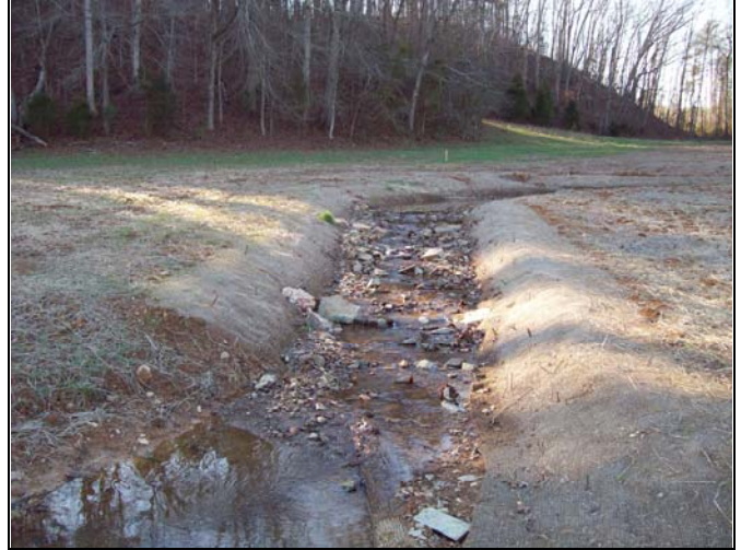
UT2 PID 2 – Constructed Riffle
