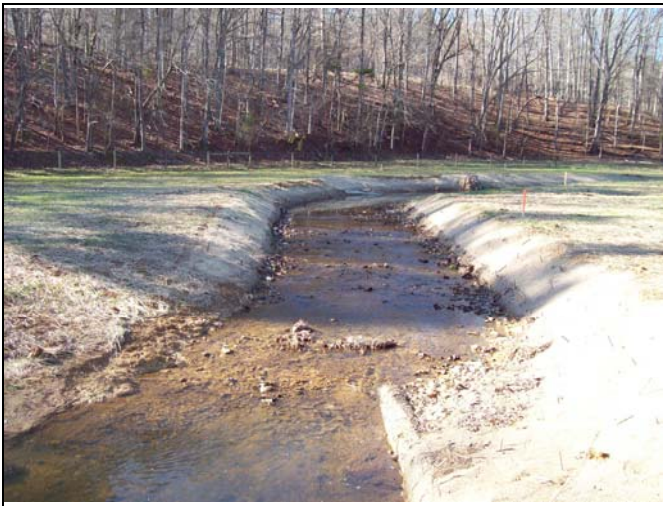
BCC PID 21 – Constructed Riffle, BCC Reach 3
