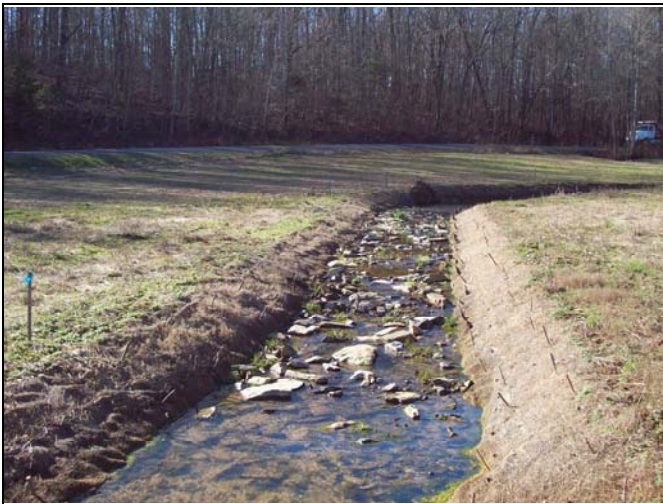
UT1 PID 21 – Constructed Riffle, UT1 Reach 3
