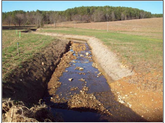
UT1 PID 8 – Constructed Riffle, UT1 Reach 4
