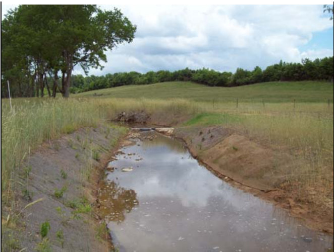
BCC PID 29 – Log J-Hook & Constructed Riffle, BCC Reach 2
