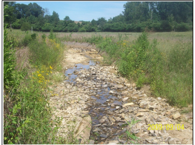
BCC PID 14 – Constructed Riffle, BCC Reach 3
