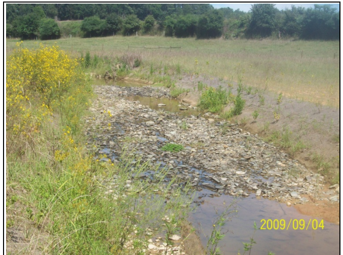
BCC PID 10 – Constructed Riffle, BCC Reach 4 Start
