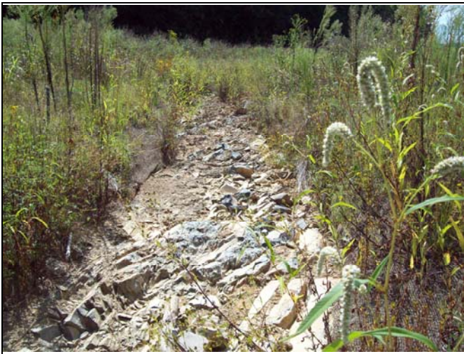
UT1 PID 27 – Constructed Riffle, UT1 Reach 3
