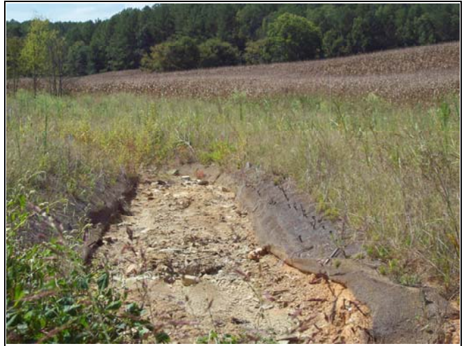
UT1 PID 8 – Constructed Riffle, UT1 Reach 4
