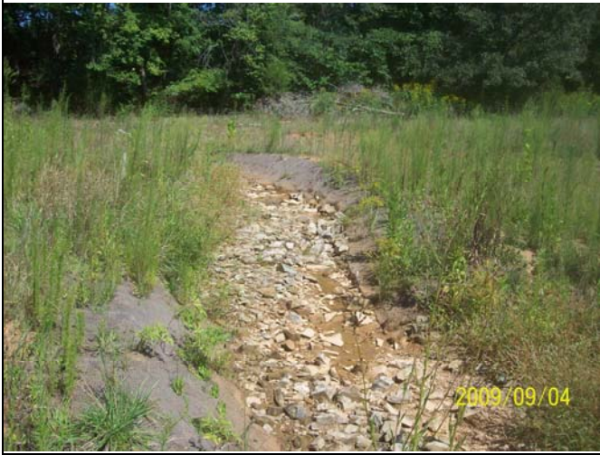
UT2 PID 7 – Constructed Riffle
