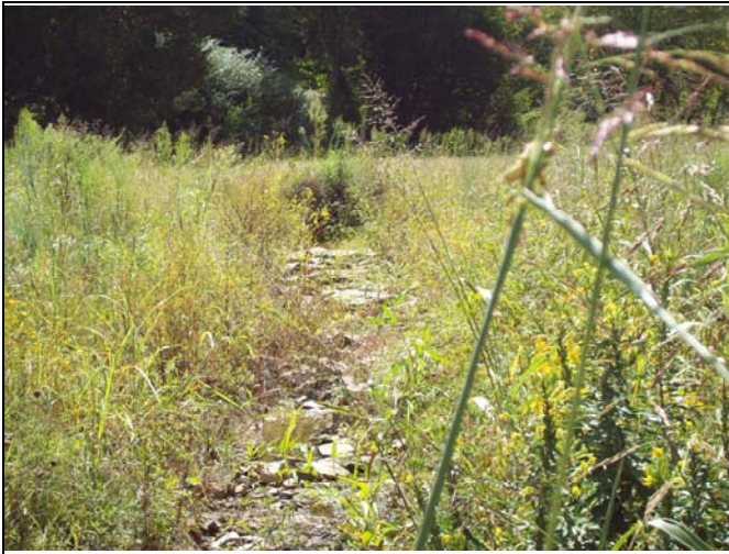
UT1 PID 13 – Constructed Riffle, UT1 Reach 3
