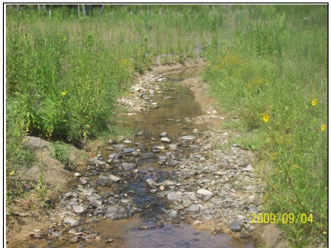
BCC PID 40 – Constructed Riffle, BCC Reach 1 End
