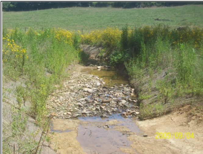
BCC PID 33 – Constructed Riffle, BCC Reach 2
