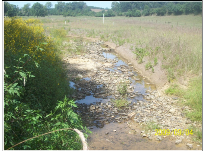
BCC PID 8 – Constructed Riffle, BCC Reach 4
