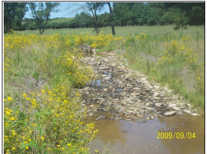
BCC PID 16 – Constructed Riffle, BCC Reach 3
