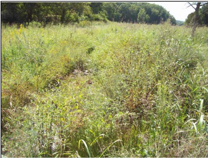
UT1 PID 15 – Constructed Riffle, UT1 Reach 3
