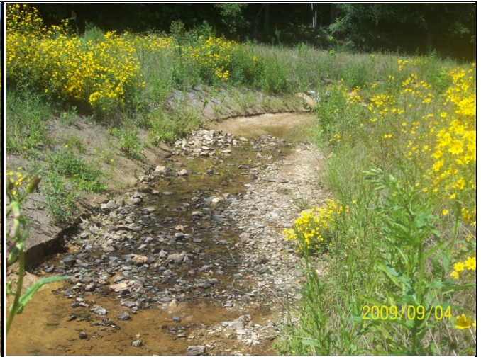
BCC PID 32 – Constructed Riffle, BCC Reach 2
