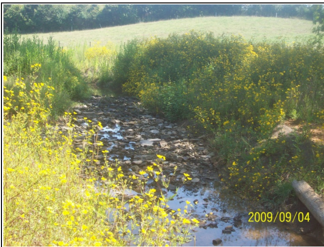
BCC PID 39 – Constructed Riffle, BCC Reach 2 Start
