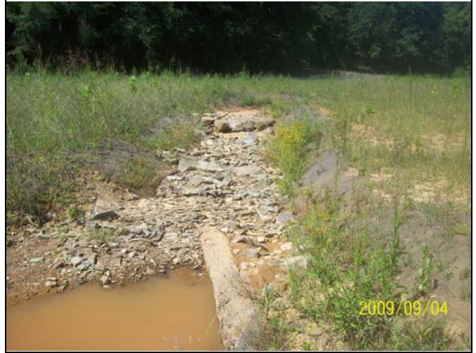
UT2 PID 2 – Constructed Riffle
