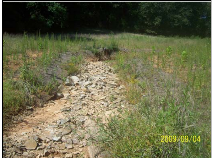
UT2 PID 4 – Constructed Riffle
