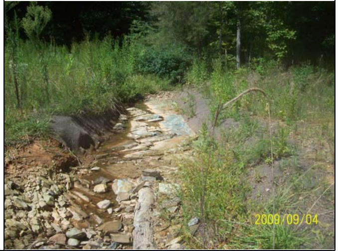
UT2 PID 8 – Constructed Riffle, UT2 Start
