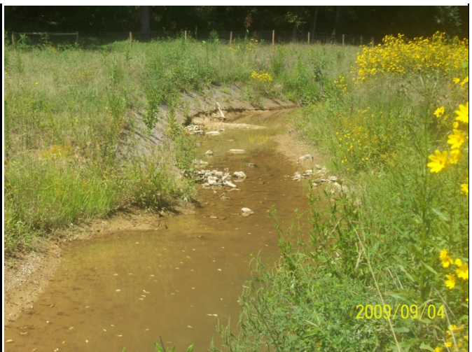
BCC PID 30 – Constructed Riffle, BCC Reach 2
