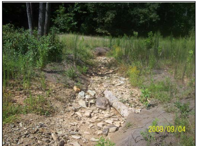
UT2 PID 6 – Constructed Riffle
