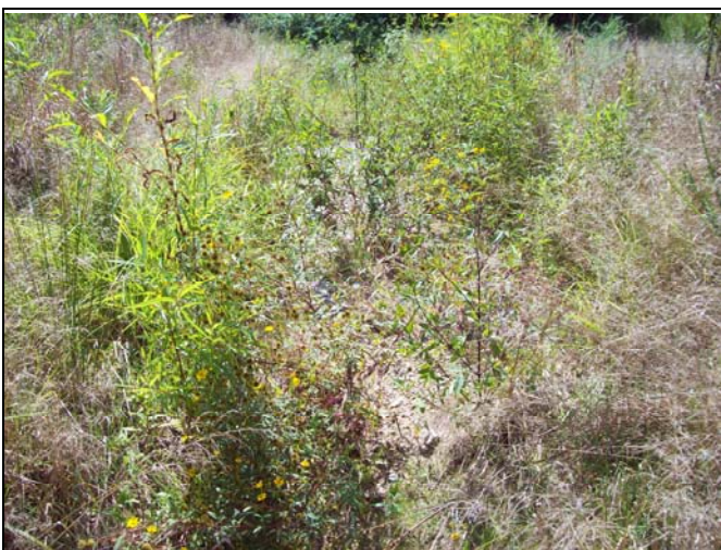
UT1 PID 47 – Constructed Riffle, UT1 Reach 1
