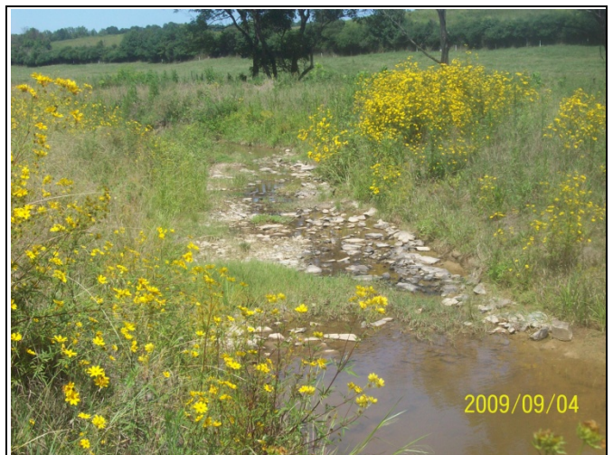
BCC PID 18 – Constructed Riffle, BCC Reach 3
