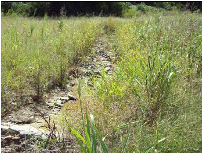
UT1 PID 11 – Constructed Riffle, UT1 Reach 4 Start
