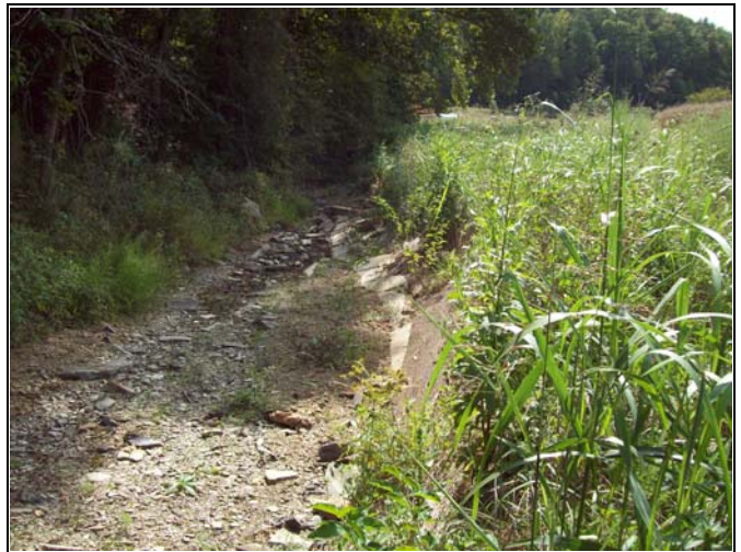
UT1 PID 4 – Constructed Riffle, UT1 Reach 4
