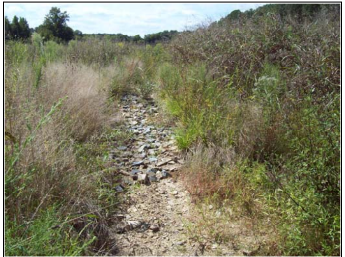
UT1 PID 40 – Constructed Riffle, UT1 Reach 2
