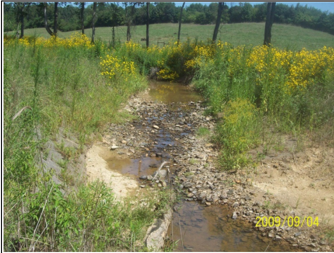
BCC PID 31 – Constructed Riffle, BCC Reach 2
