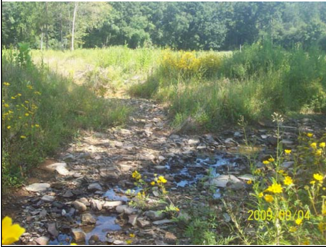
UT2 PID 1 – Constructed Riffle, UT2 End
