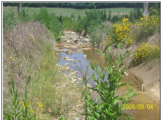
BCC PID 24 – Constructed Riffle, BCC Reach 2 End
