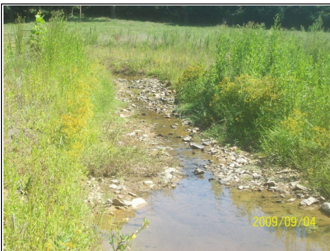
BCC PID 41 – Constructed Riffle, BCC Reach 1
