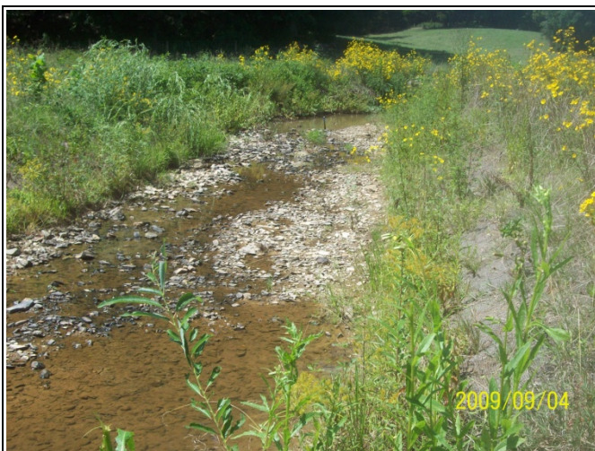
BCC PID 23 – Constructed Riffle, BCC Reach 3 Start
