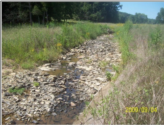
BCC PID 15 – Constructed Riffle, BCC Reach 3
