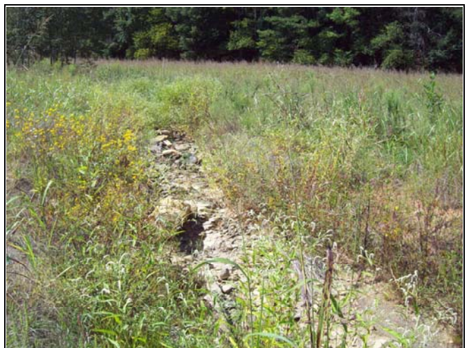
UT1 PID 18 – Constructed Riffle, UT1 Reach 3
