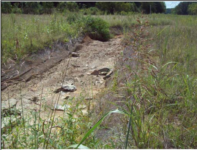
UT1 PID 7 – Constructed Riffle, UT1 Reach 4
