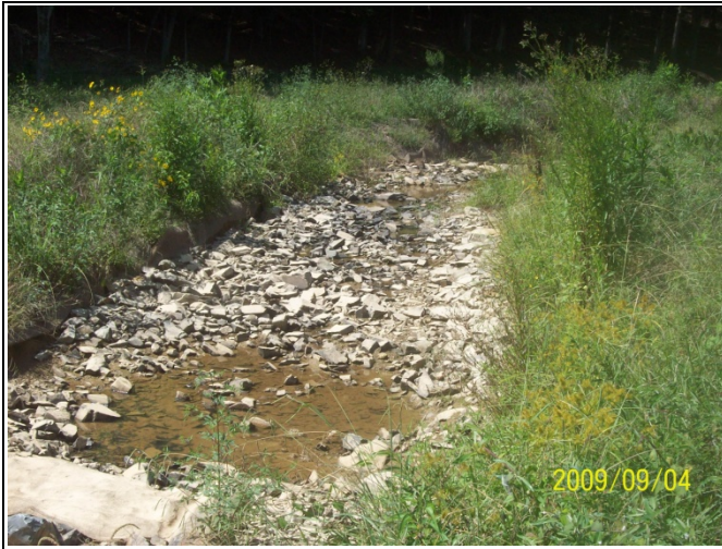
BCC PID 13 – Log J-Hook & Constructed Riffle, BCC Reach 3
