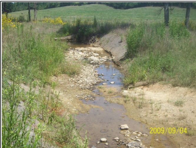
BCC PID 27 – Constructed Riffle, BCC Reach 2
