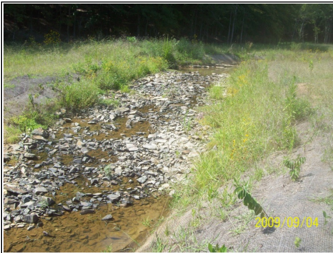
BCC PID 9 – Constructed Riffle, BCC Reach 4
