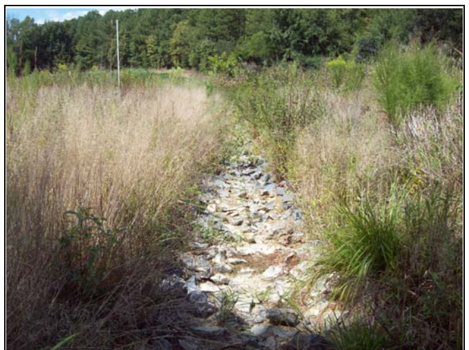
UT1 PID 48 – Constructed Riffle, UT1 Reach 1
