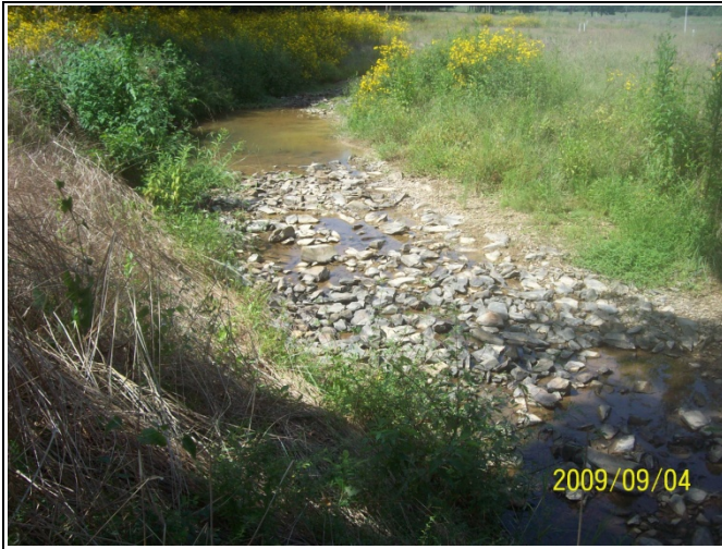
BCC PID 7 – Constructed Riffle, BCC Reach 4 End
