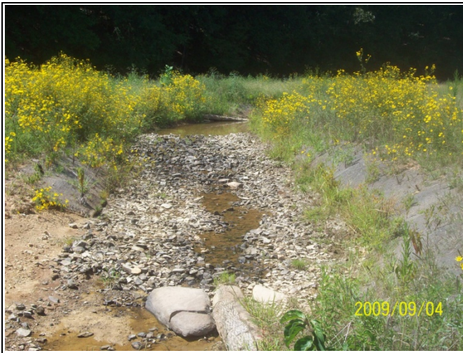
BCC PID 21 – Constructed Riffle, BCC Reach 3
