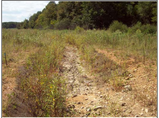
UT1 PID 20 – Constructed Riffle, UT1 Reach 3
