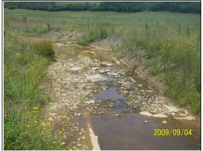
BCC PID 20 – Constructed Riffle, BCC Reach 3
