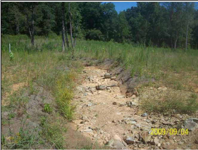
UT2 PID 3 – Constructed Riffle
