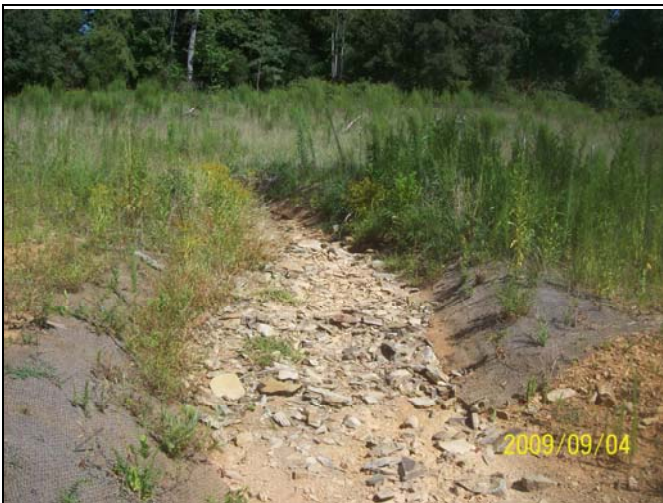
UT2 PID 5 – Constructed Riffle
