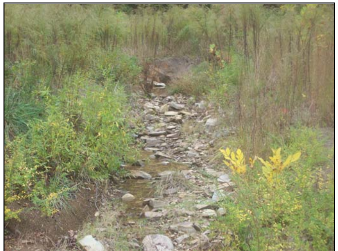
UT2 PID 6 – Constructed Riffle
