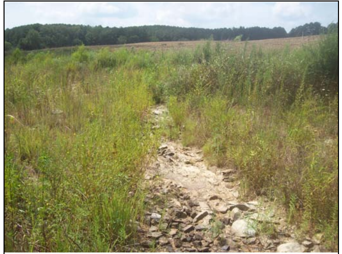
UT1 PID 32 – Constructed Riffle, UT1 Reach 2
