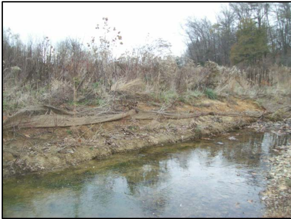
VPA 1 – Bare bank with damaged matting
