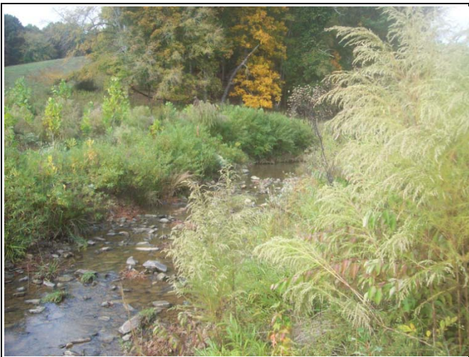
BCC PID 17 – Constructed Riffle, UT1 Reach 3
