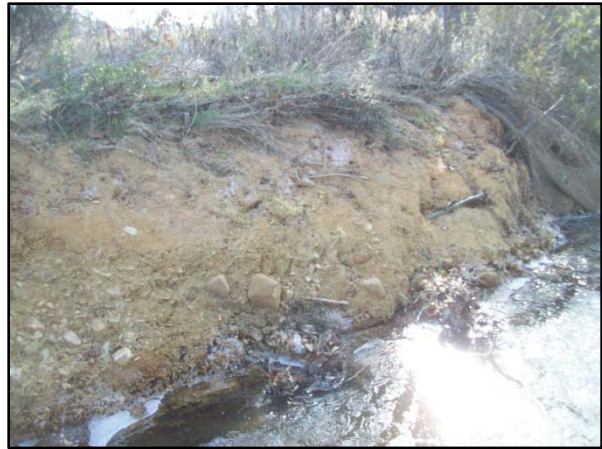
VPA 2 – Bare bank with loss of matting
