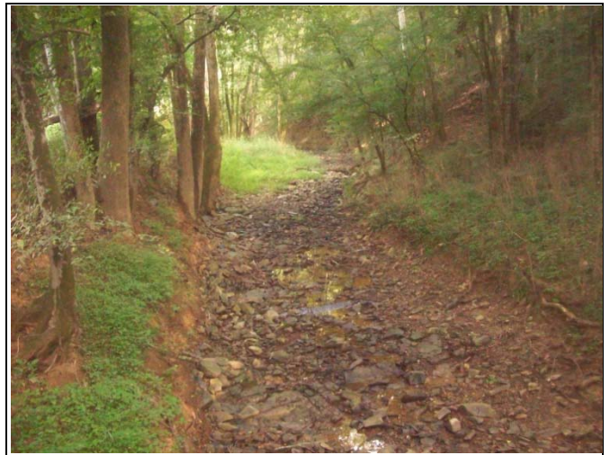
BCC PID 4 – Re-graded Riffle, BCC Reach 6
