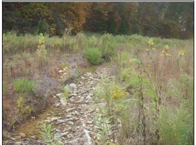
UT2 PID 4 – Constructed Riffle
