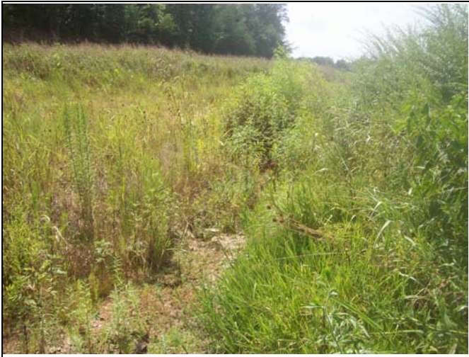
UT1 PID 31 – Constructed Riffle, UT1 Reach 2 End
