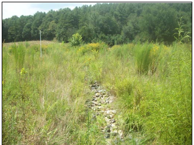
UT1 PID 48 – Constructed Riffle, UT1 Reach 1
