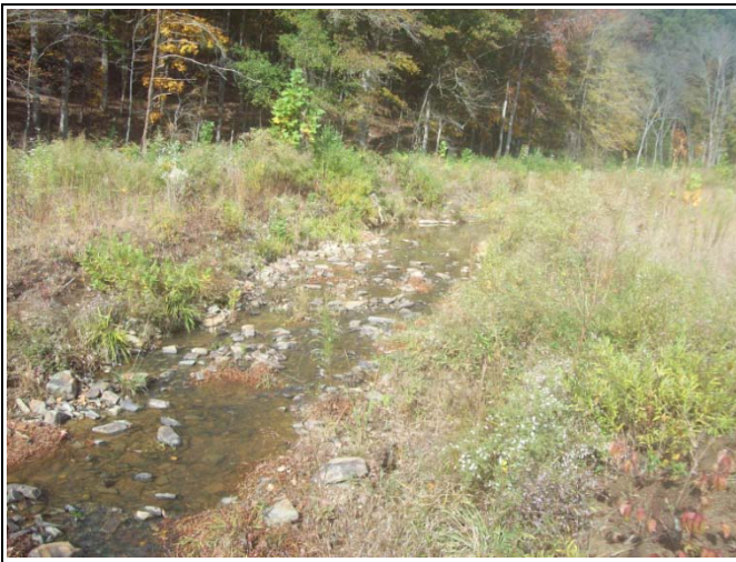
BCC PID 9 – Constructed Riffle, BCC Reach 4
