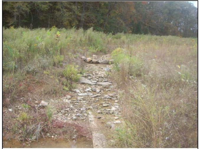
UT2 PID 2 – Constructed Riffle
