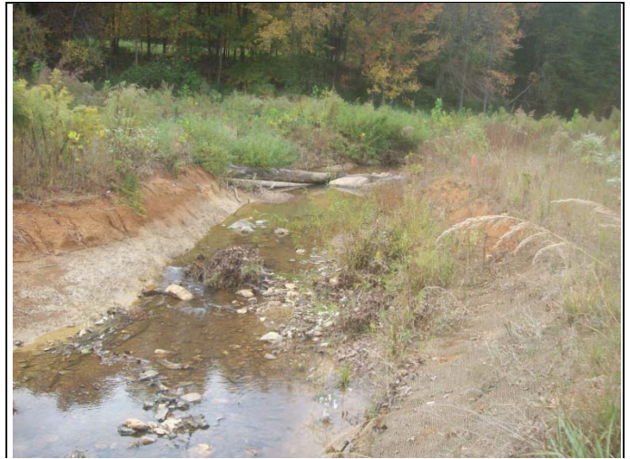
BCC PID 28 – Log J-Hook & Constructed Riffle, BCC Reach 2
