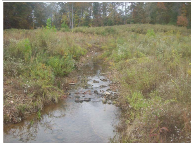
BCC PID 40 – Constructed Riffle, BCC Reach 1 End
