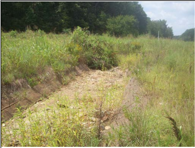
UT1 PID 7 – Constructed Riffle, UT1 Reach 4
