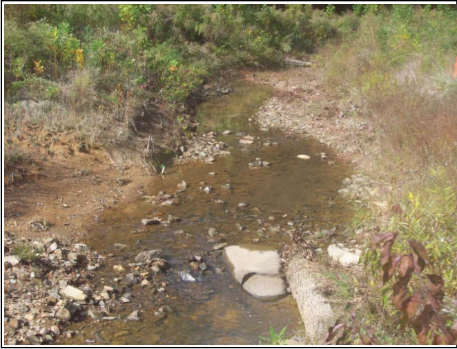
BCC PID 21 – Constructed Riffle, BCC Reach 3
