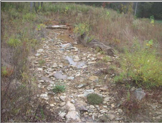
UT2 PID 3 – Constructed Riffle
