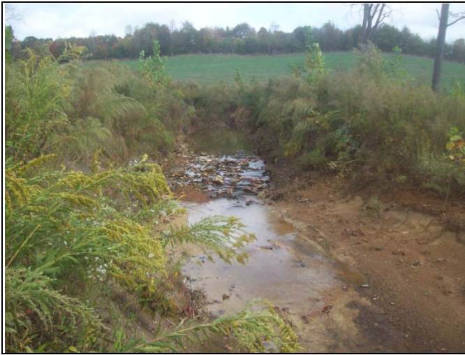
BCC PID 33 – Constructed Riffle, BCC Reach 2
