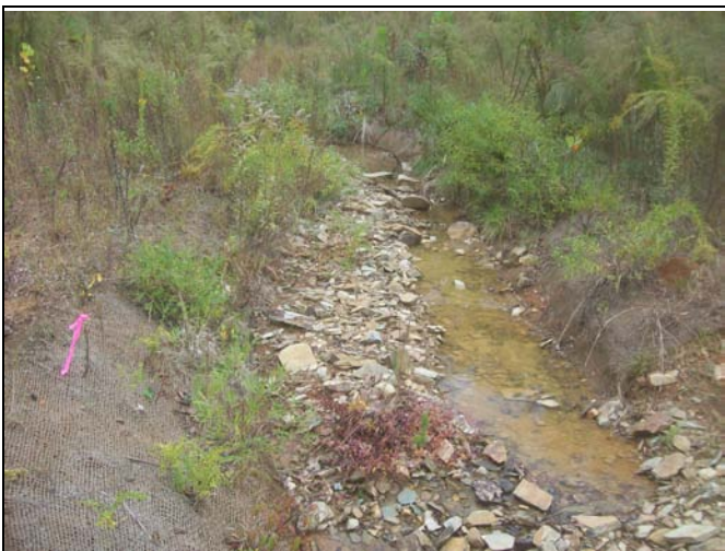
UT2 PID 5 – Constructed Riffle
