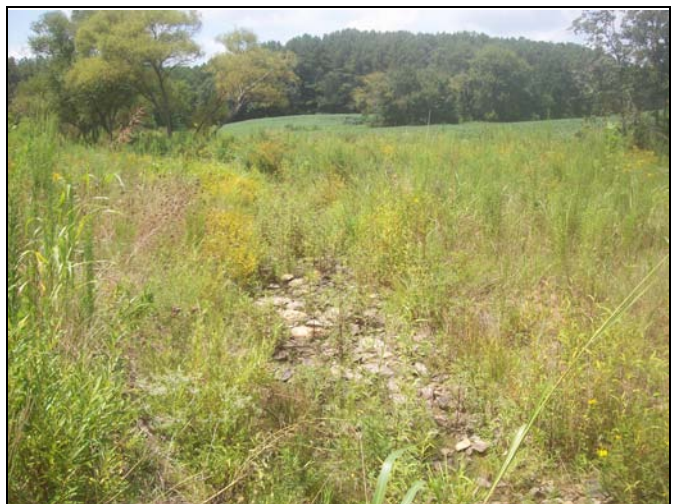
UT1 PID 12 – Constructed Riffle, UT1 Reach 3 End
