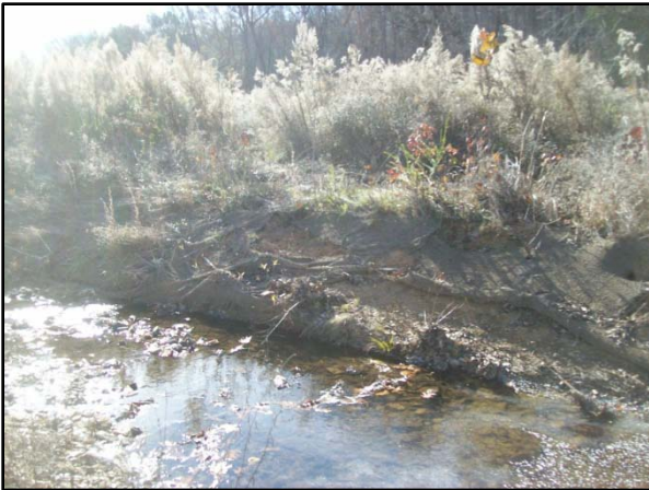
VPA 11 – UT2 Bare Bank with loss of matting
