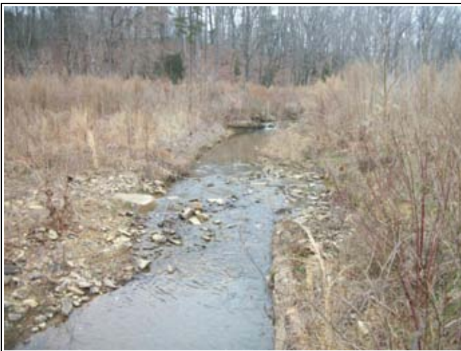
BCC PID 11 – Log J-Hook & Constructed Riffle, BCC Reach 3 End
