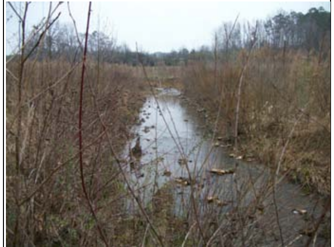
BCC PID 14 – Constructed Riffle, BCC Reach 3
