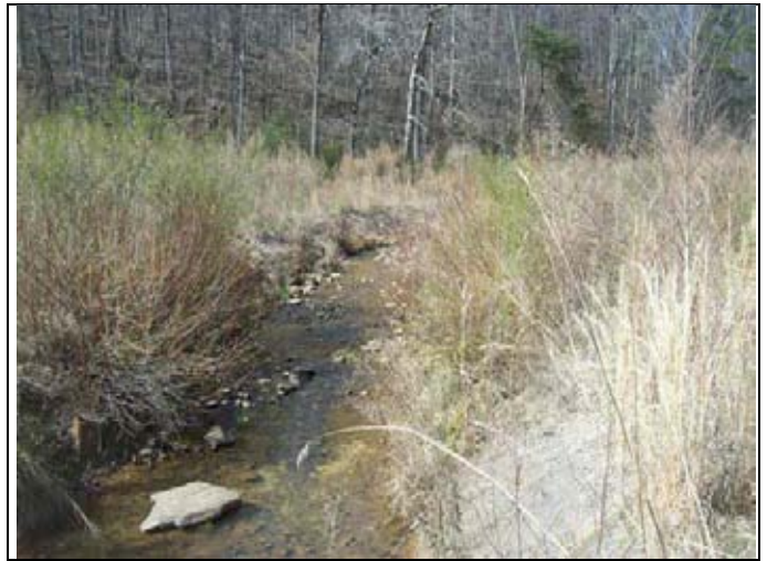
BCC PID 34 – Constructed Riffle, BCC Reach 2
