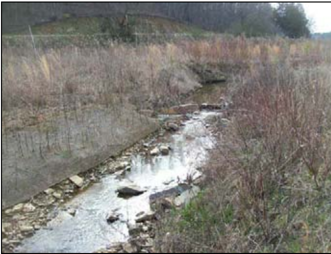
UT1 PID 9 – Constructed Riffle, UT1 Reach 4
