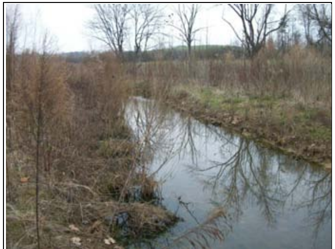
BCC PID 18 – Constructed Riffle, BCC Reach 3
