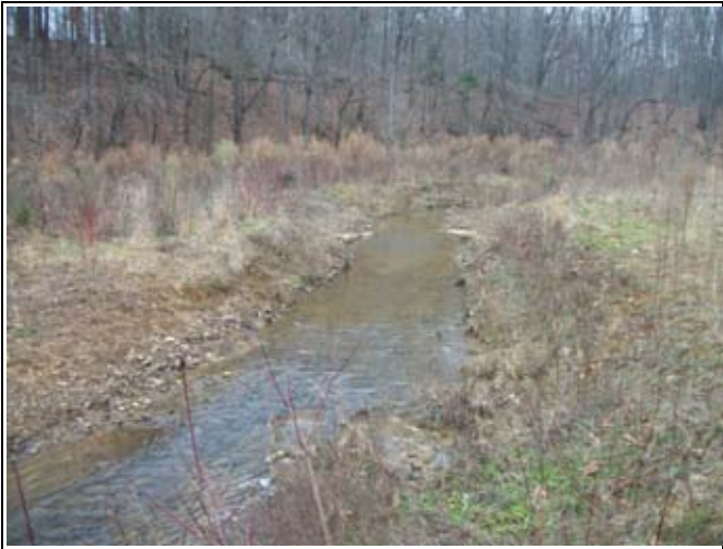
BCC PID 21 – Constructed Riffle, BCC Reach 3
