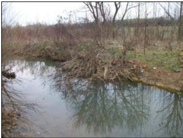
SPA 3 – Bank scour near abandoned beaver lodge
