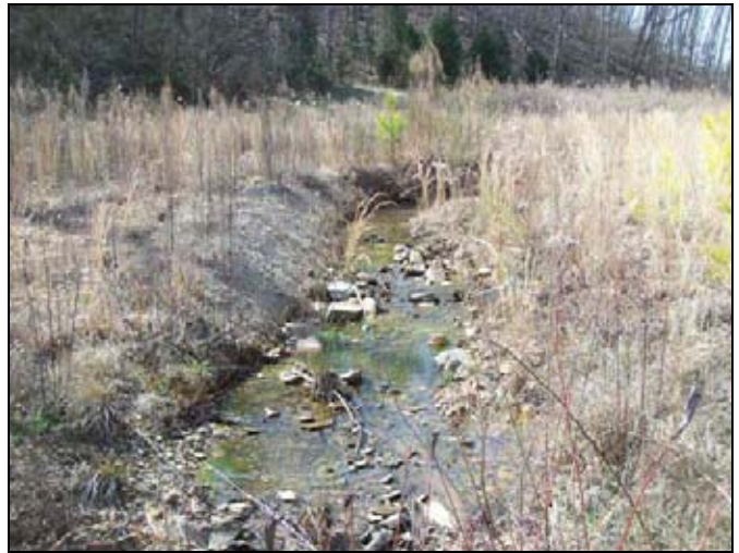
UT2 PID 4 – Constructed Riffle
