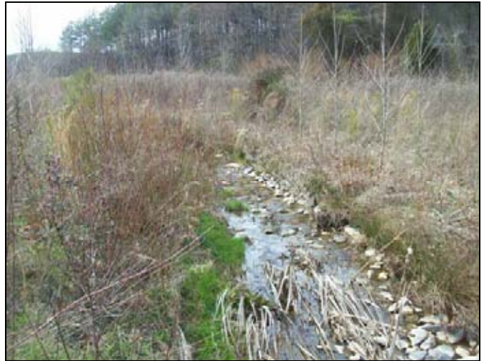
UT1 PID 22 – Constructed Riffle, UT1 Reach 3
