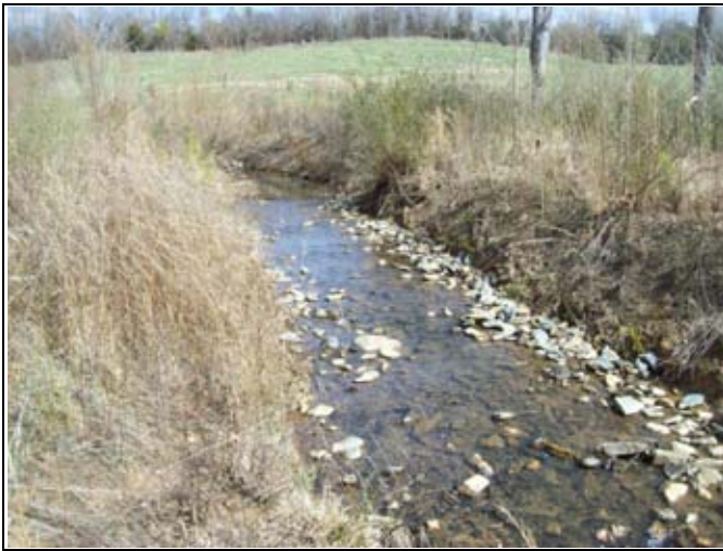
BCC PID 33 – Constructed Riffle, BCC Reach 2
