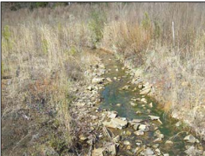
UT2 PID 5 – Constructed Riffle
