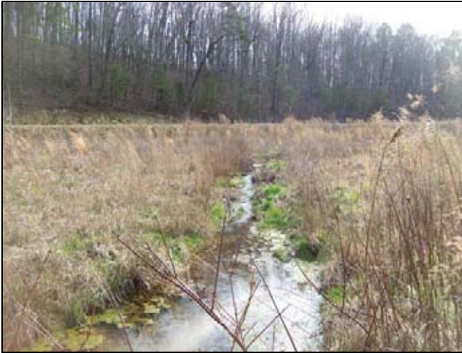
UT1 PID 19 – Constructed Riffle, UT1 Reach 3
