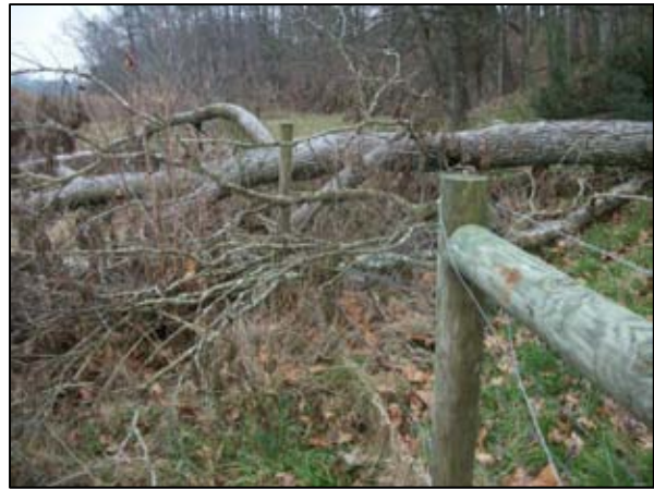
SPA 2 – Conservation easement damage caused by fallen tree
