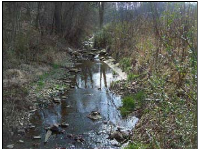
UT1 PID 4 – Constructed Riffle, UT1 Reach 4
