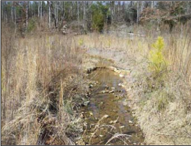
UT2 PID 7 – Constructed Riffle
