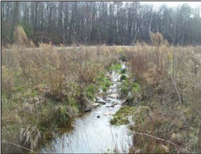
UT1 PID 21 – Constructed Riffle, UT1 Reach 3
