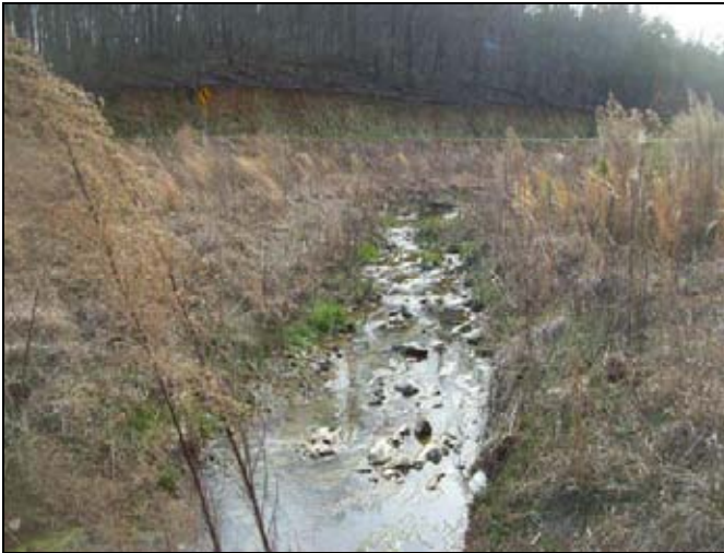
UT1 PID 27 – Constructed Riffle, UT1 Reach 3
