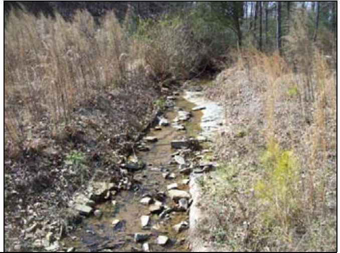
UT2 PID 8 – Constructed Riffle, UT2 Start
