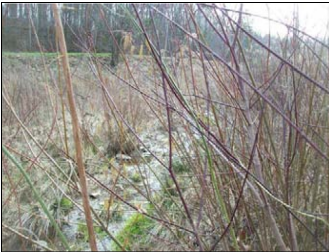
UT1 PID 15 – Constructed Riffle, UT1 Reach 3
