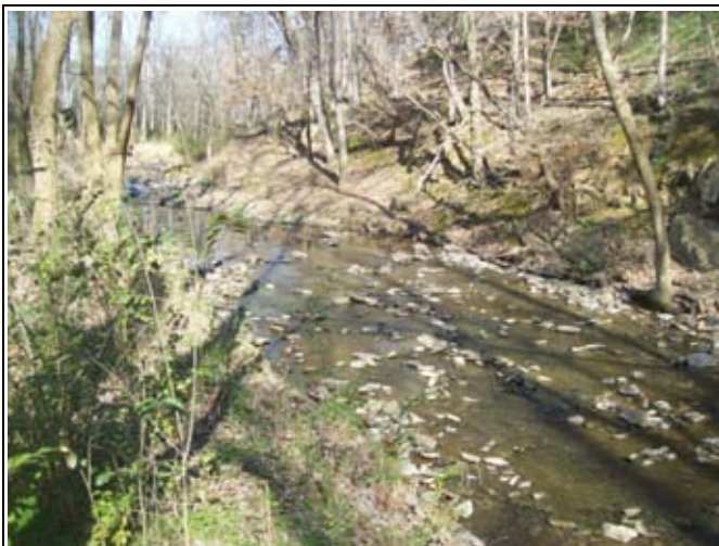
BCC PID 5 – Re-graded Riffle, BCC Reach 6
