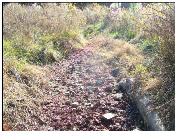
SPA 6 – Shifted thalweg along UT1 Station 44+25-44+75
