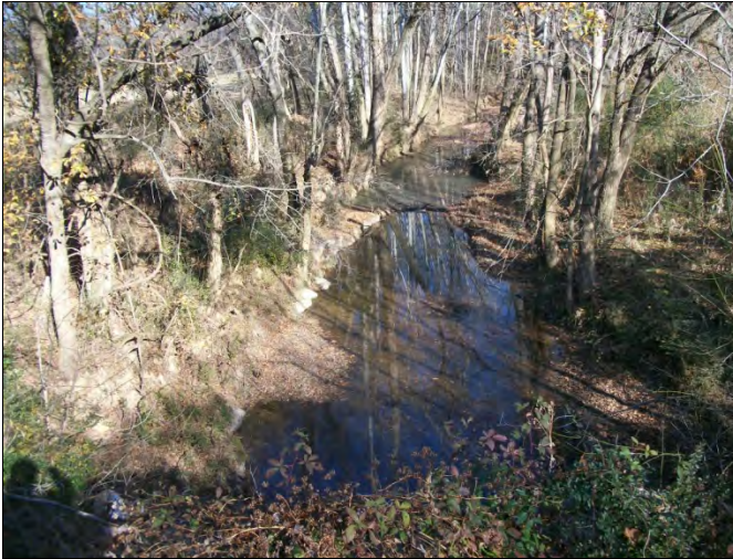
BCC PID 1– Cross Vane, BCC Reach 6 End
