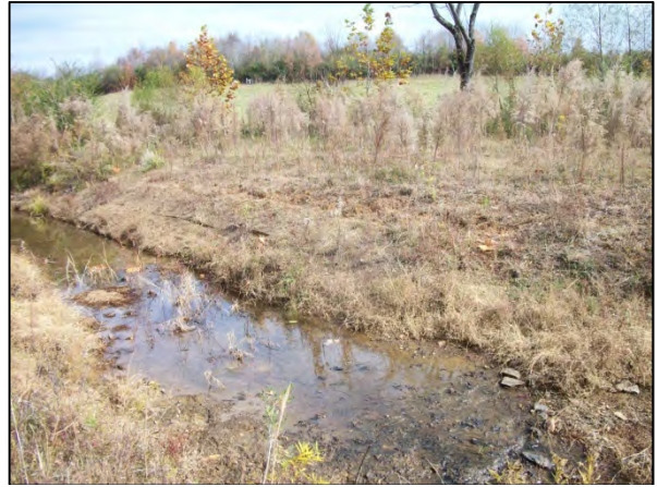
SPA 2 – Minor bank erosion along BCC at Station 30+50 to 32+75, left bank
