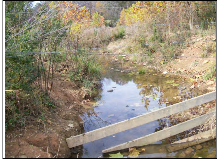
BCC PID 26 – Constructed Riffle, BCC Reach 2
