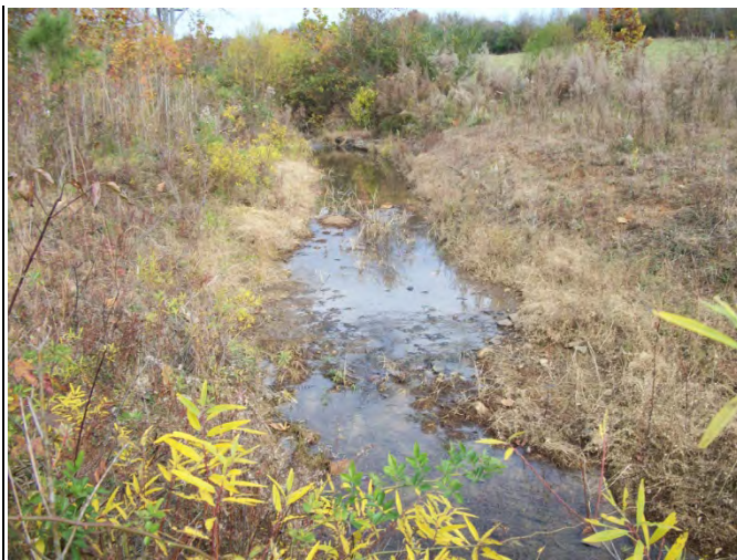
BCC PID 29 – Log J-Hook & Constructed Riffle, BCC Reach 2
