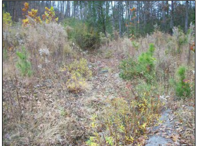
UT2 PID 8 – Constructed Riffle, UT2 Start
