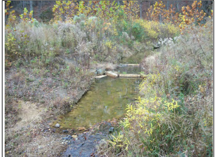
BCC PID 32 – Constructed Riffle, BCC Reach 2
