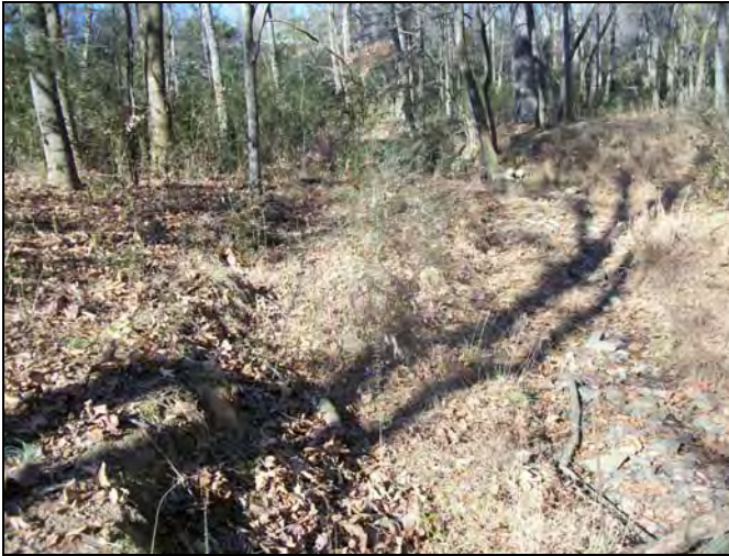
UT1 PID 1 – Constructed Riffle, UT1 Reach 4 End
