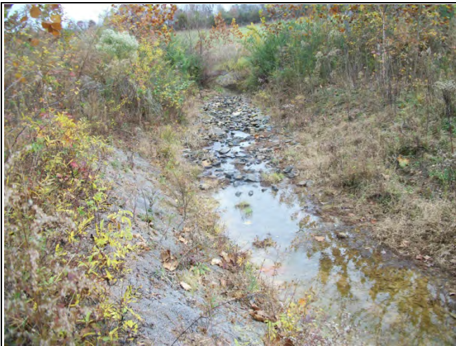
BCC PID 33 – Constructed Riffle, BCC Reach 2
