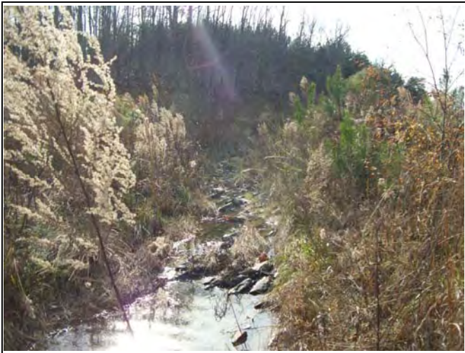
UT1 PID 27 – Constructed Riffle, UT1 Reach 3
