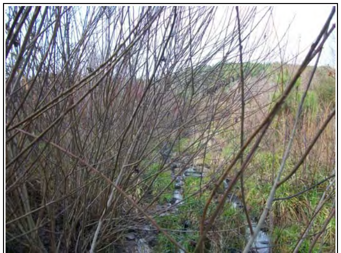
UT1 PID 12 – Constructed Riffle, UT1 Reach 3 End
