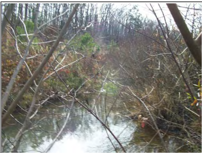
UT1 PID 17 – Constructed Riffle, UT1 Reach 3
