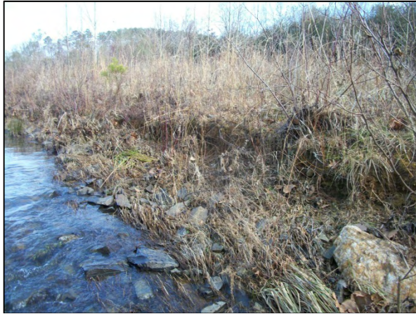
SPA 3 – Minor bank erosion on left bank of BCC from Station 60+00 to 59+60
