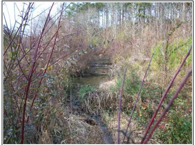
UT1 PID 28 – Log sill step pools (3), UT1 Reach 3
