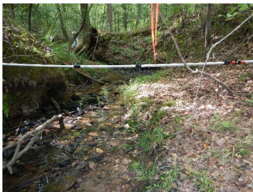
Narrow bankfull bench along right bank of riffle section (looking downstream)
