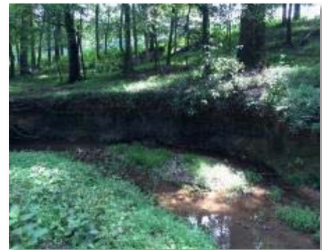
Upper Stick Elliott Creek Reach 4a, eroding banks
