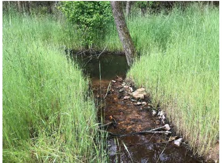
Bridges Crk UT1 Photo Point 82 – view downstream (04/25/2018)
