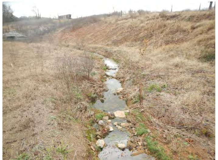
Royster Creek Photo Point 41 – view downstream (11/29/2018)
