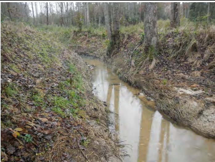
USEC R3 Photo Point 62 – view upstream (11/14/2018)
