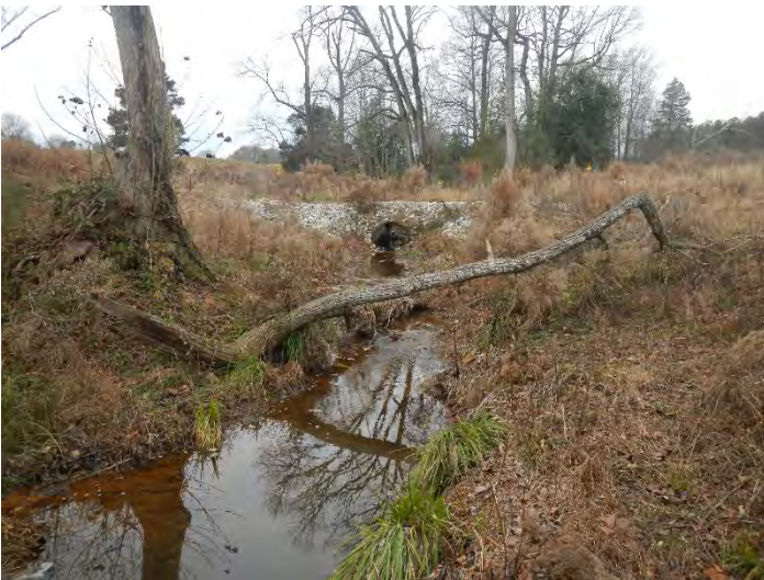
UFC R2 Photo Point 88 – view upstream (12/07/2018)
