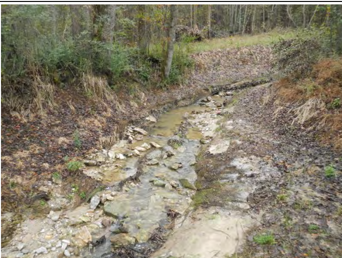
USEC R2 Photo Point 59 – view upstream (11/14/2018)
