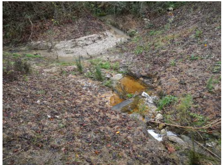
USEC UT1 Photo Point 74 – view downstream (11/14/2018)
