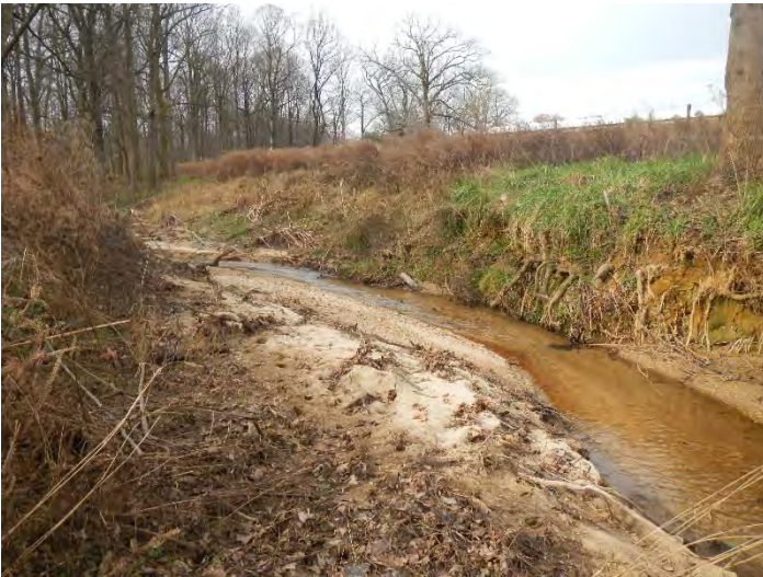
LFC R1 Photo Point 94 – view upstream (12/07/2018)
