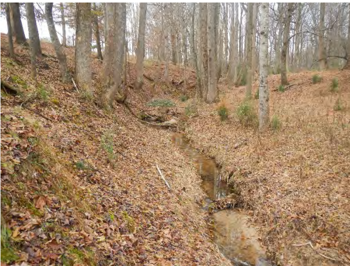
UFC R1 Photo Point 85 – view upstream (12/07/2018)
