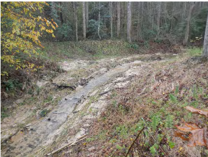
USEC R3 Photo Point 61 – view upstream (11/14/2018)
