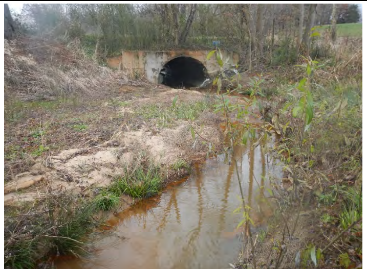
UBHC R2B Photo Point 9 – view downstream (11/30/2018)
