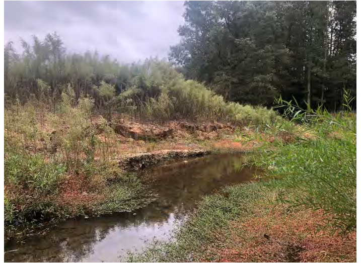
UBHC R6 Bank Scour (Station 176+00) – view downstream (10/8/2019)
