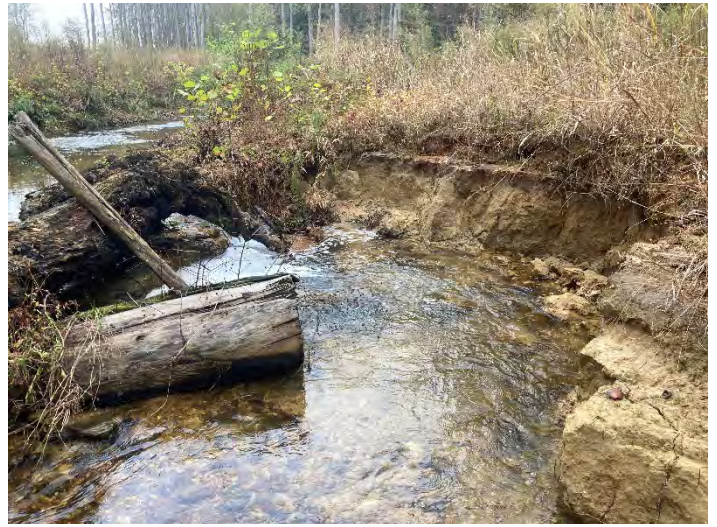
LBHC R2 Log Sill Bypassed (STA 317+45) – view upstream (10/27/2020)
