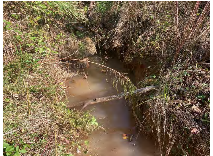
Scott Creek Incision (STA 1211+25 – 1211+36) – view upstream (11/2/2020)
