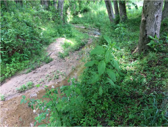
LFC R1 Photo Point 93 – view upstream (5/5/2020)
