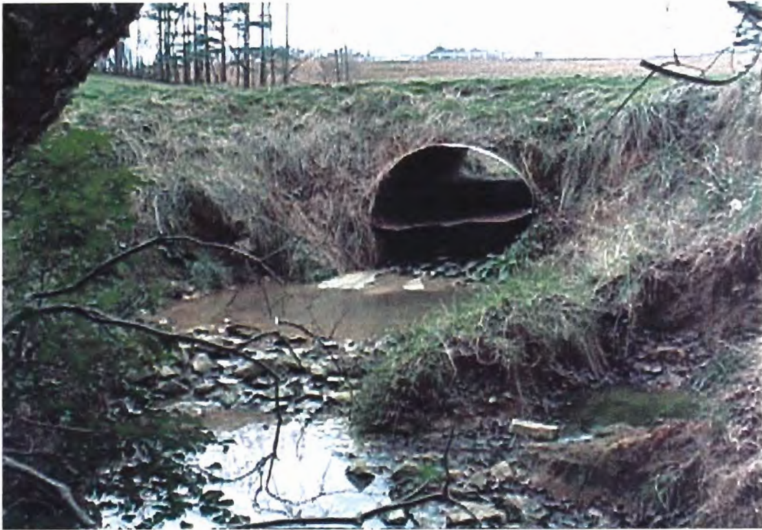
Lwbypassed culvert, AH&W 98-12-11
