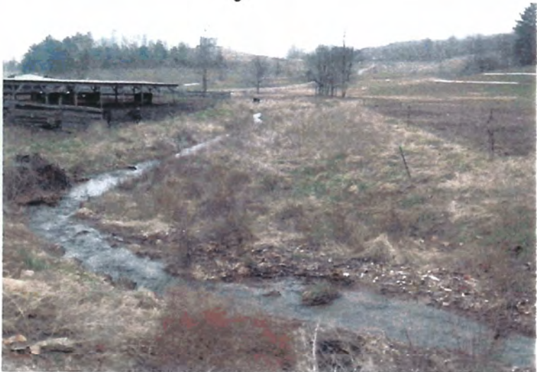
Big Warrior Creek after construction, 1/30/03
