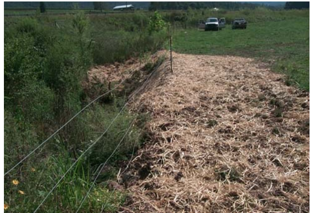
After stream bank repairs to the left bank around cross-section 3, September 2005.
