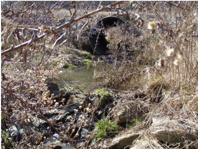
Photograph looking upstream at the culvert, December 2007.
