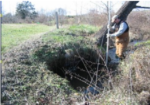
Area below cross-section 4. Note: large walnut tree leaning.
