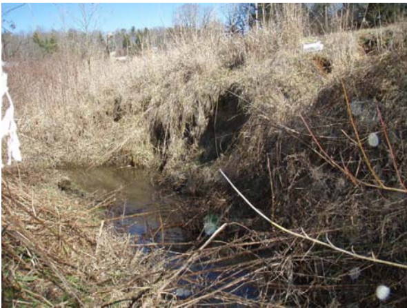
Area between cross-sections 1 and 2, LDS.
