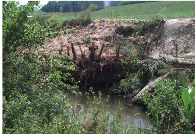
After stream bank repairs to the left bank above cross-section 3, September 2005.
