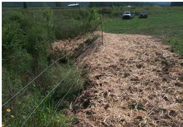
After stream bank repairs to the left bank around cross-section 3, September 2005.
