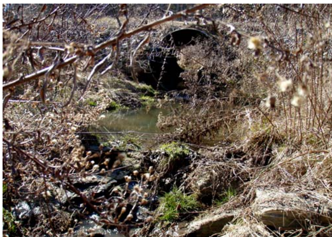
Photograph looking upstream at the culvert, December 2007.
