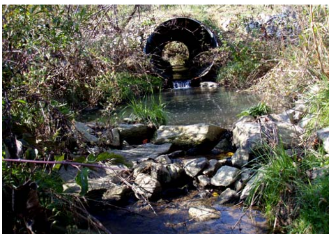
Photograph looking upstream at the culvert, November 2008.
