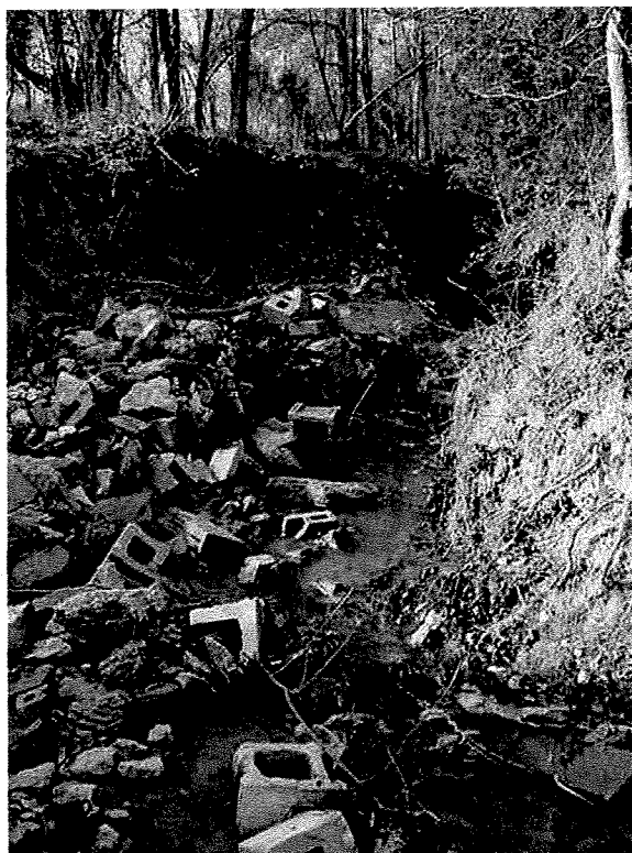
Picture 25. Highly incised and eroded stream banks. Debris added to stabilize channel.
