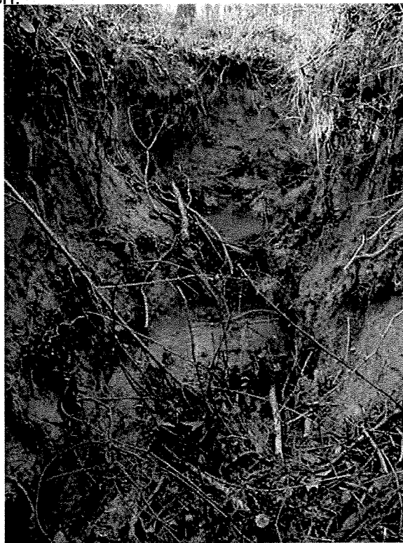
Picture 22. Highly incised and eroded stream banks downstream from Picture 21.
