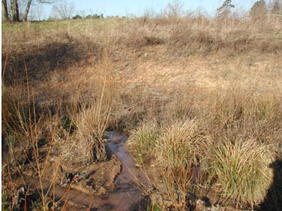
Photo 1. Representative bare floodplain problem area (Station 10+50 along plan view).
