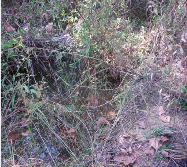
Photo 1. Representative bare bank problem area (Station No. 21+02; view from left bank; 9-14-2008).
