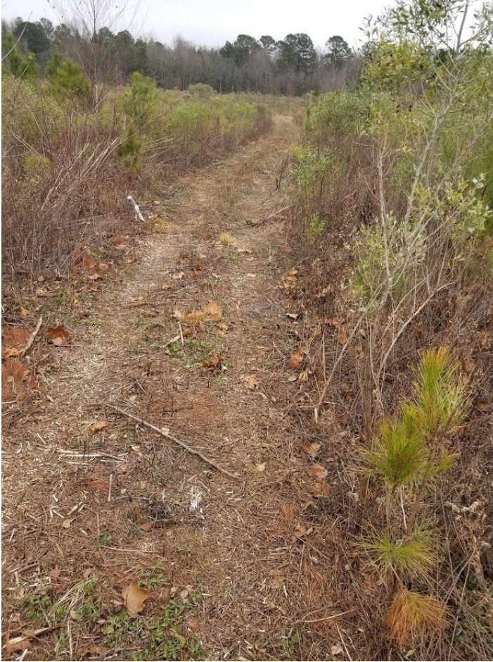
Mowed path inside credit area and destroyed wetland gauge 1. 12/9/20 Total area of mowed path ~1,200' x 4' wide = 0.1 acre
