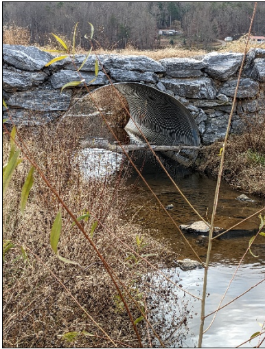
PP-13: R1, Downstream, Station 24+25- Culvert
