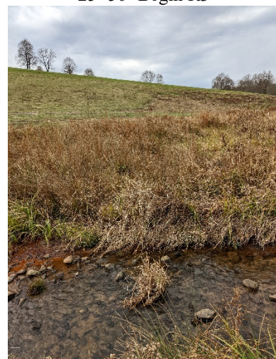
PP-42: R1, Swale on Right Floodplain, Station 16+25
