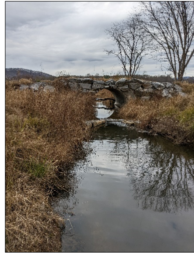
PP-14: R1, Upstream, Station 25+60- Culvert
