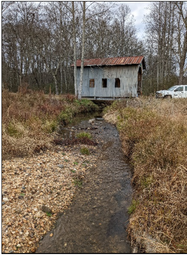
PP-1: R1 Upstream, Station 10+75- Begin R1
