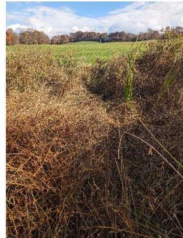
Encroachment Area into existing drain swale. R1 Left floodplain.
