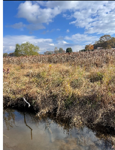
PP-44: R1, Swale on Left Floodplain, Station 20+70
