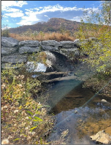
PP-13: R1, Downstream, Station 24+25- Culvert
