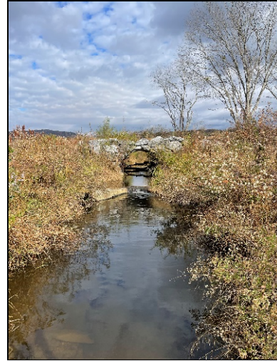
PP-14: R1, Upstream, Station 25+60- Culvert
