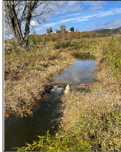
PP-22: R1, Upstream, Station 36+75
