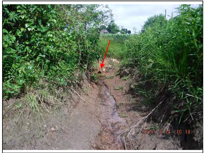
Lower R2, field drain pipe outfall into left bank (6/14/18)
