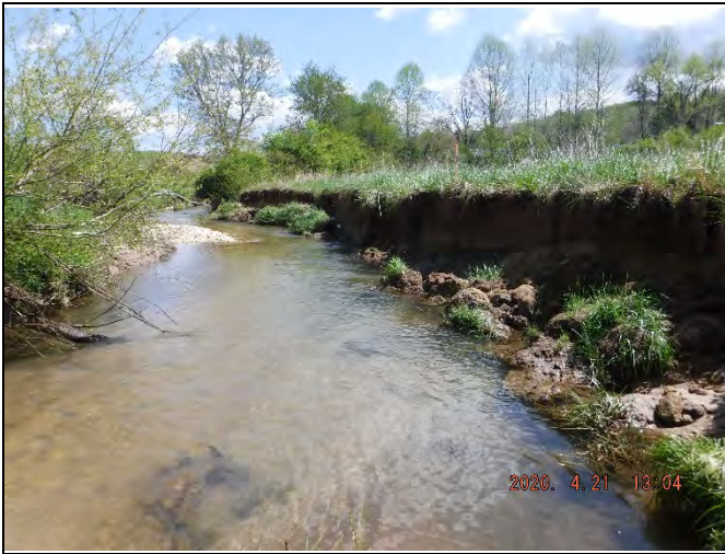
Reach R3, downstream (4/21/20)
