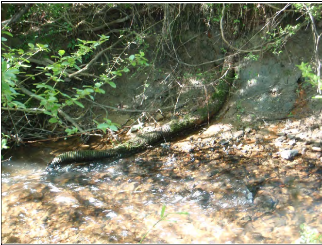
Old Field Drain Pipe along Reach R1
