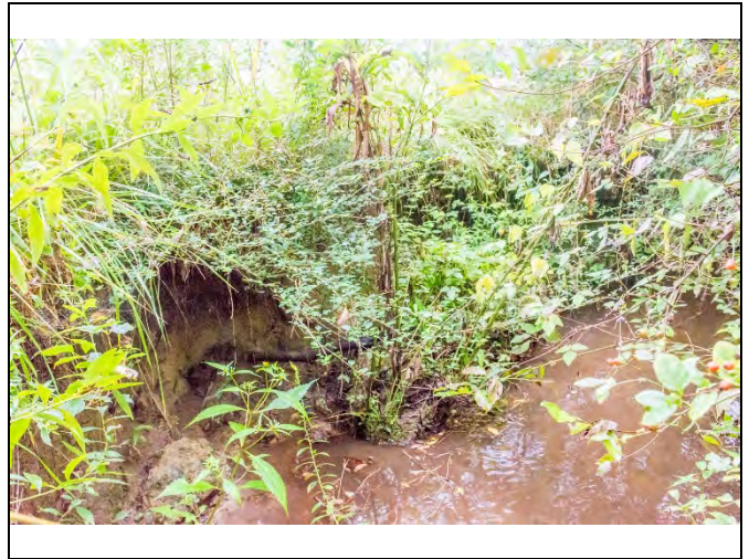
Lower Reach R2, left bank (Aug 2017)
