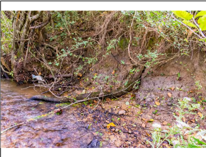
Upper Reach R1, drain pipe outfall (Aug 2017)
