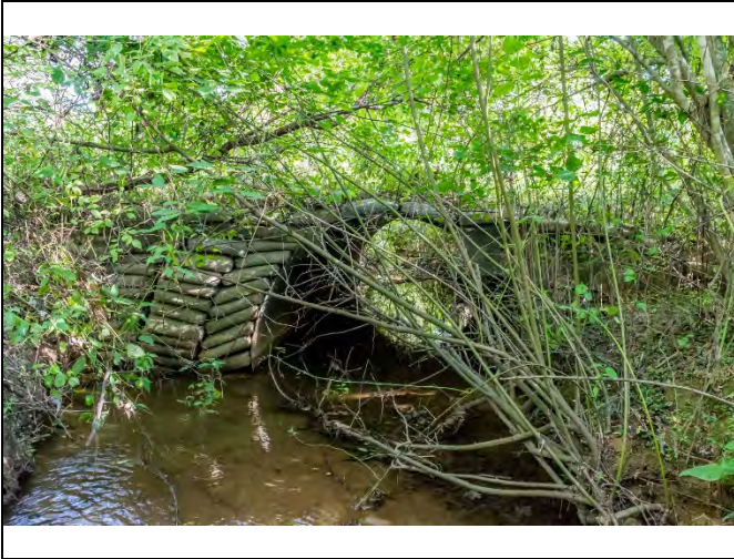
Mid Reach R1, culvert crossing (Aug 2017)
