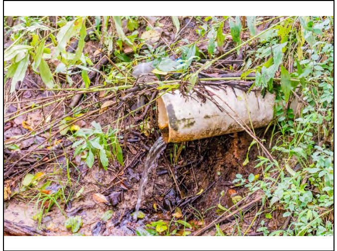
Upper Reach R1, drain pipe outfall (Aug 2017)
