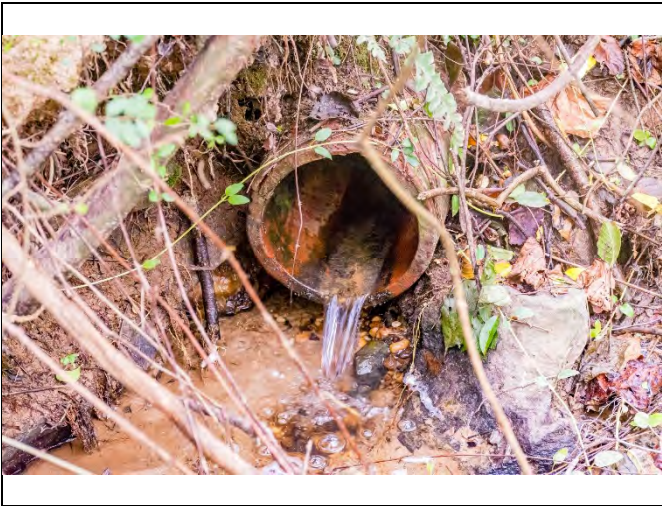
Upper Reach R1, drain pipe outfall (Aug 2017)
