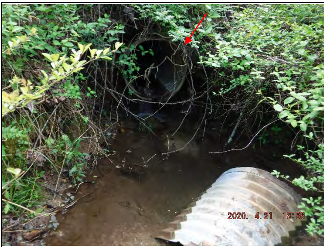
Reach UT1, culvert origin under Cherry Rd (4/21/20)
