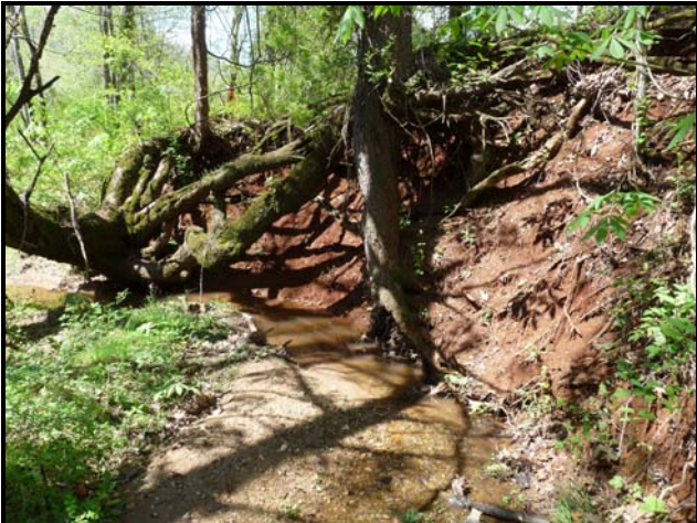
Undercutting of vegetation and side slope degradation
