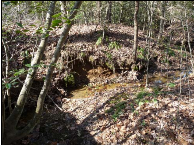
Undercutting of bank in meander
