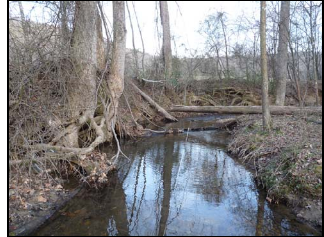
Undercut trees stabilizing bank at terrace
