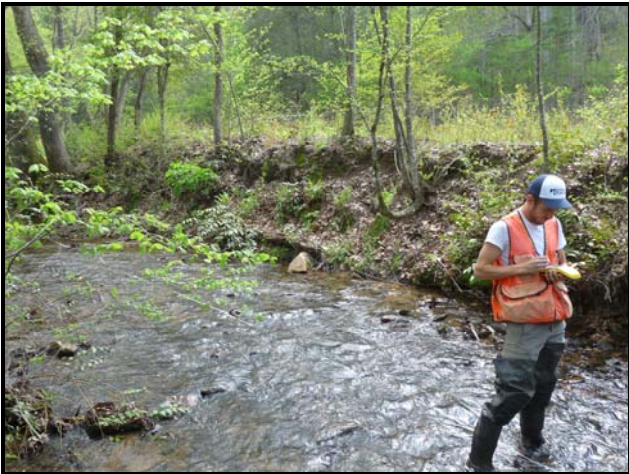
Degrading left bank along terrace side slope
