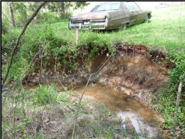
Vertical bank in meander
