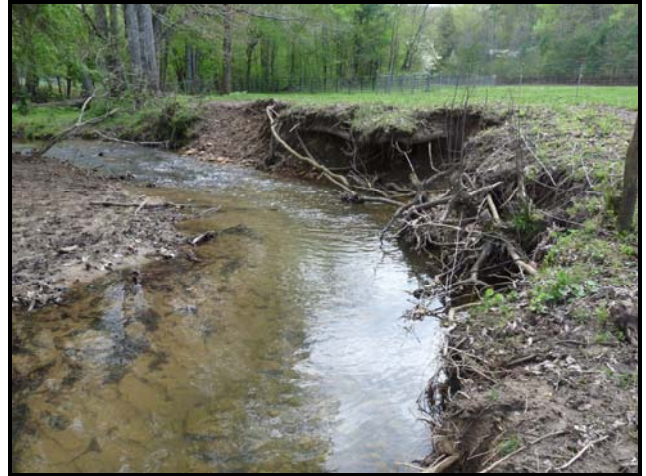
Degraded meander and fine sediments in channel
