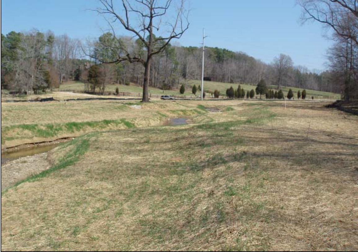
Photo Point 4c: View looking east, with vegetation plot #3 on the right. 3/9/07 – As-Built
