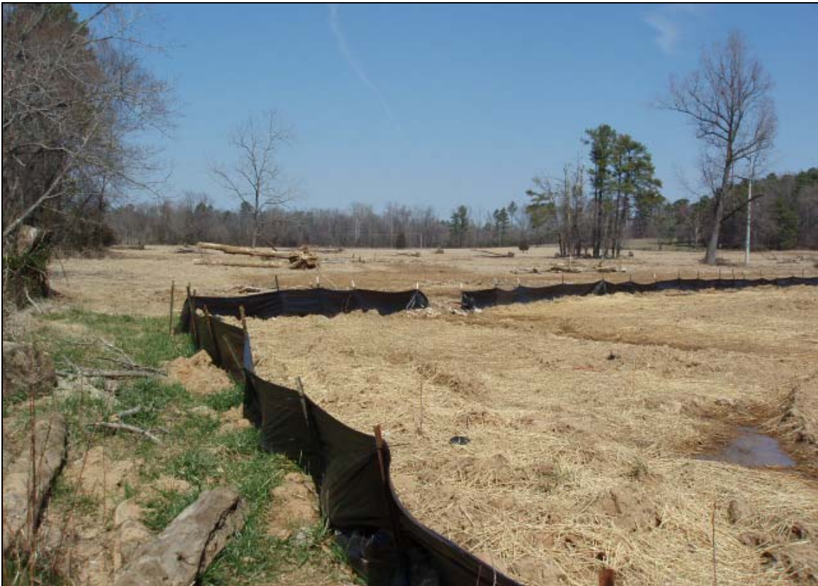
Photo Point 5a: View looking northeast, toward buffer area. 3/9/07 – As-Built
