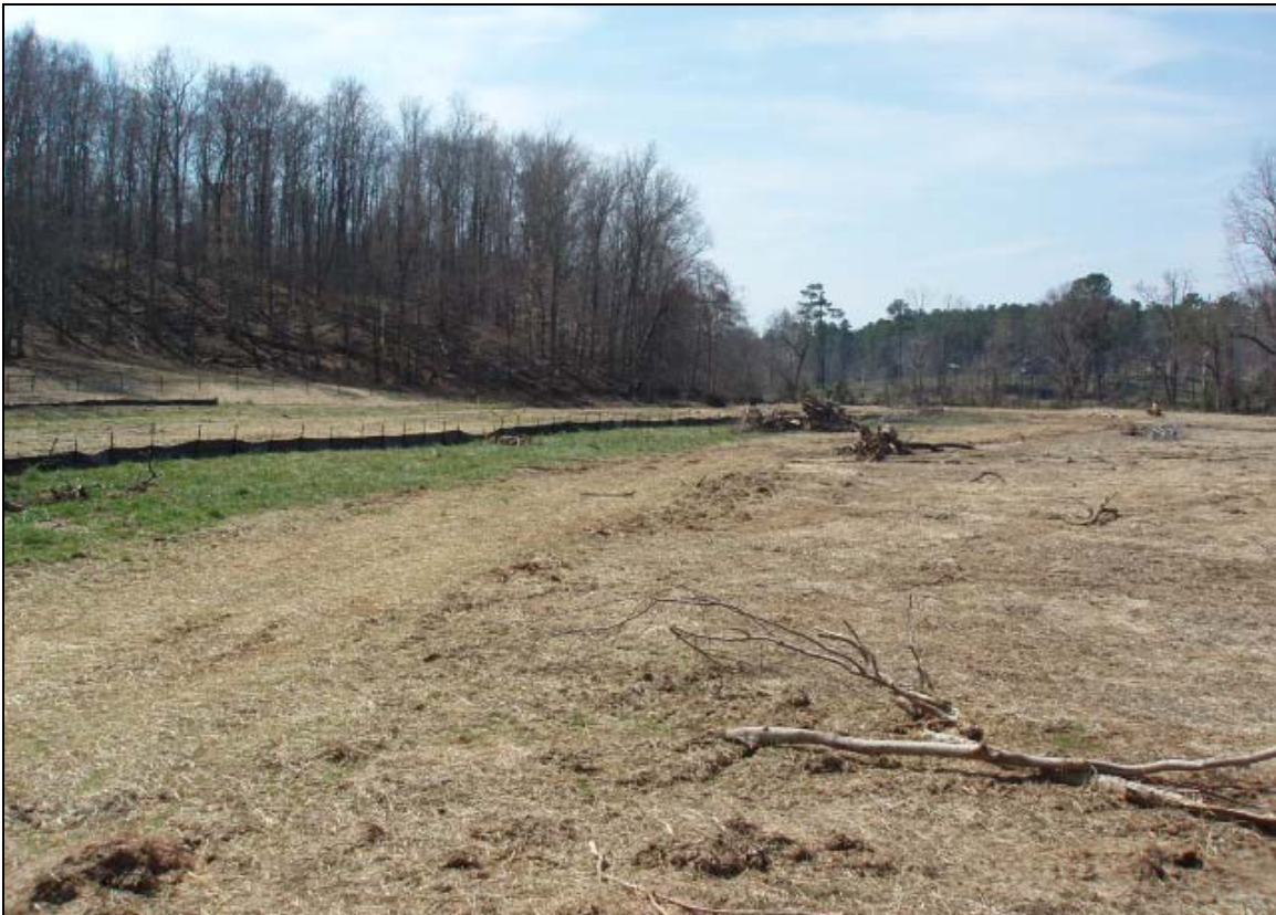
Photo Point 3b: View looking west, toward vegetation plot #5. 3/9/07 – As-Built
