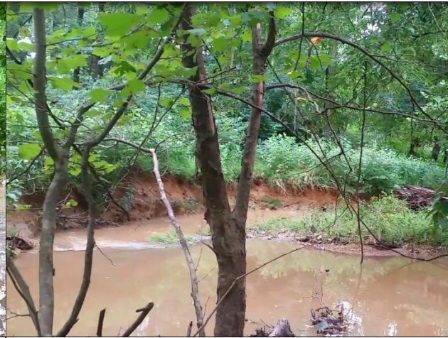
View looking east at eroded bank where the second soil lift will be installed. 7/14/15
