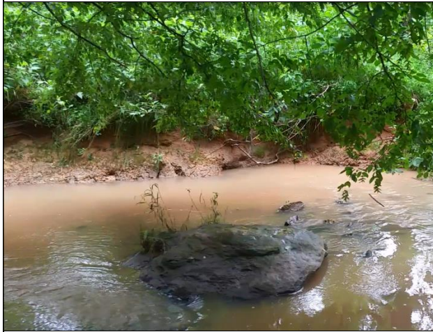
View looking west at eroded bank at the top of the project reach where the first (most upstream) soil lift will be installed. 7/14/15
