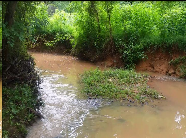
View looking west where the third soil lift will be installed. The bar will be graded. 7/14/15
